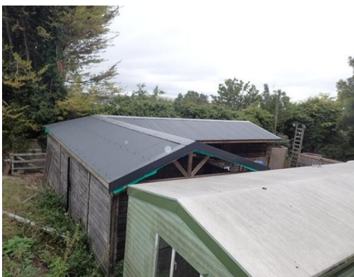
Figure 2.5. The stables viewed from the south
