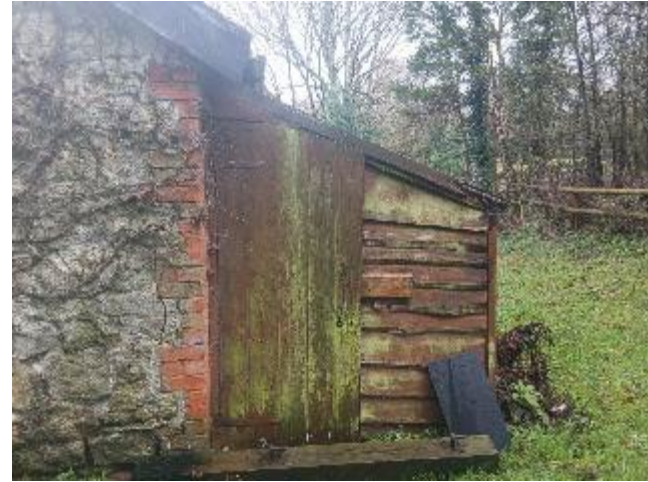
Photo 10: Southern elevation of B1
