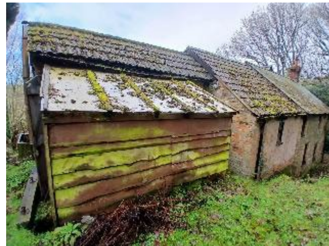
Photo 8: Eastern elevation of B1
