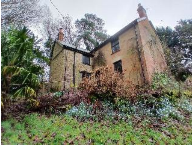
Photo 9: Northwestern elevation of B1
