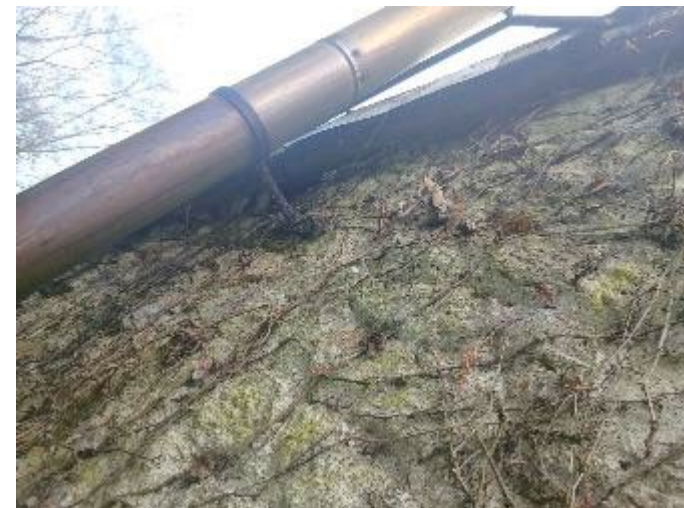
southern elevation of B1
