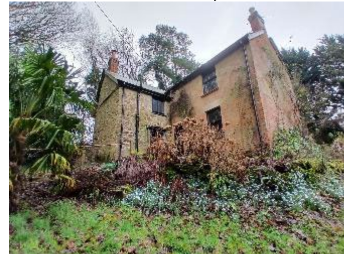
Northwestern elevation of B1
