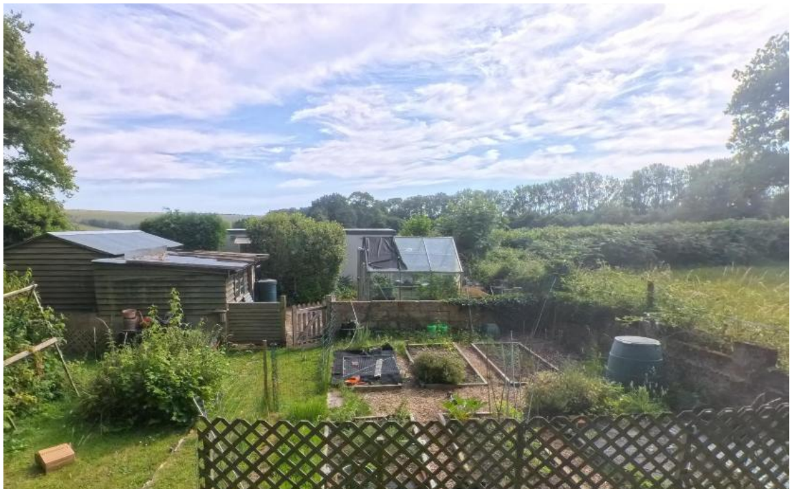
Figure. 4 - View looking south showing existing buildings.
