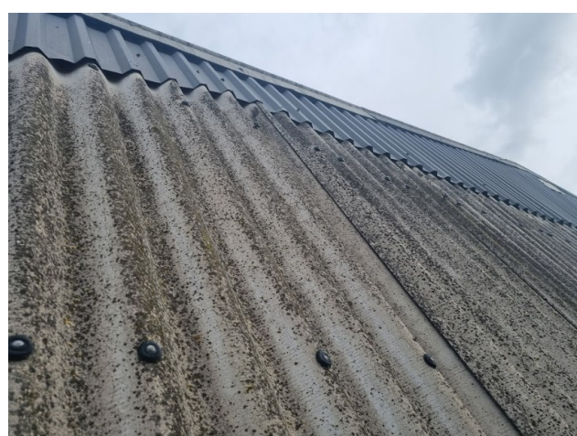
Photograph 4. Overlap of panel type on the front elevation.
