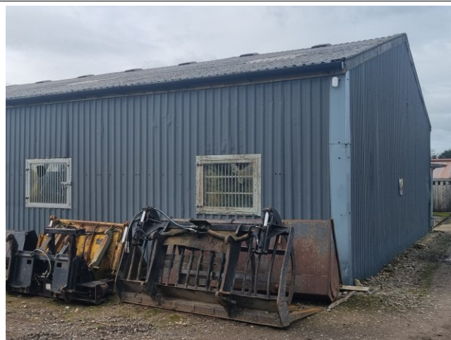
Photograph 6. Windows on the south-east elevation.
