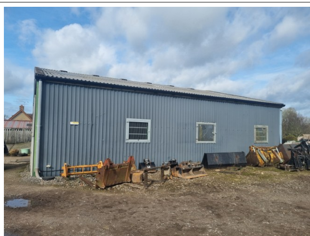
Photograph 2. Steel corrugated panels.
