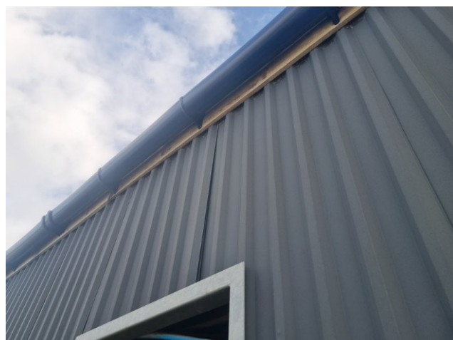
Photograph 5. Wooden fascia supporting the guttering.
