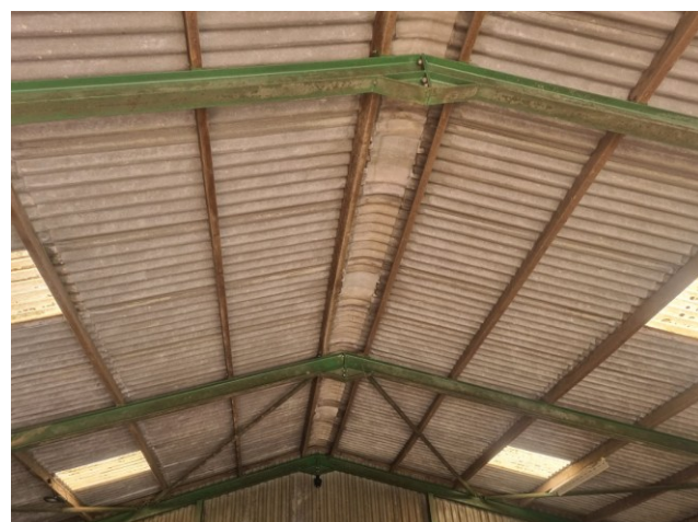
Photograph 9. The building had no internal roof void.
