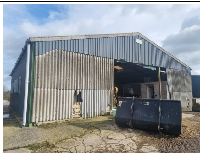
Photograph 3. The front south-western elevation.
