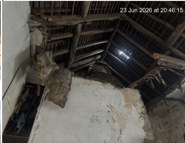
Photo 8: Internal roof view, partial collapse of roof and collapse of first floor in house.
