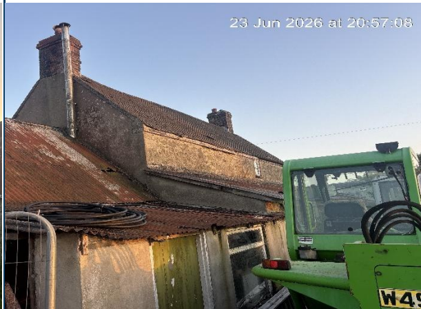
Photo 2: Rear elevation house.
