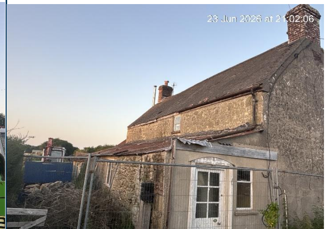
Photo 3: Rear elevation and extension of house.
