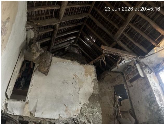
Photo 7: Internal roof view, partial collapse of roof and collapse of first floor in house.
