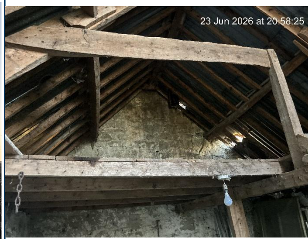
Photo 8: Internal roof view, partial collapse of roof and collapse of first floor in house.
