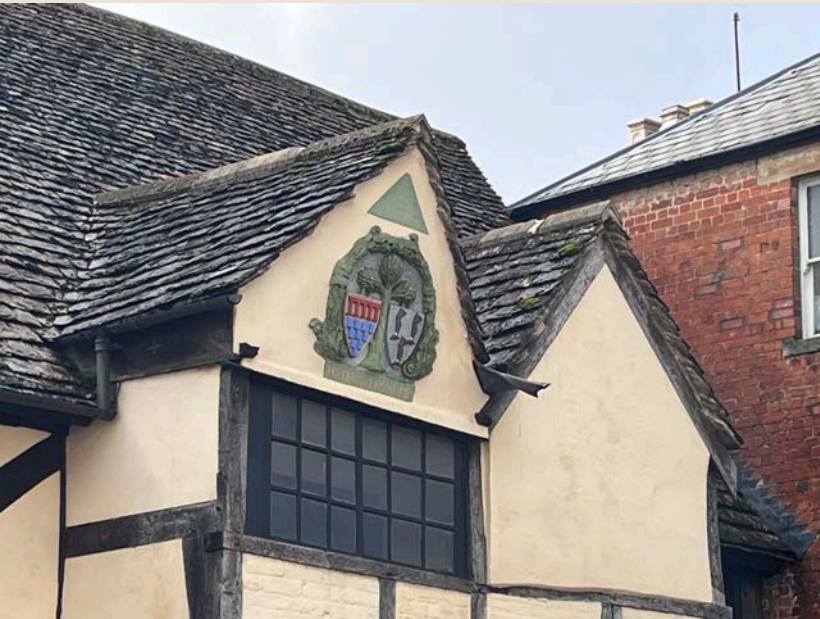
Figure 6: North elevation, lead-lined valley gutter (G4) discharging onto pavement below
