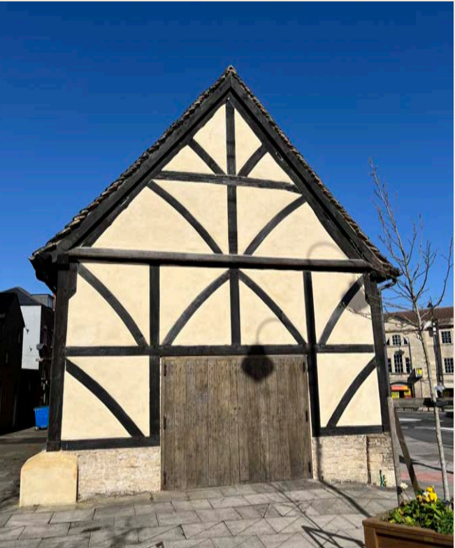
Figure 3: Yelde Hall, East elevation
