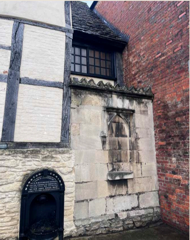
Figure 4: North elevation. Single storey section with metal roof, dog-toothed parapet stone wall, blank niche
