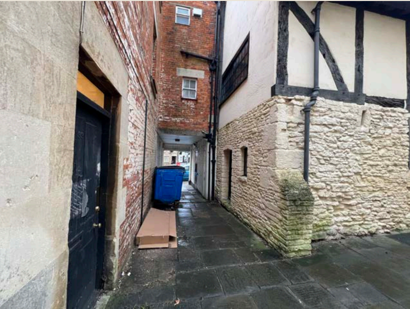
Figure 8: Yelde Hall, West elevation
