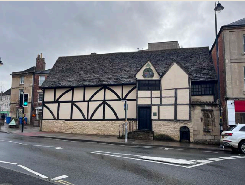
Figure 5: Yelde Hall, North elevation
