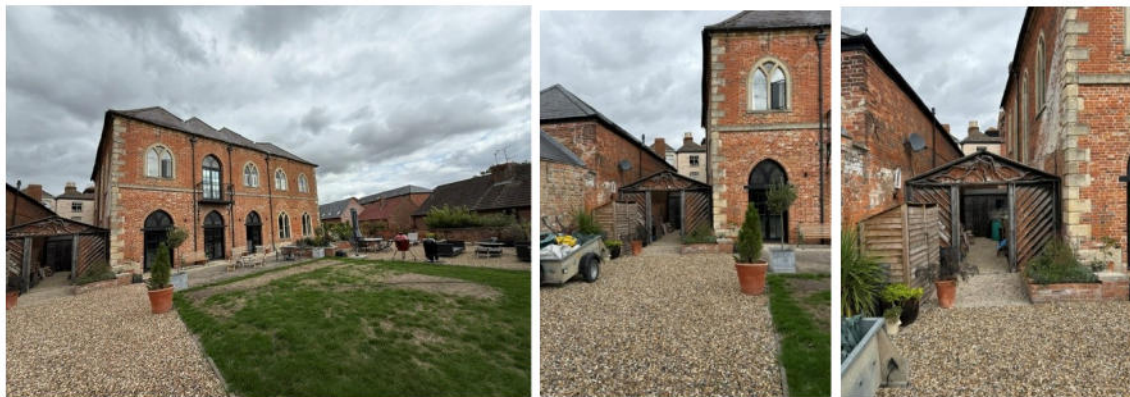
Southern elevation including timber side façade to the west, including various storage sheds in front and to the side of the house.
