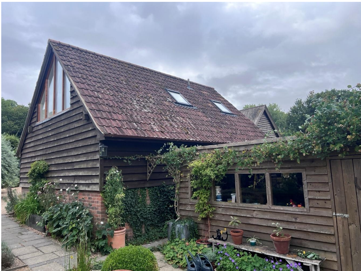
4. View of Garage from North West
