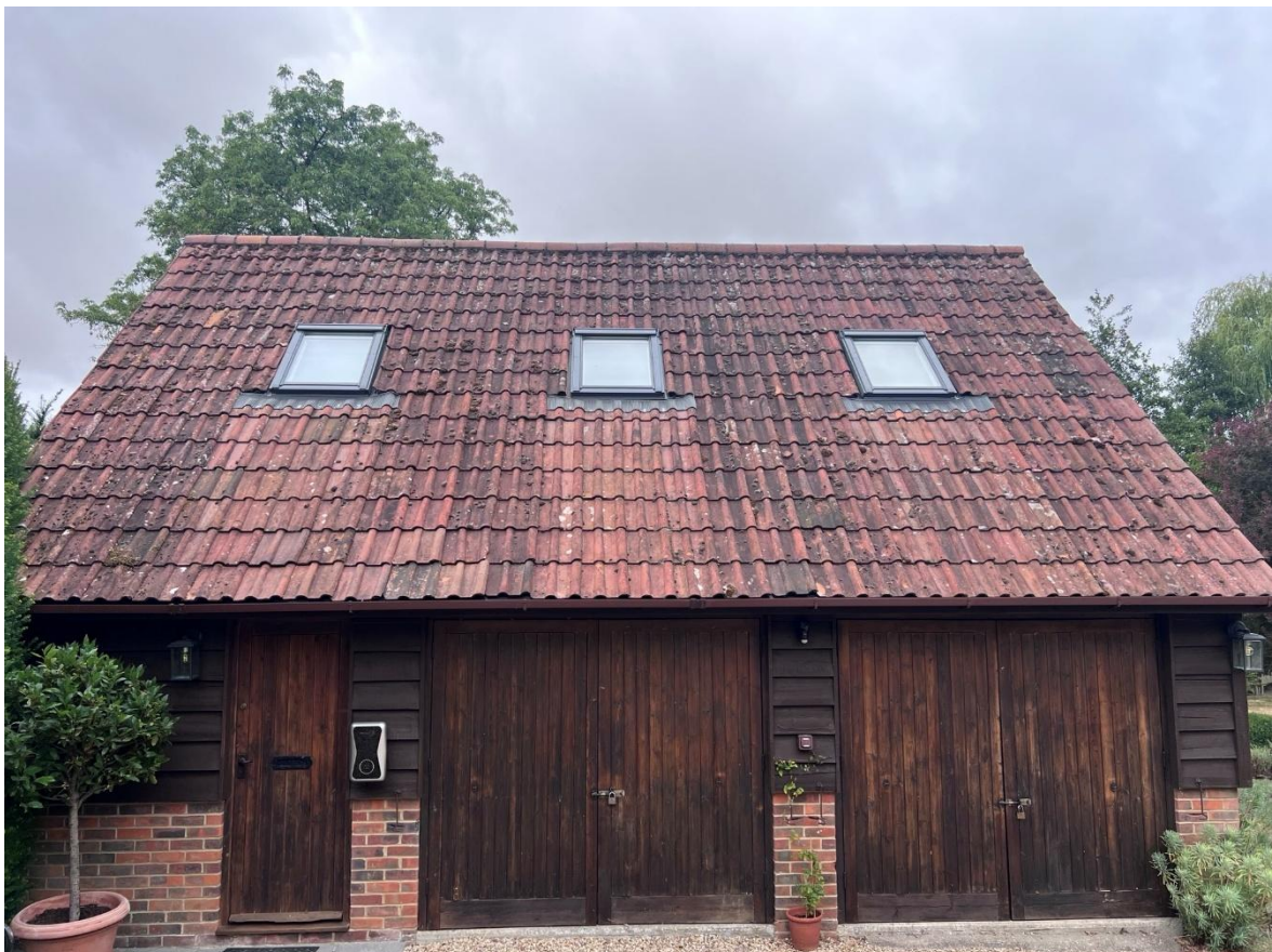
2. View of Garage from East
