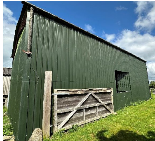
Image 5: Eastern Barn – east elevation
