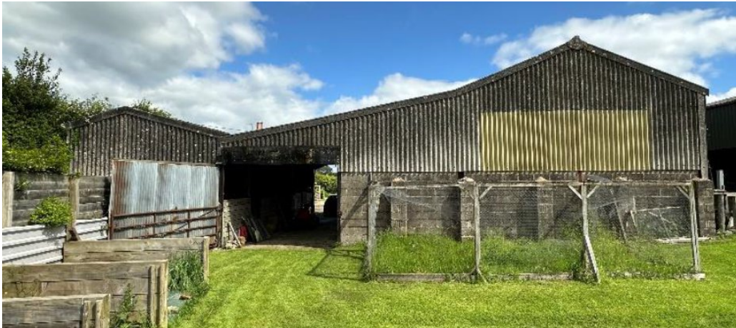
Image 3: Western Barn – south elevation
