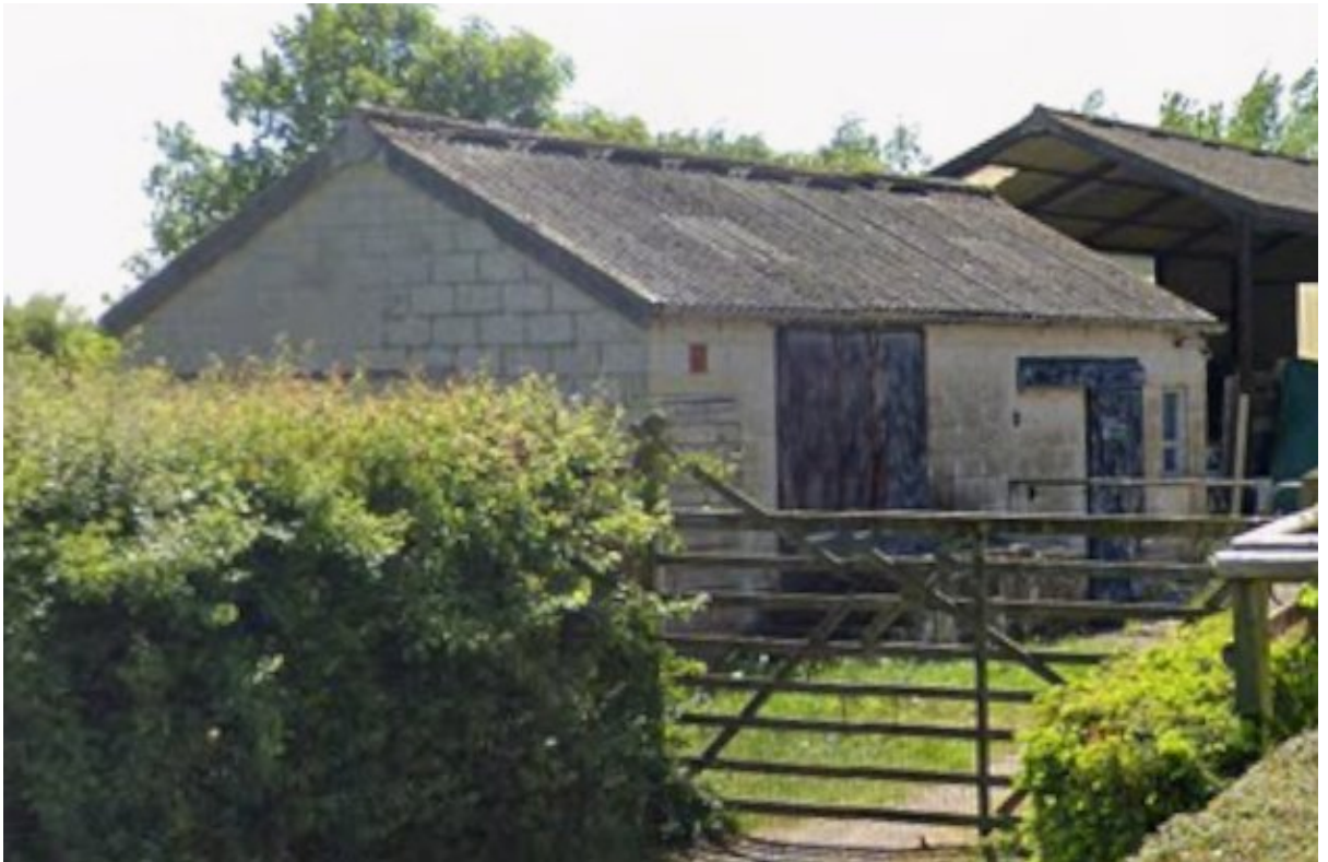
Image 6: Existing Blockwork Barn
