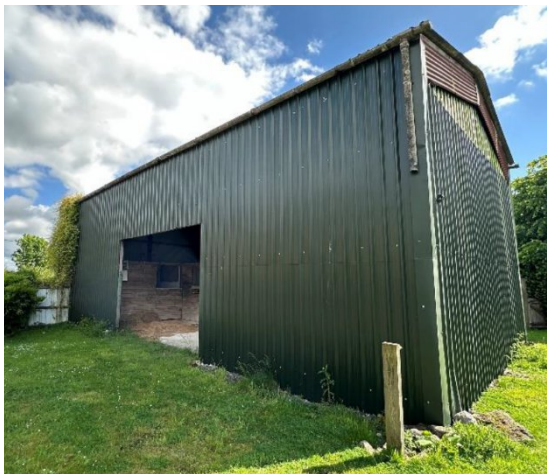
Image 4: Eastern Barn – west elevation
