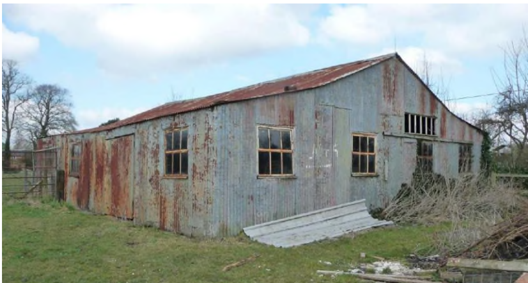
Figure 20 The workshop associated with The Malthouse prior to its conversion to ancillary residential use in 2017. (Source: D&A Statement for 17/01942/FUL).
