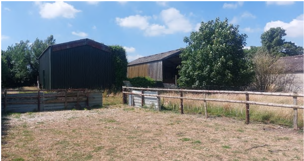
Figure 7 The agricultural sheds as seen from the north-east corner of the plot east of No. 21. From the street itself, this view is totally screened by the tall hedgerow.
