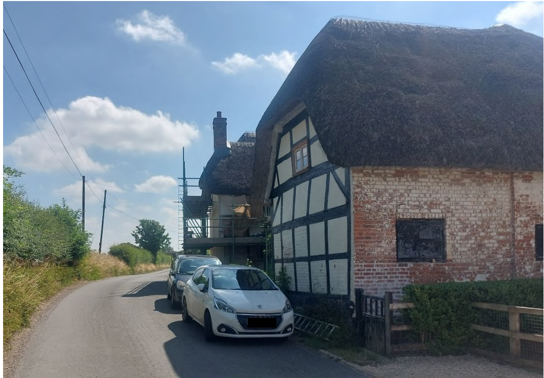
Figure 10 Further west along the village street passing The Malthouse, the position of the projecting wings of The Malthouse and the slight curve in the road means that No. 21 is concealed from view, and there is no sightline to the agricultural sheds.
