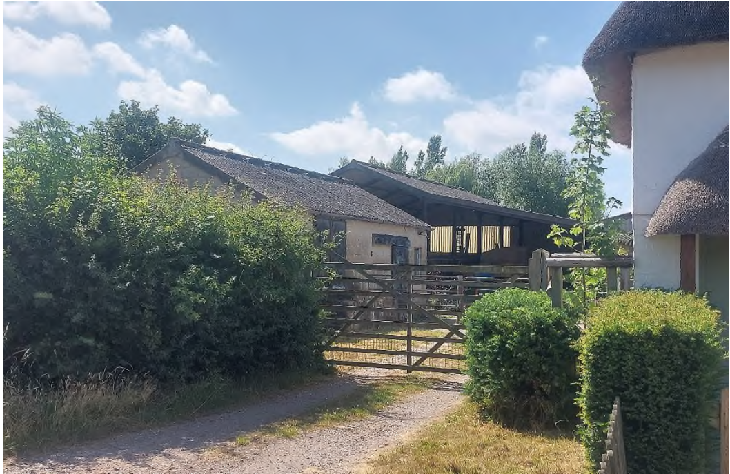
Figure 6 An angled view through the gateway to the agricultural sheds adjacent to the east end of No. 21. The part rendered block building to the front of the plot is to be demolished.
