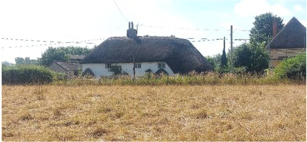
Figure 12 A footpath leads to the north from The Street west of No. 21. The path is slightly set down from the field level but from the field boundary No. 21 can be seen with the rendered blockwork shed to the left (to be demolished). The eastern shed proposed for conversion can just be glimpsed beyond, set well back from the street frontage.
