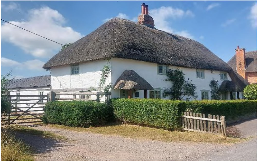
Figure 4 No. 21 The Street as seen from the north-east. That the house was formerly two cottages is evident by the presence of the two doors and porches. The character is largely as described in the list description, the early origins of the house as a cruck-framed building of possible 15 th century date is not evident from the front elevation.
