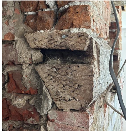
Fig.7 South-west end of beam showing cuts from a former use
