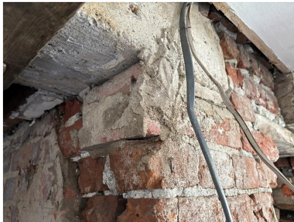
Fig.13 Concrete lintel with edge of Newtonite lath lining to left
