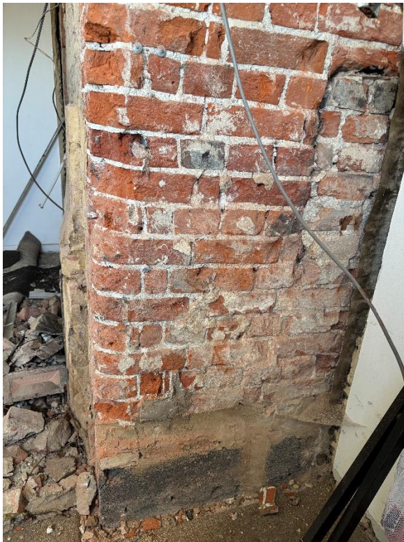
Fig.9 South-west return of fireplace with narrow recess of 6 bricks' height cut in for a flue
