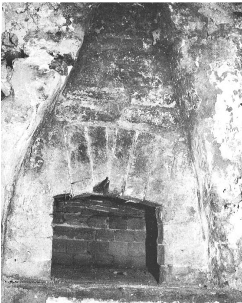
Fig.17 Bread oven in tapered recess in a farmhouse in Semington
