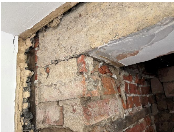
Fig.13 Concrete lintel with edge of Newtonite lath lining to left
