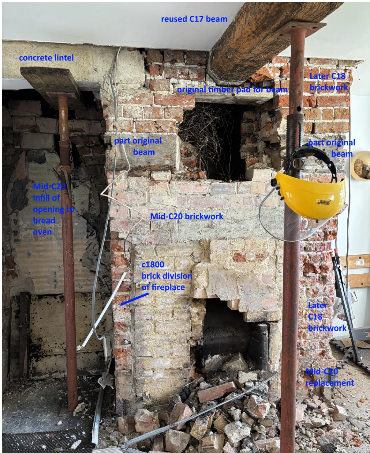
Fig.6 Main hearth at ground floor level
