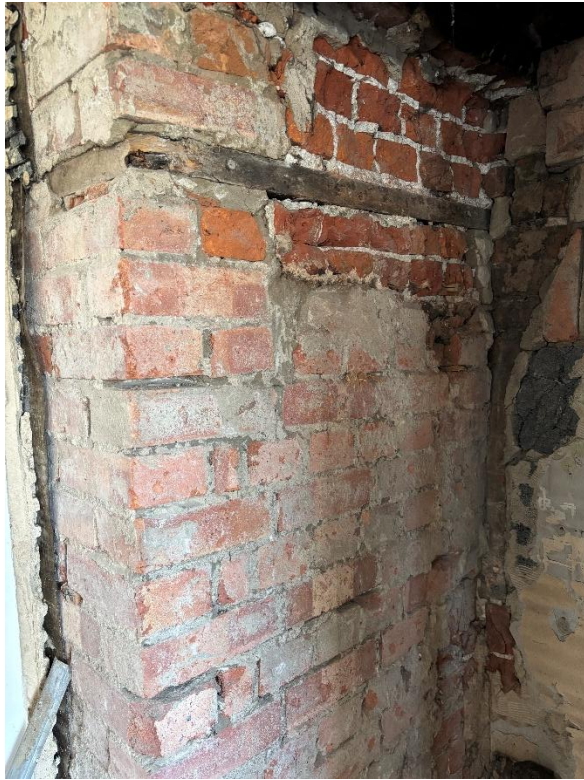
Fig.11 The original north-east wall of the fireplace, showing a remaining timber levelling course
