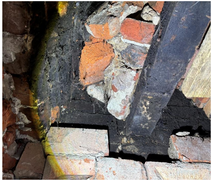
Fig.15 Junction of later partition with back wall of hearth
