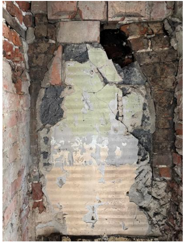
Fig.11 The original north-east wall of the fireplace, showing a remaining timber levelling course
