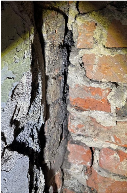
Fig.15 Junction of later partition with back wall of hearth
