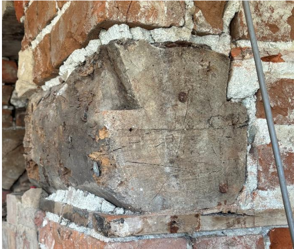
Fig.7 South-west end of beam showing cuts from a former use
