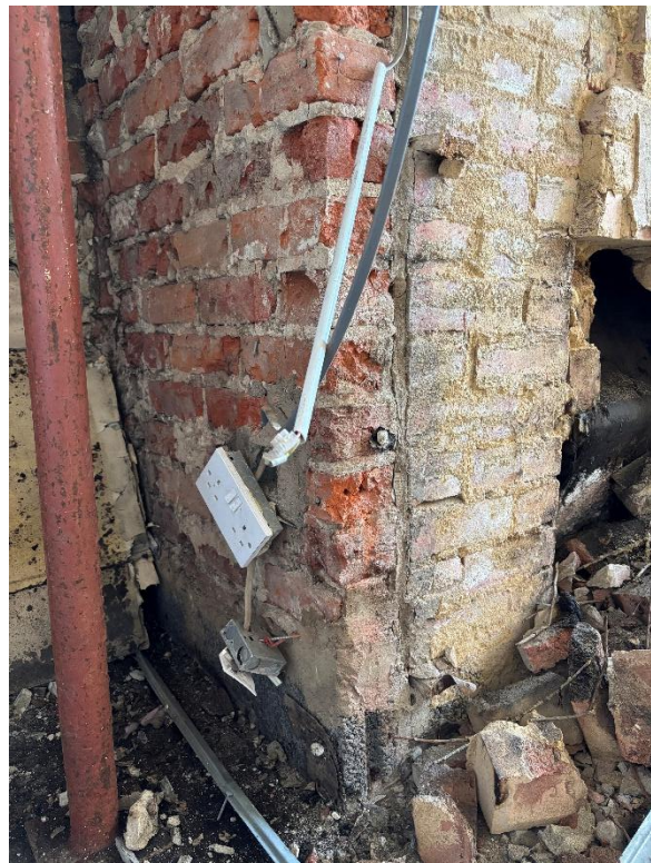
Fig.9 South-west return of fireplace with narrow recess of 6 bricks' height cut in for a flue
