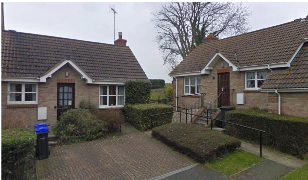
Figure 1: Front elevation of subject properties, (No. 9 on LHS & No. 10 on RHS)
