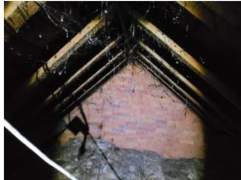
Photo 6: An internal view of the loft void.
