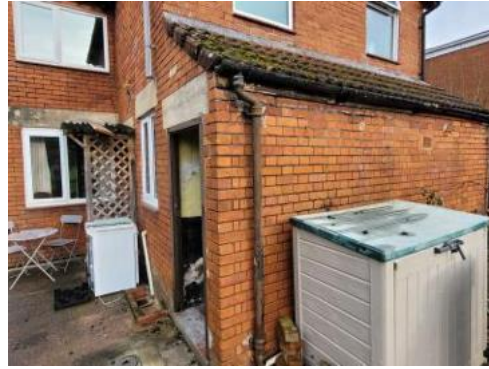
Photo 8: View of the WC building which adjoins southern elevation.
