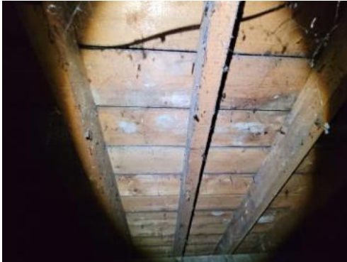
Photo 7: Wooden boarding beneath tiles.
