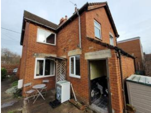
Photo 1: View of the building from the south-west.
