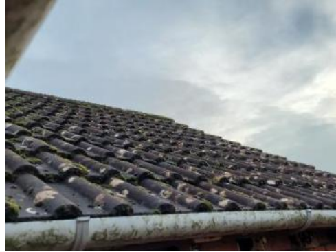
Photo 2: Well fitted concrete interlocking tiles.
