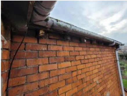
Photo 3: View of the eaves along the southern elevations.
