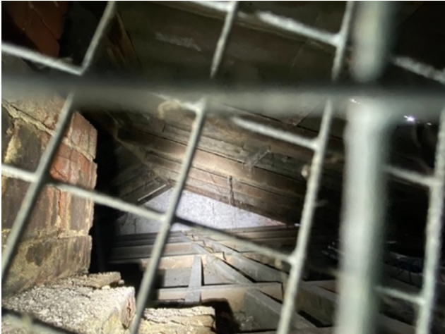
Image 13: Void space above utility room connected to the garage through metal mesh.
