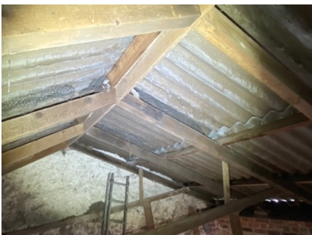
Image 11: Interior garage roof.
