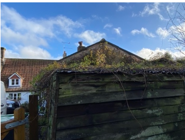
Image 5: Western aspect of lean-to at western gable.
