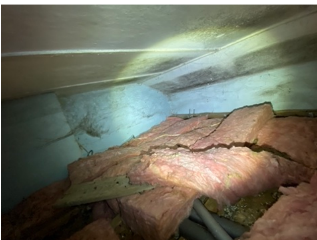
Image 17: Utility room loft.
