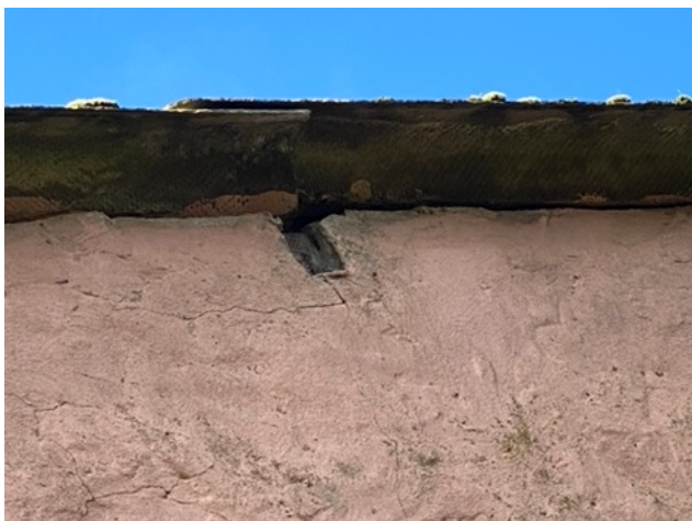
Image 9: Crevice leading above wall plate to the purlin on the east gable
