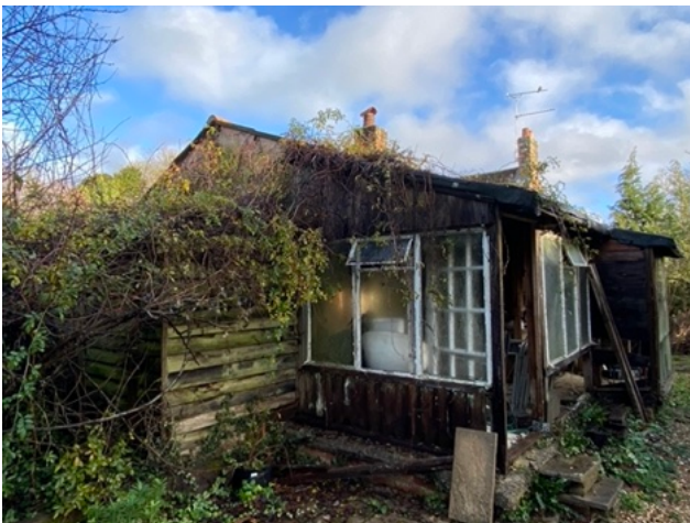
Image 3: Southwest aspect of the southern wooden lean-to with open door.
