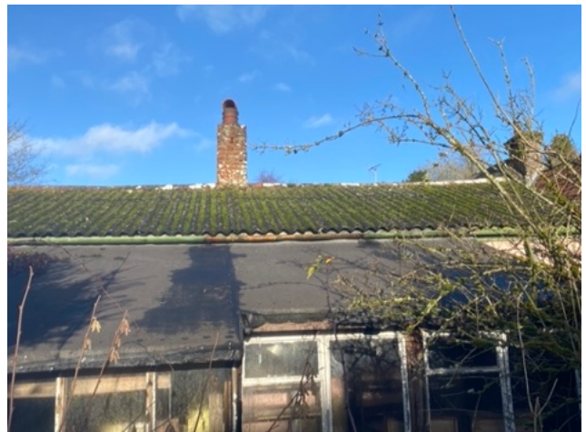
Image 4: Southern aspect of garage and lean-to roofs.
