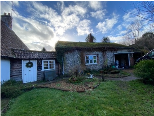
Image 1: Northern aspect of target building showing garage and eastern link structure.
