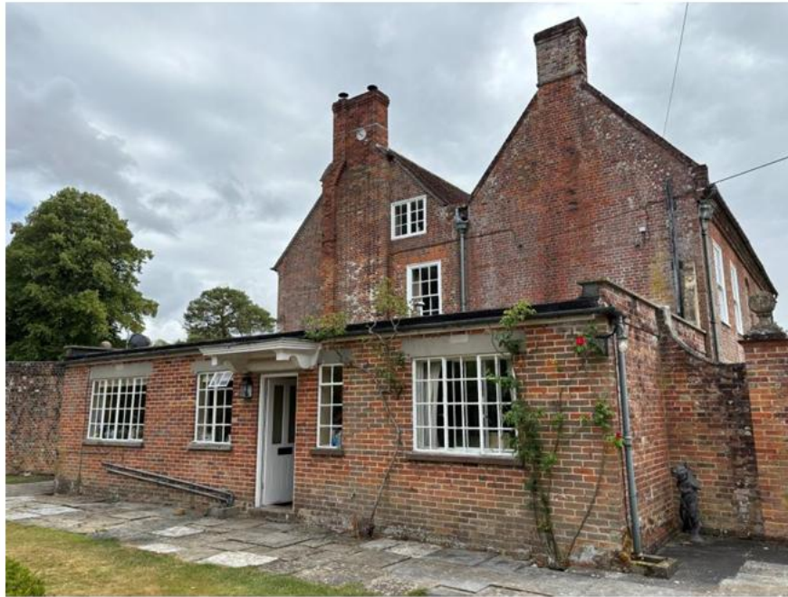
Fig.6 Single-storey flat-roofed extension on the northern end of the house – note the Crittal windows with concrete lintels and cills
