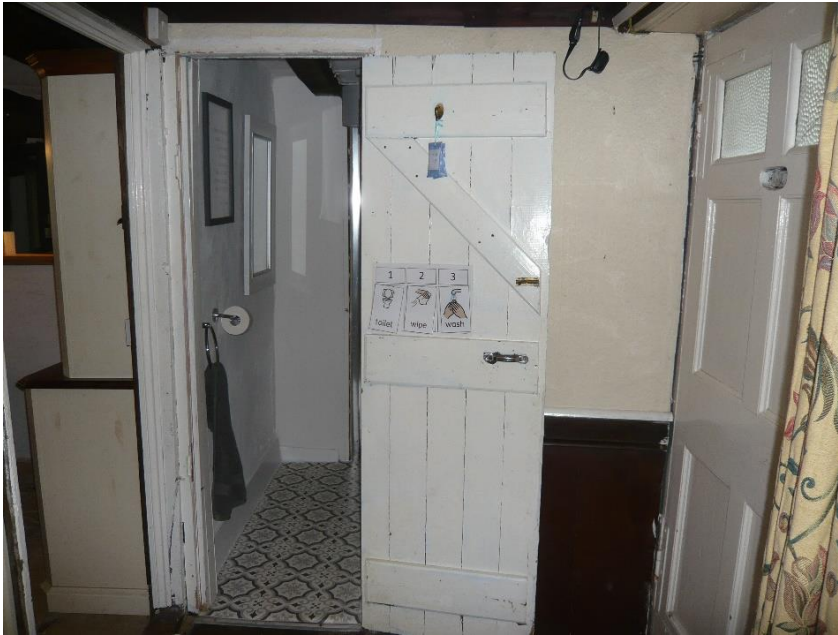
Modern partition to the WC next to the front entrance
