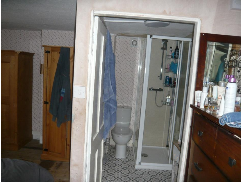
Modern partitions to the en-suite bathroom at the southern end of the first floor
