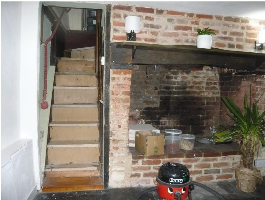
Precipitously steep staircase adjacent to the fireplace within the cross-wing
