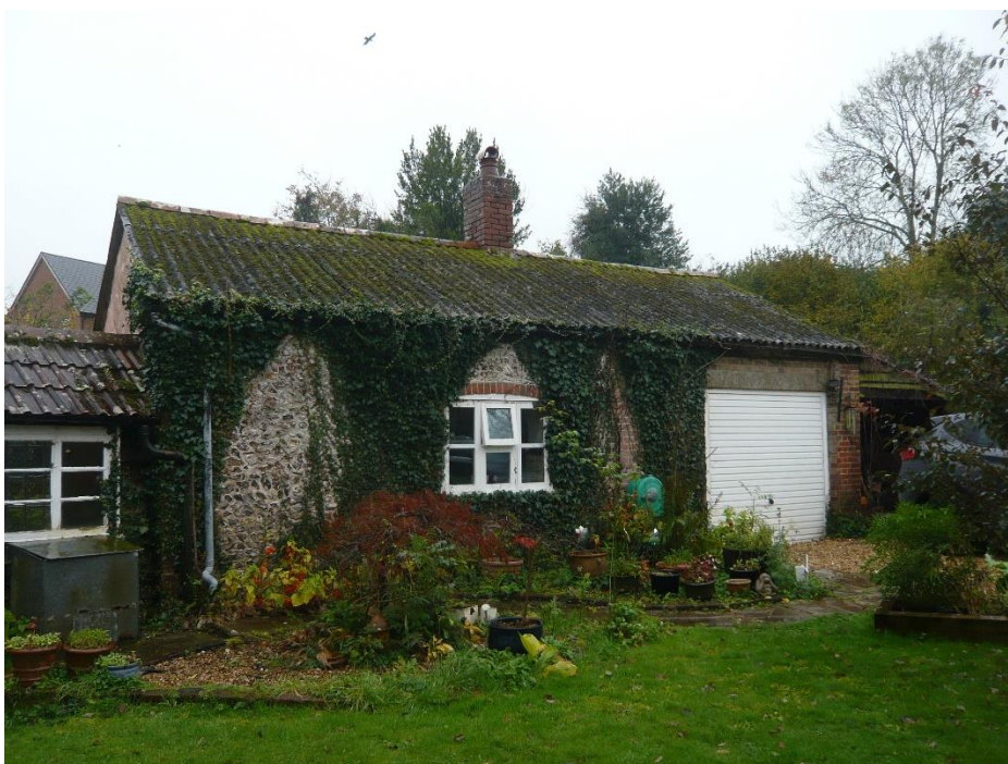
Garage building proposed for demolition
