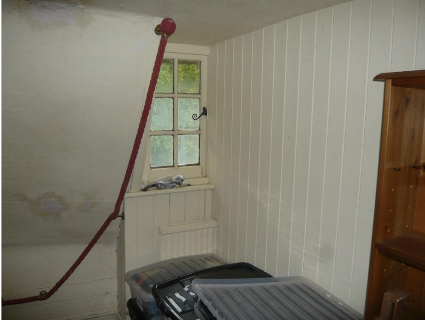
Boarded partition cutting across the casement window
