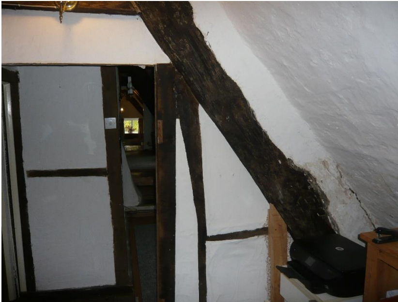
1960s faux timber-frame partition on the left
