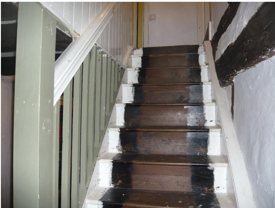
Fig.12 Secondary staircase within the northern end of the house
