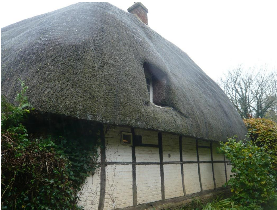
Fig.4 Exposed timber-framed north wall as seen from Back Drove
