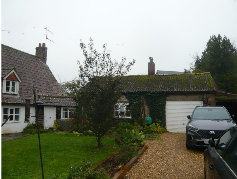
Fig.30 Looking towards the north side of the barn from the rear garden
