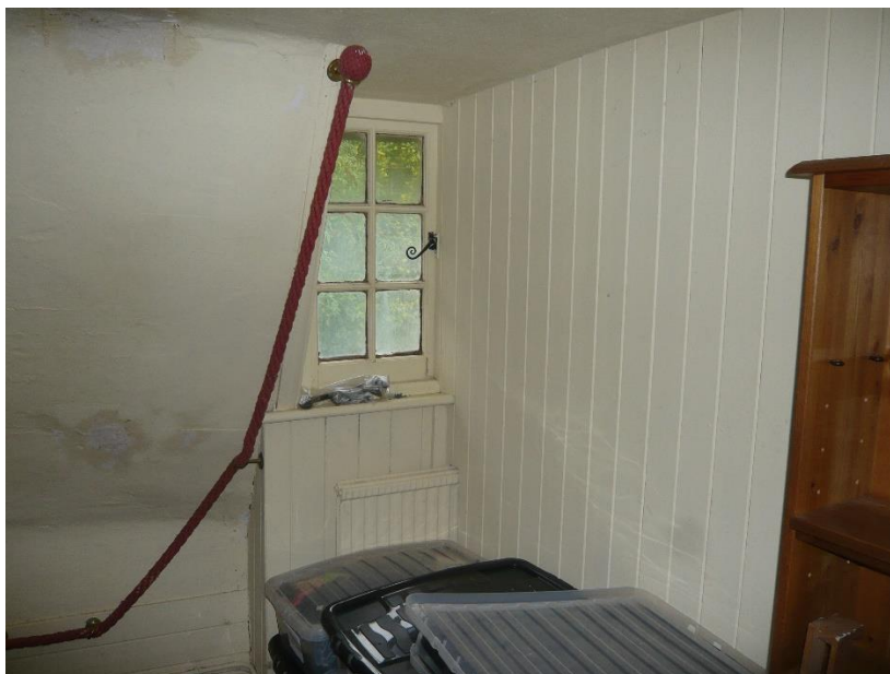
Fig.26 Early C20 matchboard partition within the first floor of the former dairy range
