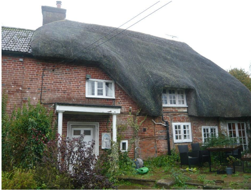
Fig.17 C18 six-panel front door within C19 flat-roofed canopy porch
