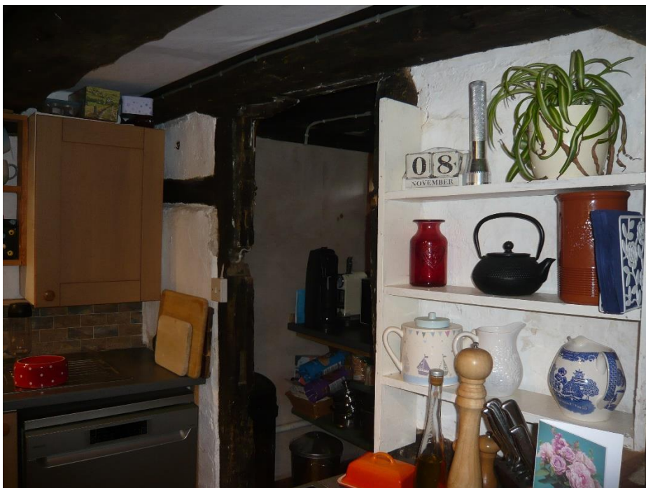
Fig.10 Timber-framed Pantry wall
