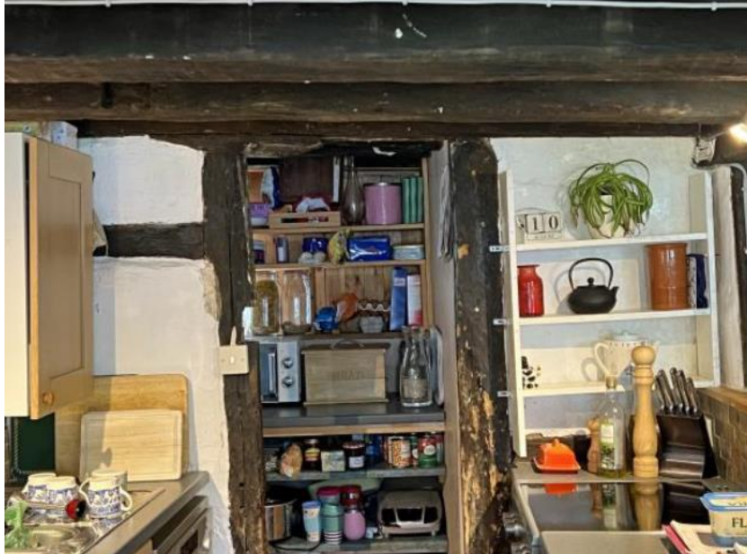
Fig.21 C15 timber-framing of the Pantry - former loft stair/ladder space
