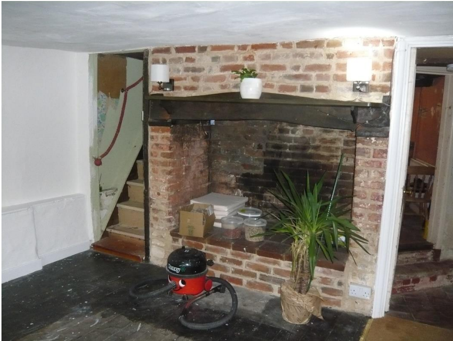
Fig.15 Western room of the northern cross-wing
