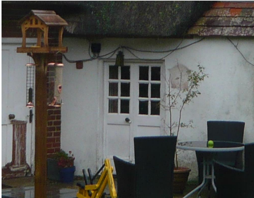
Fig.19 Early C20 half-glazed doors on the rear
