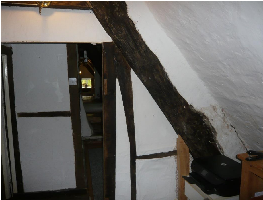
Fig.13 Lower blade of one of the original cruck trusses
