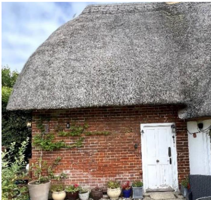
Fig.18 Inserted early C20 door to the dairy; original opening was to the left
