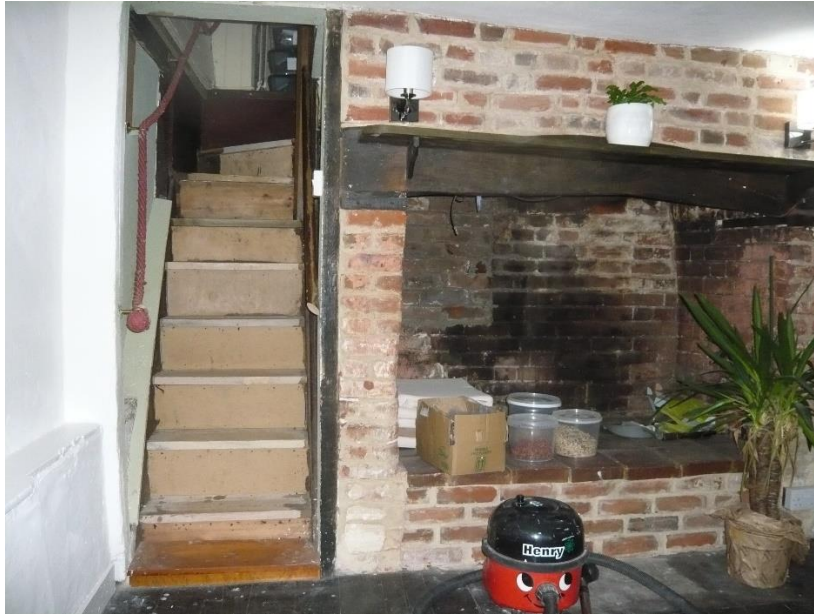
Fig.25 Steep C18 staircase within the former dairy range
