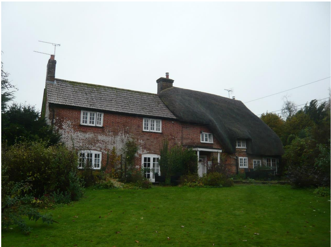
Fig.3 Front of Kings Farm
