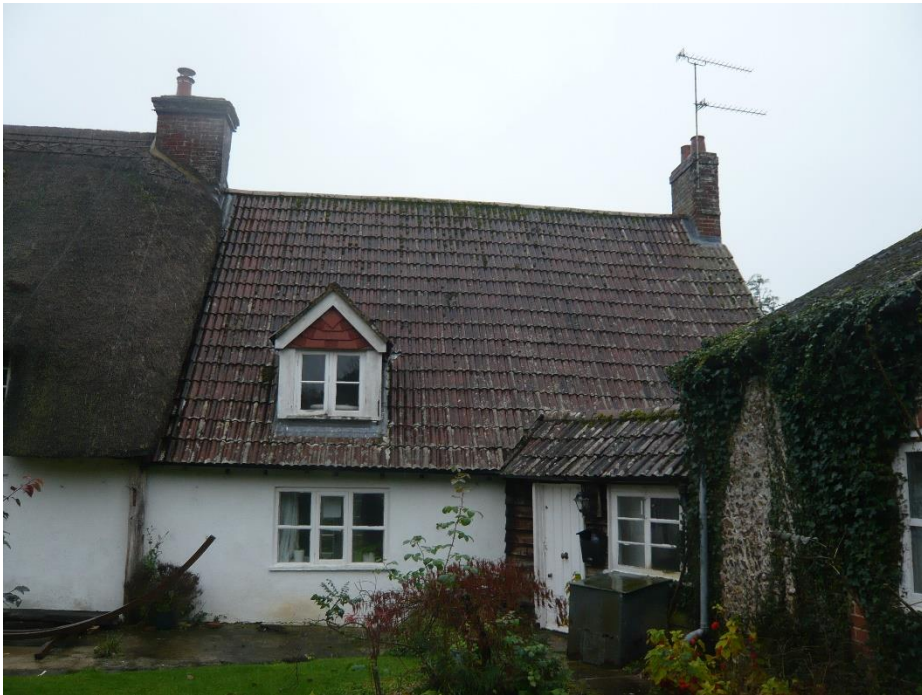
Fig.6 Rear of the tiled element
