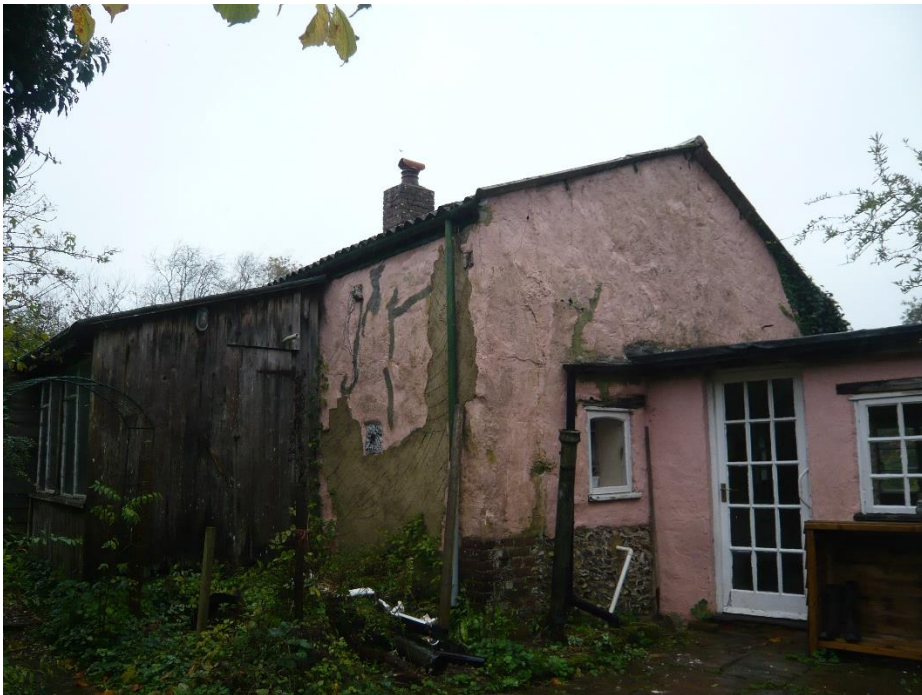
Fig.7 Link and barn attached to the south-west of the house
