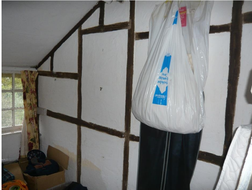
Fig.27 Early C20 faux framing between Box Room and Bathroom
