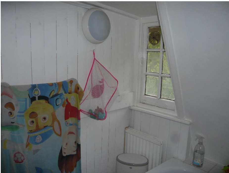
Fig.16 Matchboard partition in the first floor of the cross-wing; note the restricted ceiling height
