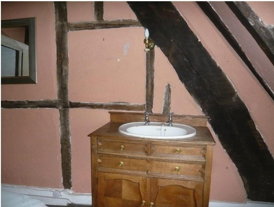
Fig.14 Some faux timber-framing in one of the first-floor bedrooms
