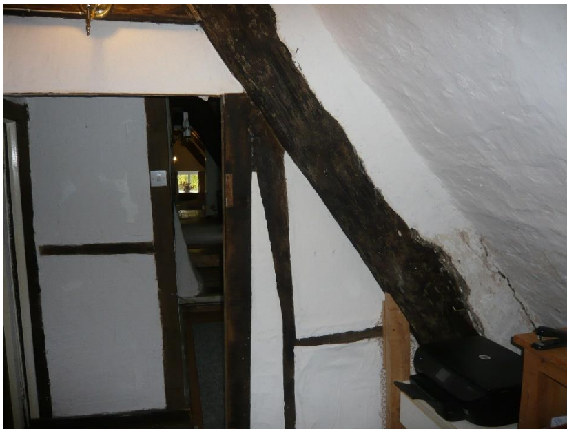
Fig.28 View looking south within the first floor corridor – 1960s faux timber-frame partition on the left
