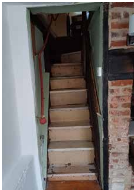
Annexe staircase to form quirky storage cupboard
