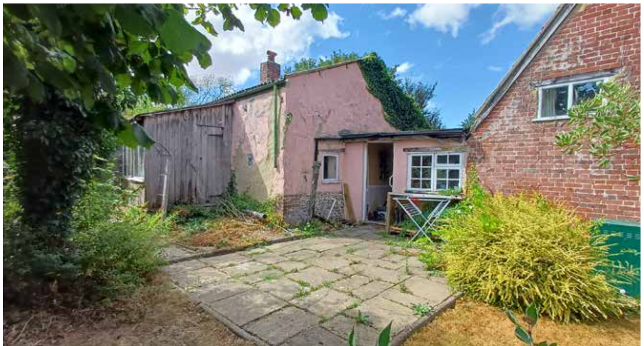
South range and link from south east with linking space against the house
