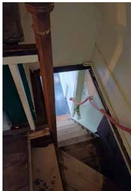
Annexe staircase from above. Trapdoor will cover over stair void
