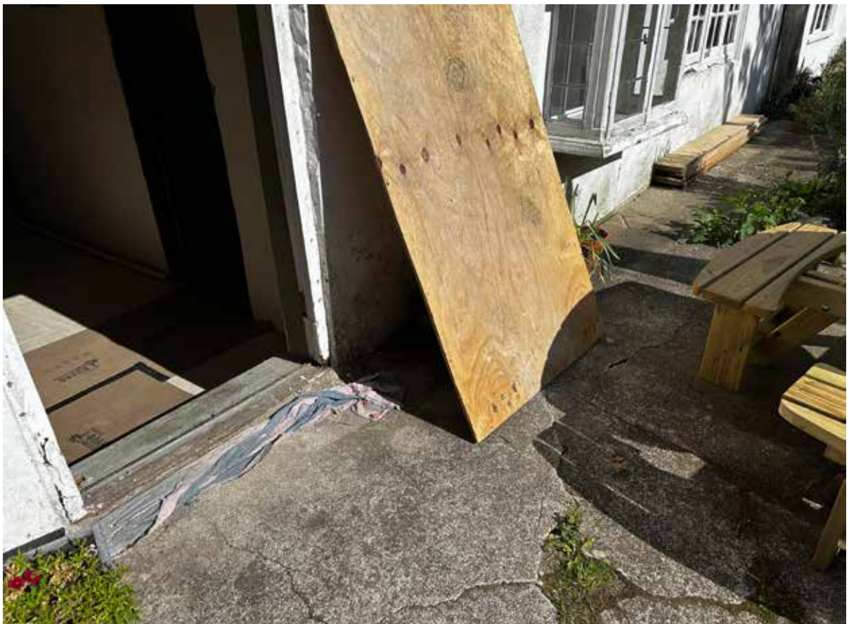
Raised ground levels externally in a concrete hardstanding with cement rendered walls
