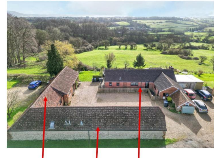
The Byres, Mead View and the wider residential group
