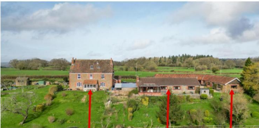
Westbrook Farmhouse, The Flat, Mead View and The Byres an established group of buildings and houses
