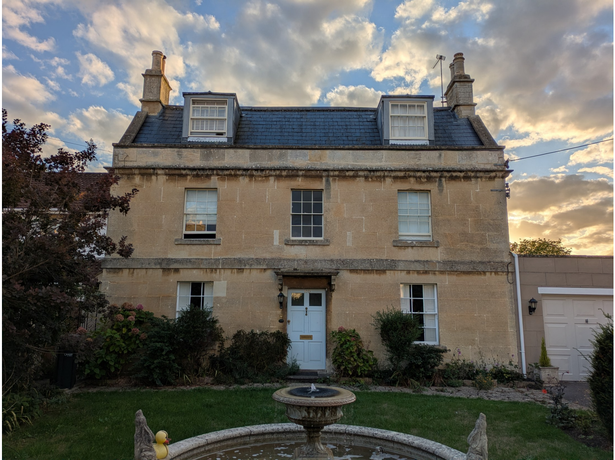
Figure 4. Wider view showing the detached house, formal principal elevation and relationship of the central entrance to the adjoining garage and garden.
