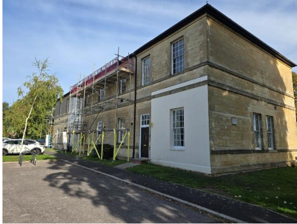
P1 – Cedar House Front Facade
