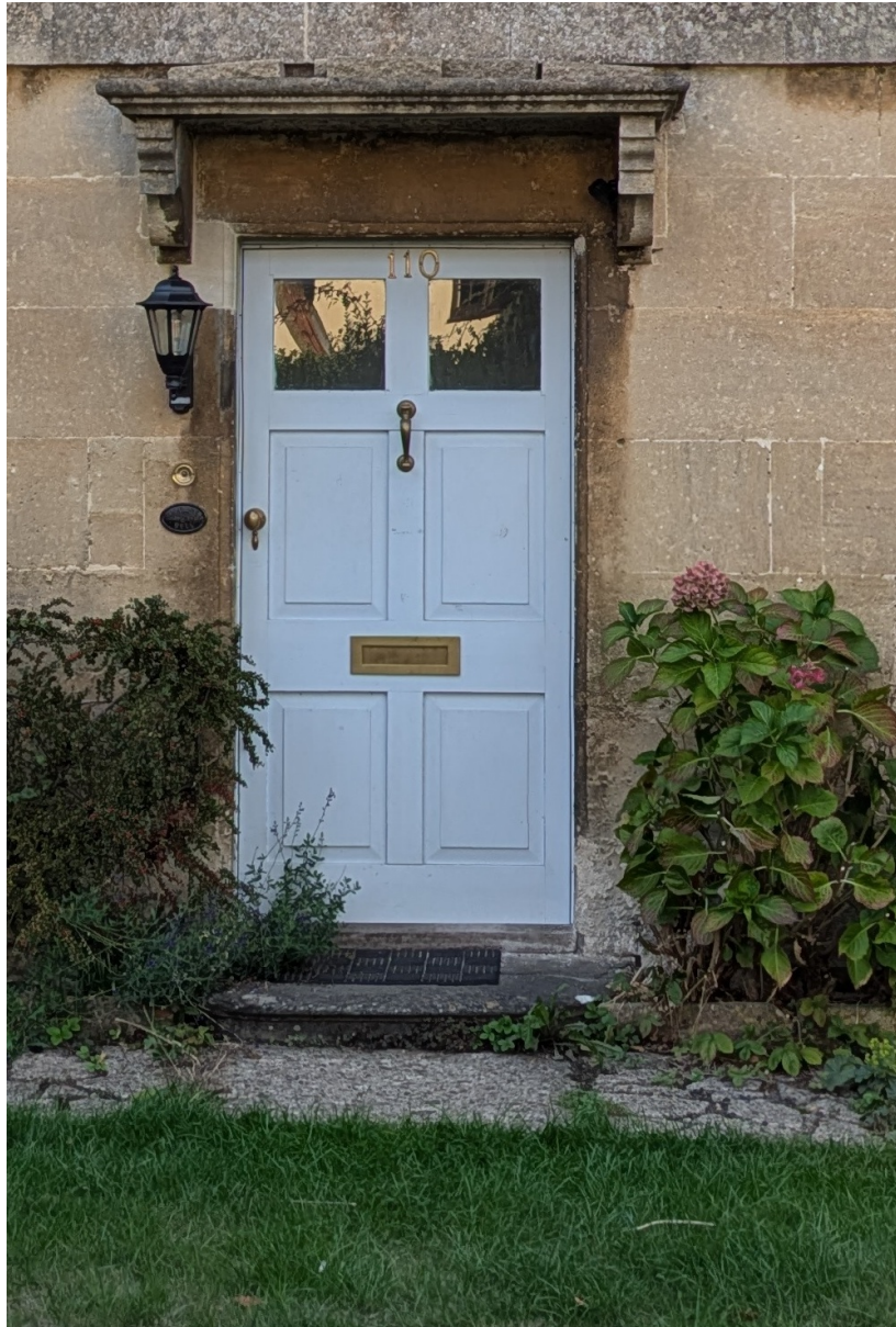
Figure 3. Existing central C20 glazed door within the chamfered stone opening.
