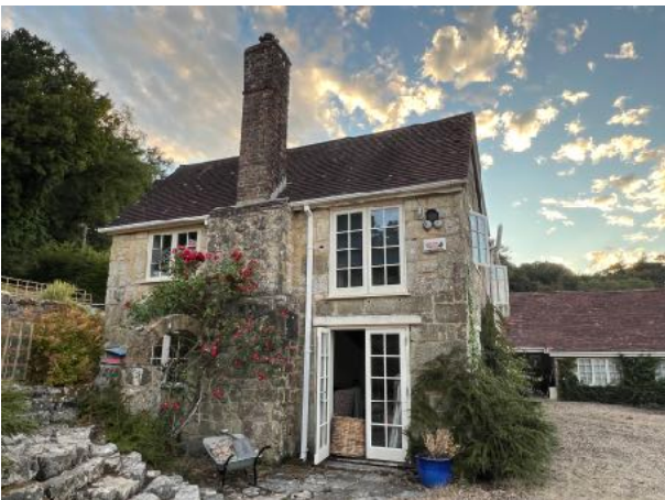
Figure 5 - SE elevation of cottage
