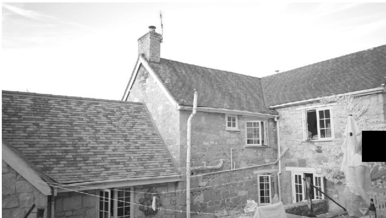
Figure 22 - Camera 1 13/08/2026 NW & SW elevations. Start of dusk emergence survey
