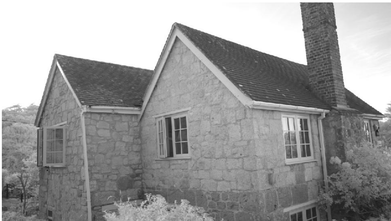
Figure 24 - Camera 2 13/08/2026 SW & SE elevations. Start of dusk emergence survey
