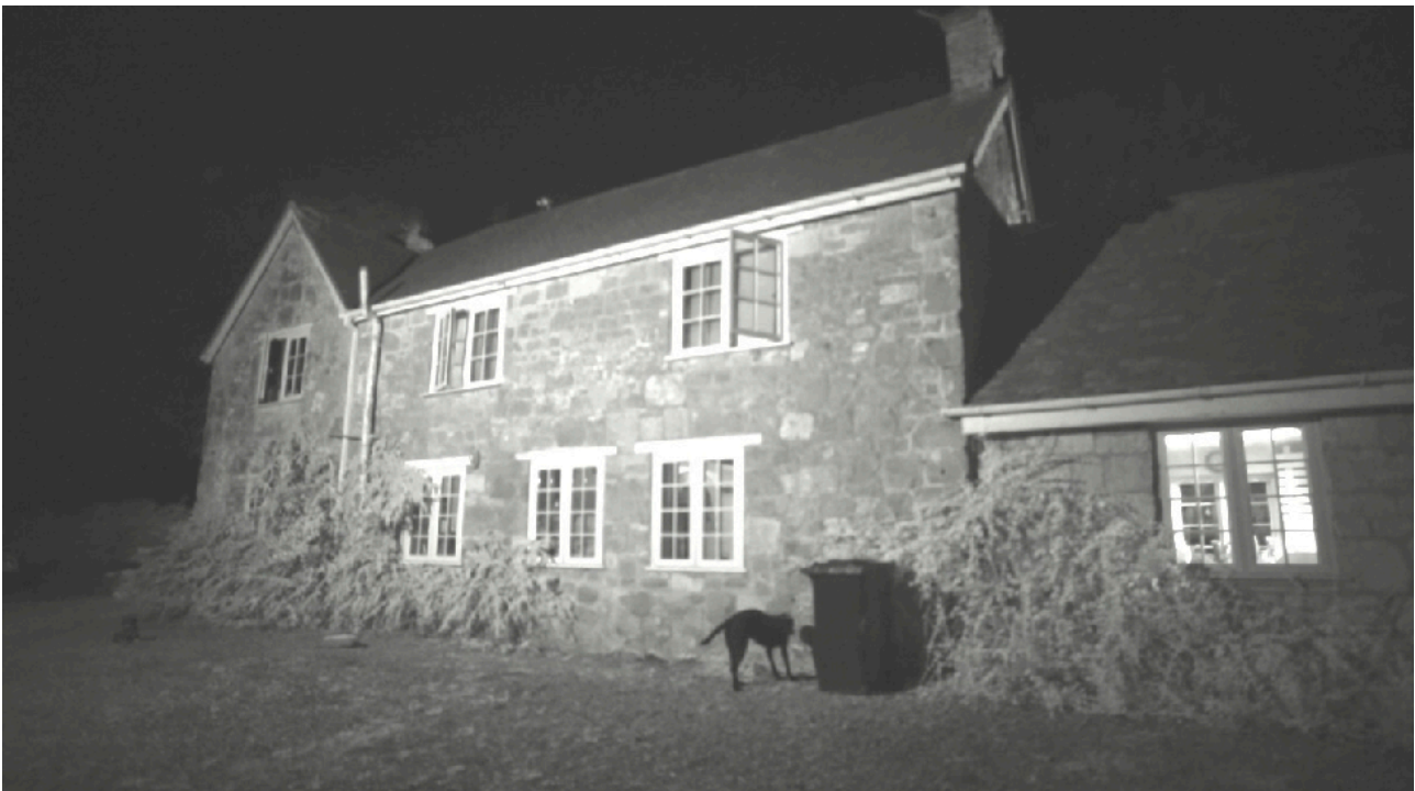
Figure 21 - Camera 3 28/07/2026 NE elevation. End of dusk emergence survey
