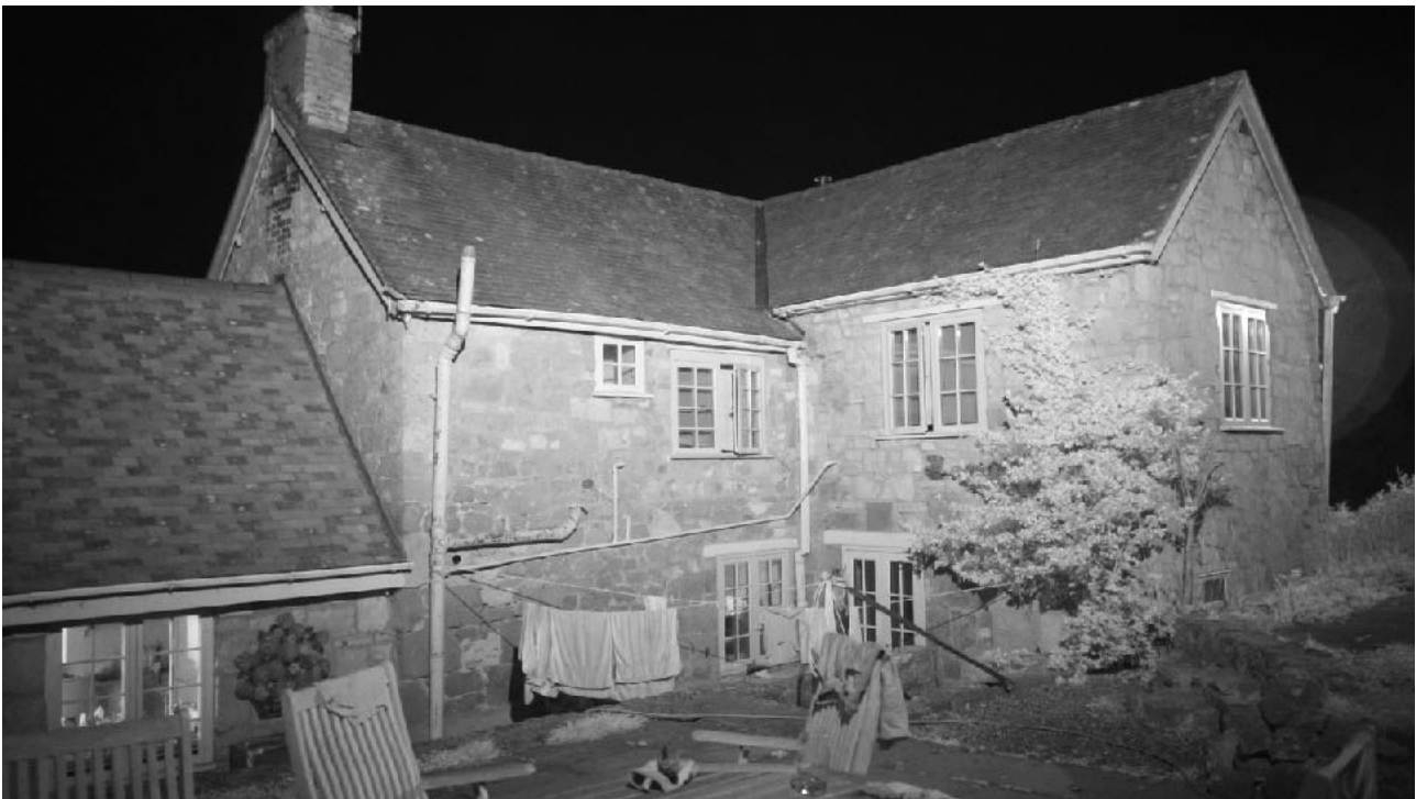
Figure 17 - Camera 1 28/07/2026. SW & NW elevations end of dusk emergence survey
