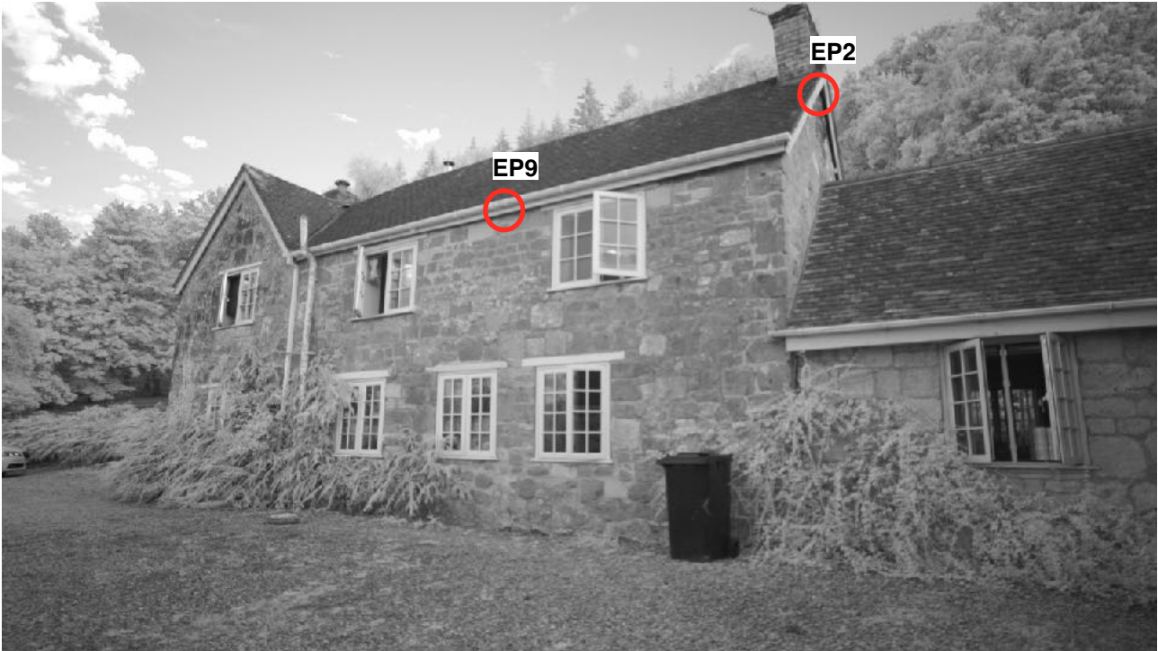
Figure 34 - Cottage NE and NW elevations - Exit points 2 and 9. 28/07/2026 (Red circle: soprano pipistrelle bats)
