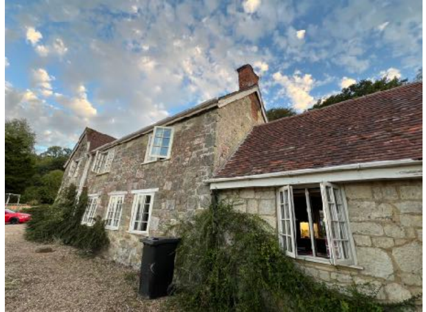
Figure 2 - NE elevation of cottage
