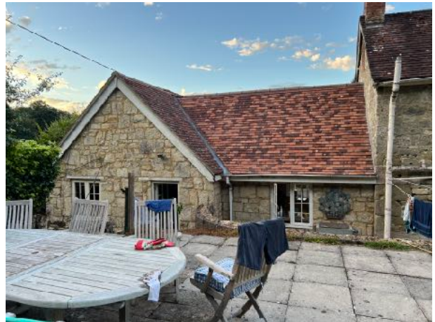
Figure 8 - SW elevation of cottage
