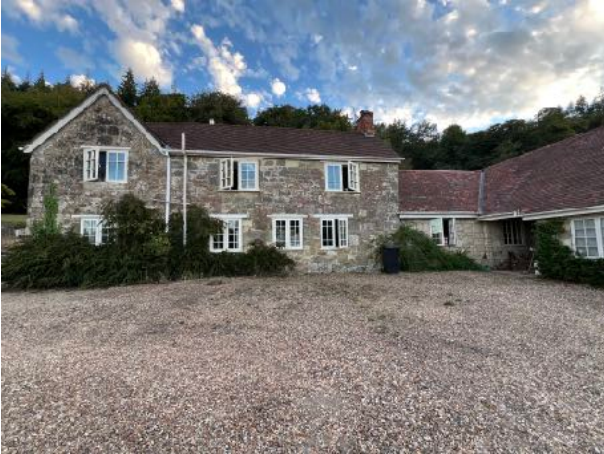
Figure 1 - NE elevation of cottage
