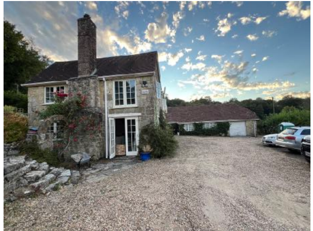
Figure 4 - SE elevation of cottage
