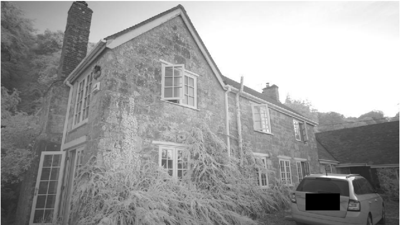
Figure 26 - Camera 3 13/08/2026 SE & NE elevations. Start of dusk emergence survey
