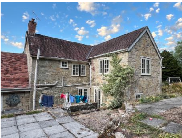
Figure 9 - SW elevation of cottage
