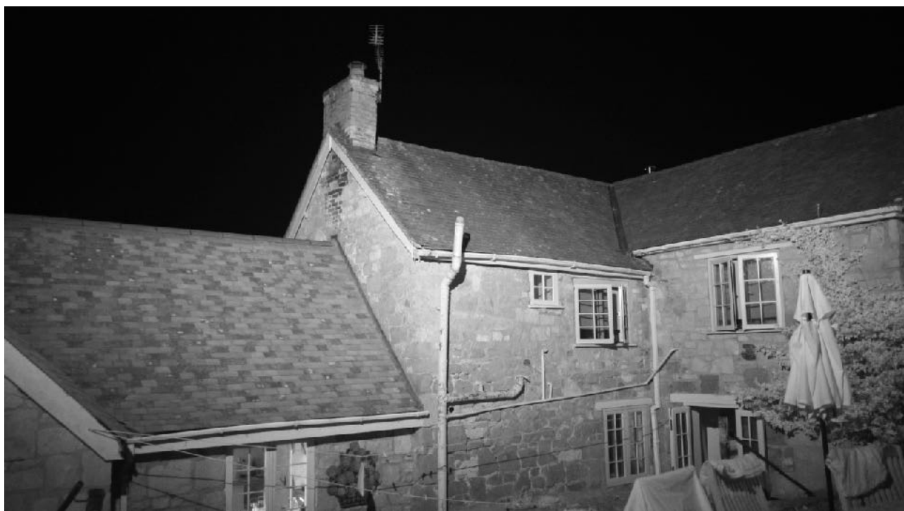
Figure 23 - Camera 1 13/08/2026 NW & SW elevations. End of dusk emergence survey
