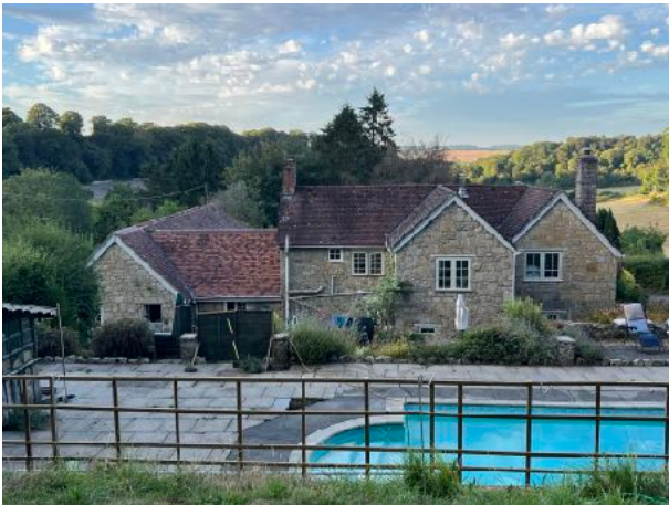
Figure 7 - SW elevation of cottage
