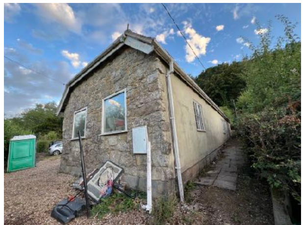
Figure 10 - NE and NW elevations of garage
