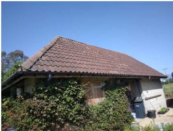
Building B1 - Eastern elevation
