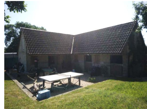
Building B1 - Northern and western elevations
