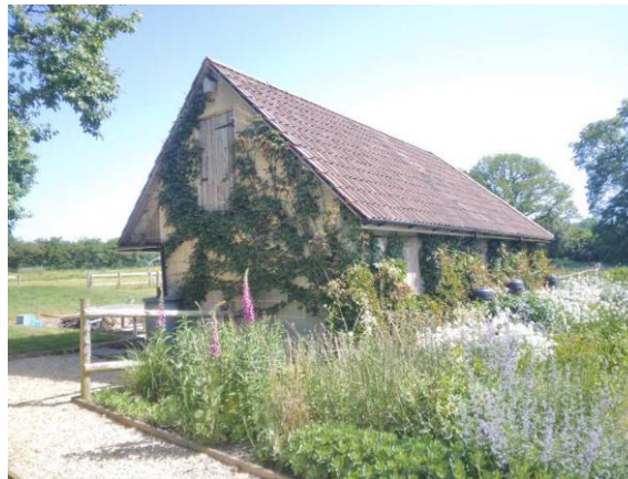
Building B1 - South-western elevation
