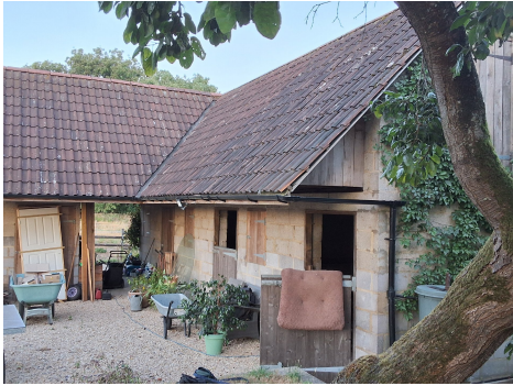
V1 B1-2 surveyor photo
