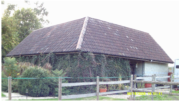
V3 B1-3 surveyor photo
