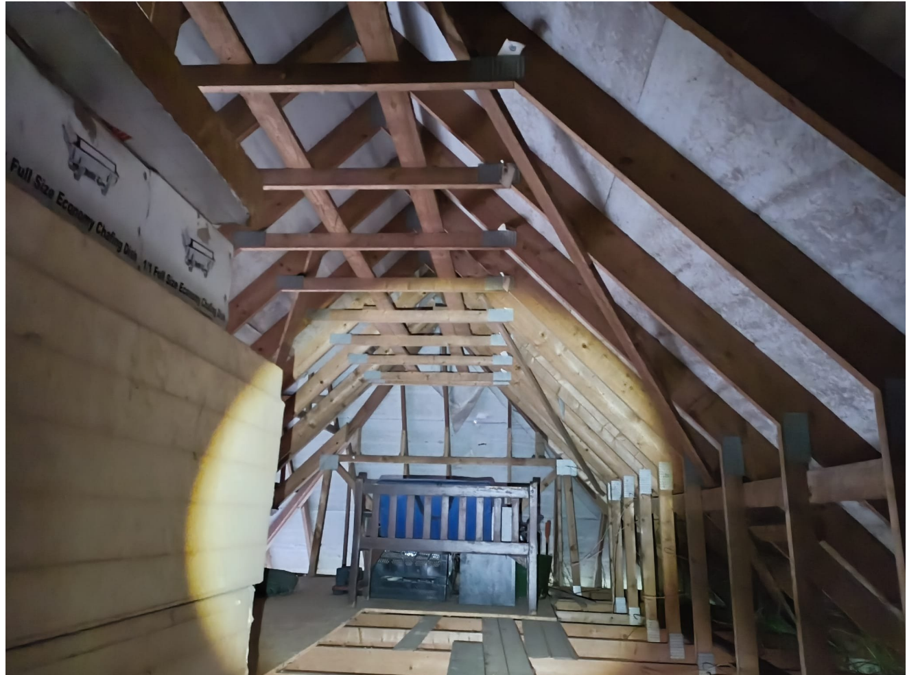
Figure 1a: Interior loft space of B1.
