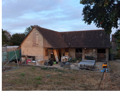
V2 B1-1 surveyor photo
