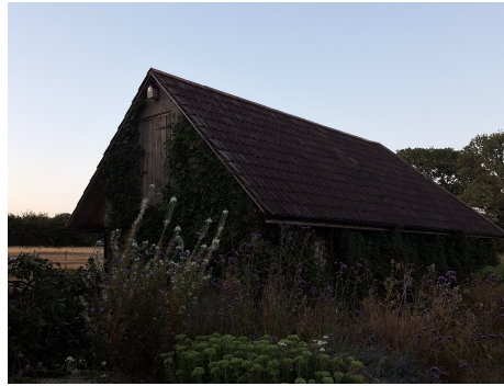
V1 B1-4 surveyor photo
