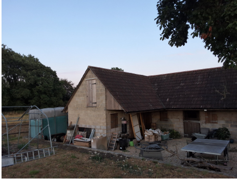
V1 B1-1 surveyor photo
