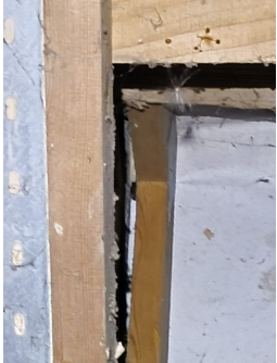
Internal space of B1. Bat identified inside B1 at the westernmost end between timber framing.
