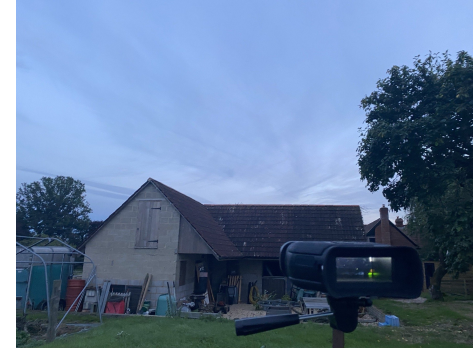
V3 B1-1 surveyor photo
