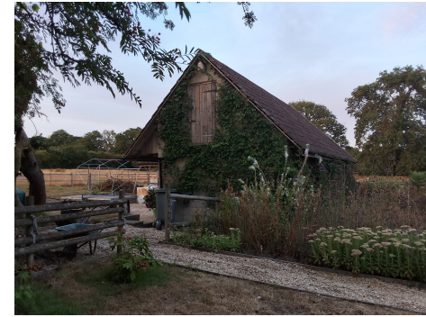
V2 B1-4 surveyor photo
