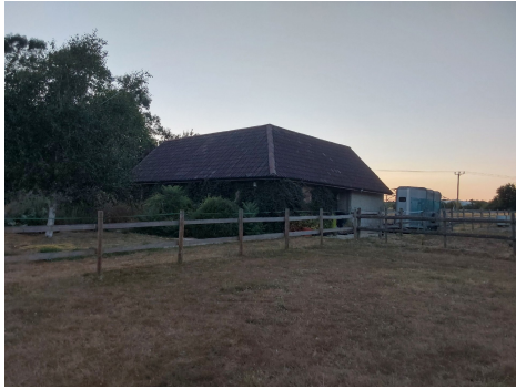
V1 B1-3 surveyor photo
