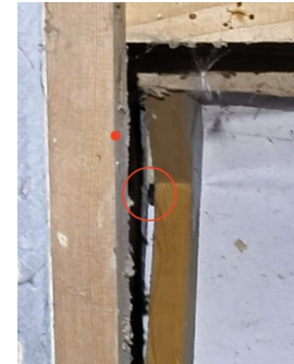
Roost 2 (B1) - bat found internally during updated inspection
