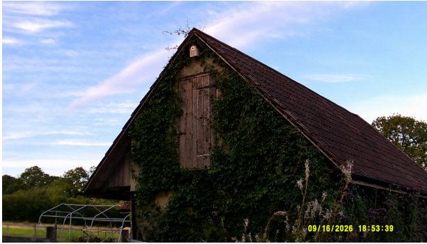
V3 B1-4 surveyor photo
