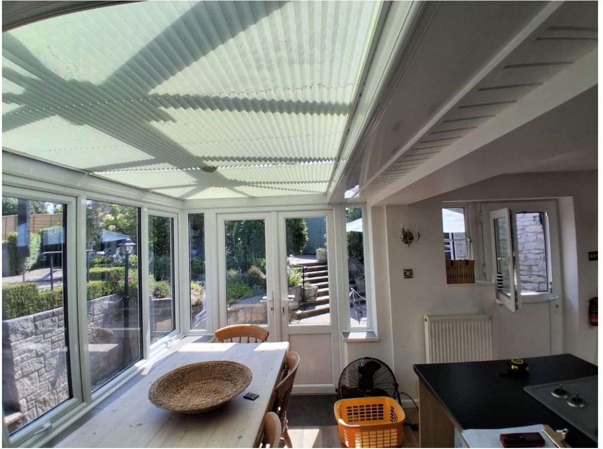
Fig7. Existing conservatory and kitchen
