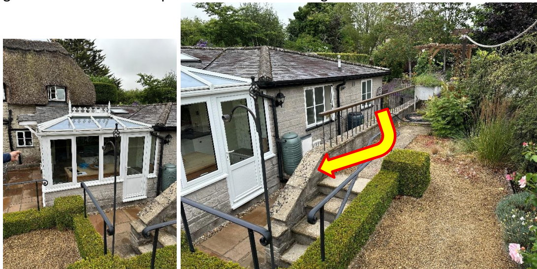
Fig.2 & 3 Rear view of existing extension and retaining wall to be re-sited (indicated)
