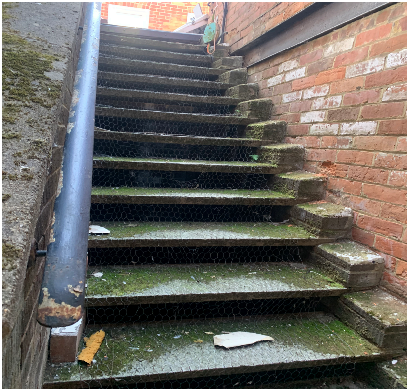
Concrete slab steps to be removed and replaced with new powder coated metal staircase
