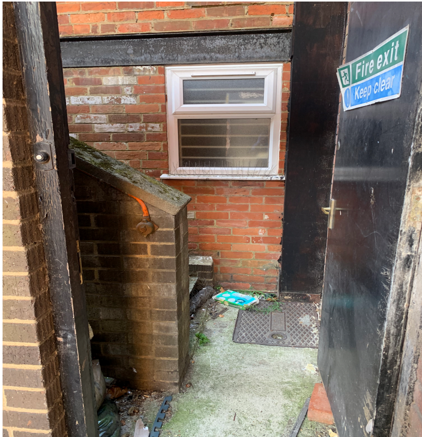
Removal of UPVC window along with brickwork nib to make way for new store entrance
