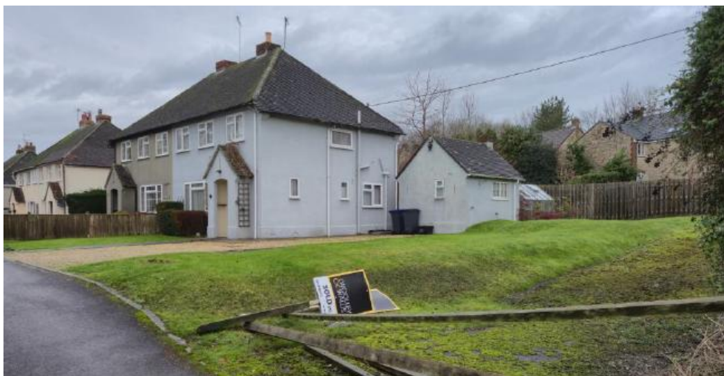
Photo of No 1 Old Hollow and adjacent land
