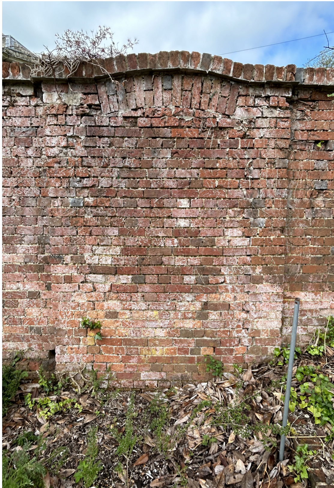
Figure 20. On the west face of the wall, the historic opening is closed by bonded brickwork
