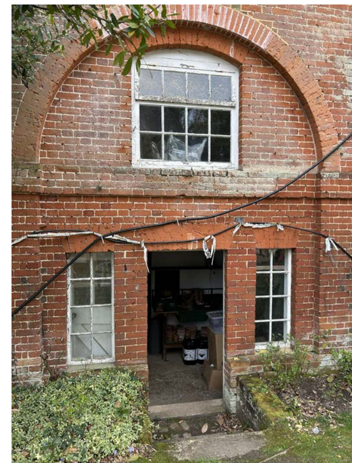
Figure 32. Raised ground levels to eastern side of Coach House, and truncated proportions
