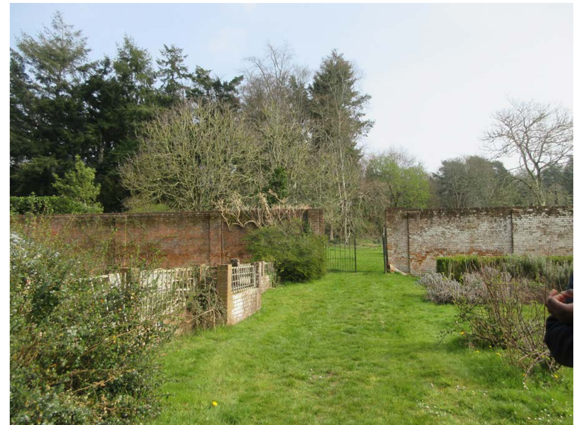
Figure 41. Section of wall removed for vehicular access
