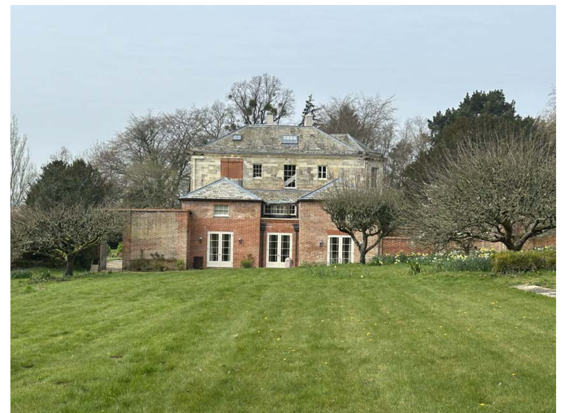
Figure 26. View towards newly revised service range
