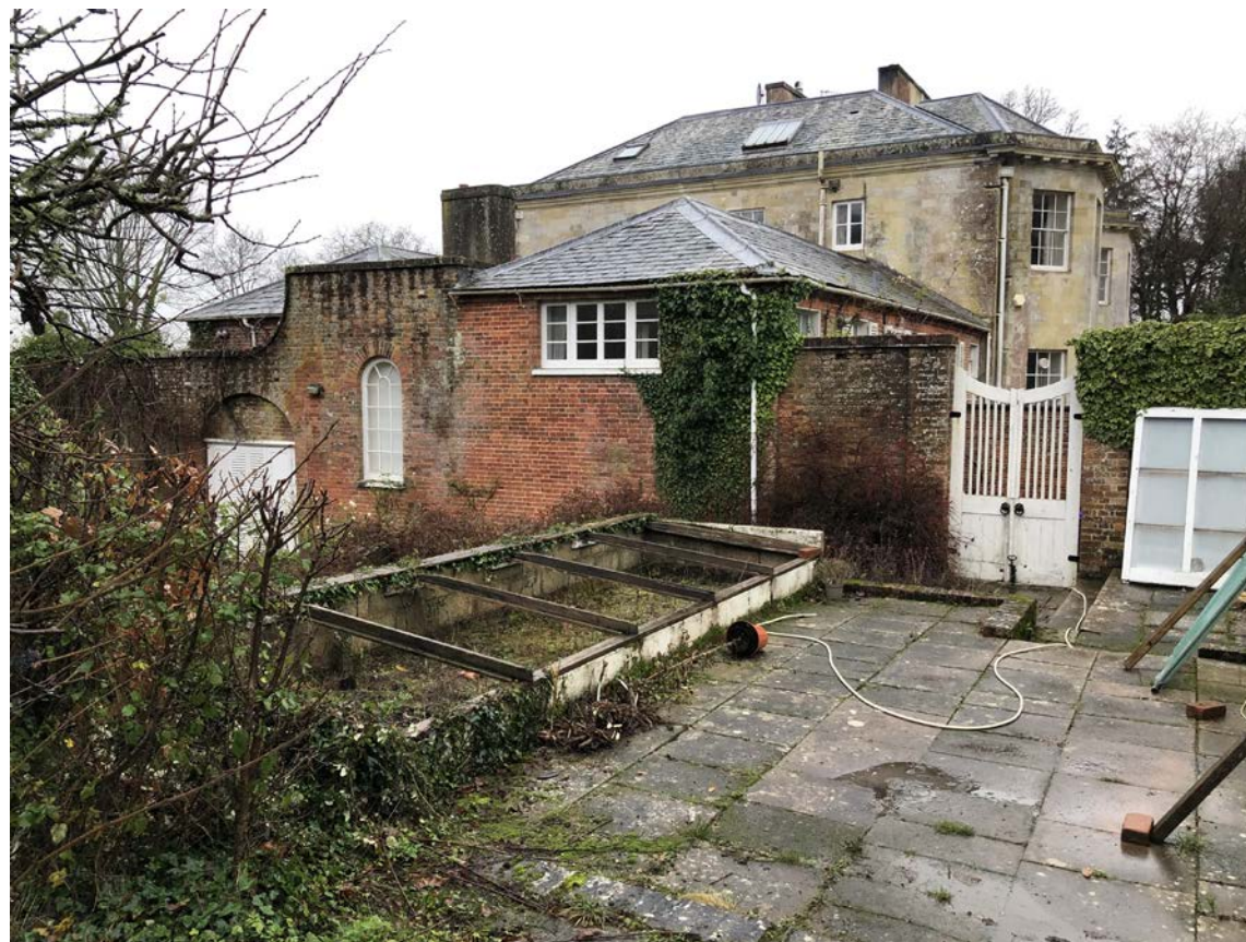
Figure 16. The C20th gateway opening to the right prior to the commencement of the works.
