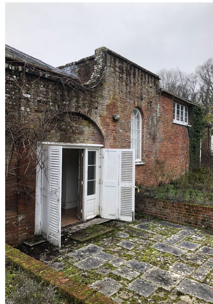
Figure 01. South service range east elevation, with a muddle of different levels and steps in combination with the assorted 1960's fenestration
