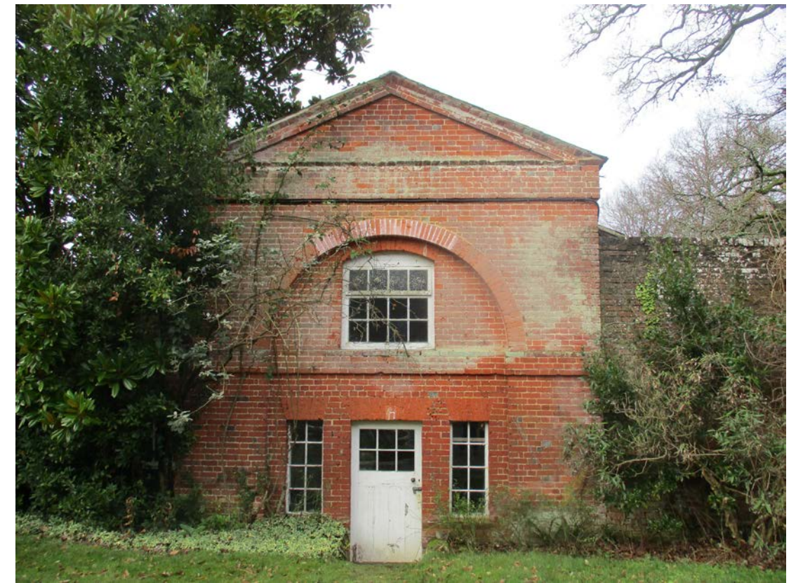
Figure 29. East elevation of the Coach House
