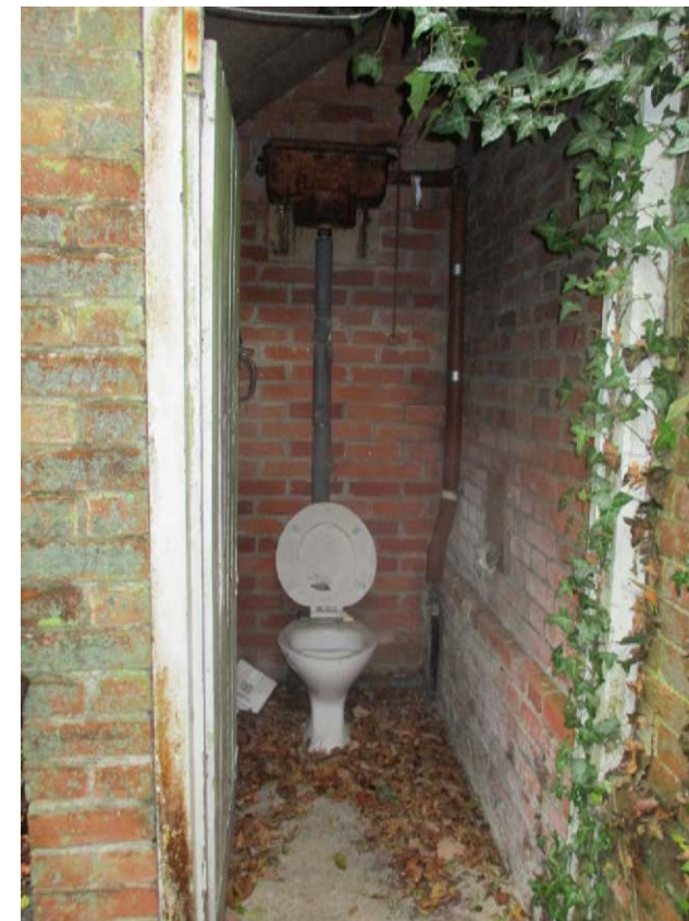
Figure 36. Gardeners WC along garden wall north of the Coach House
