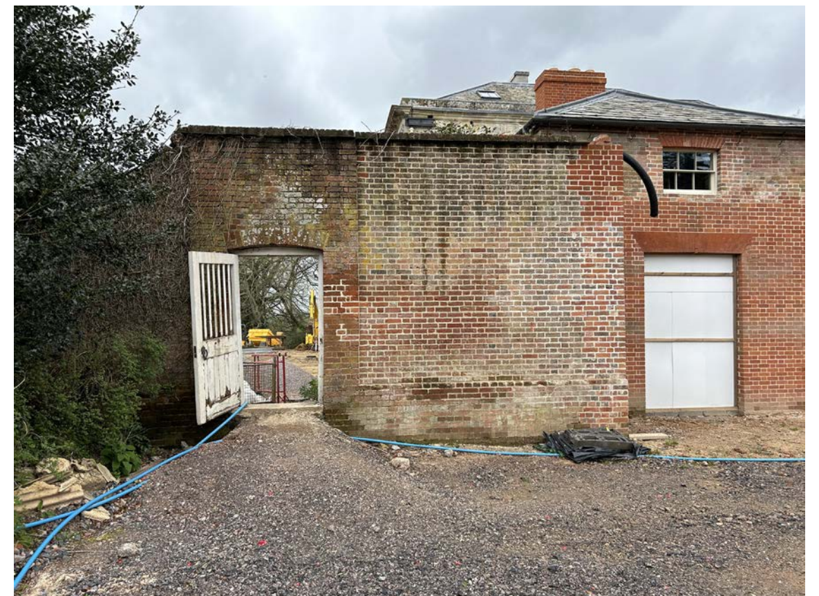
Figure 17. Cockerell period door opening to the SW, which is set in a thicker brickwork panel
