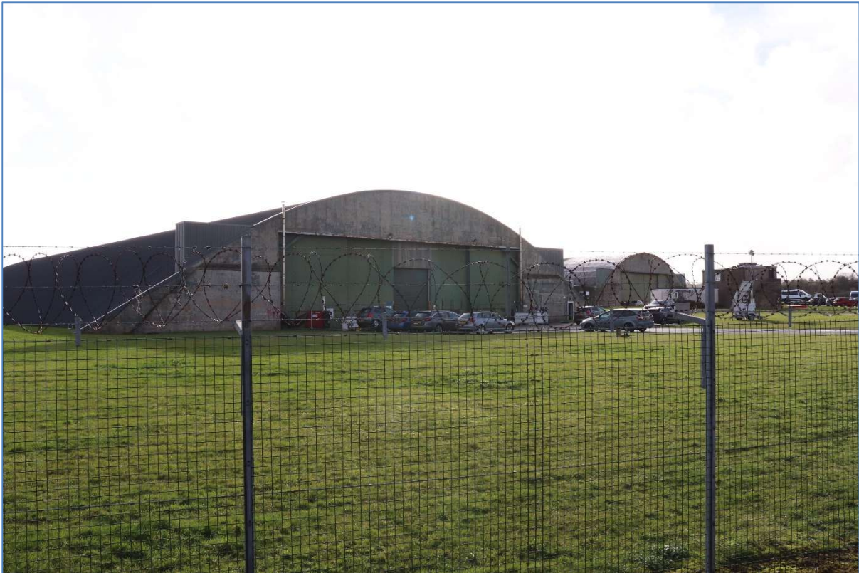
Plate 22 The L Type hangars at Priddle's Site 4, in January 2026, illustrating that their 'ears' enabling the wider opening of the sliding doors were positioned at the opposite end of these hangars to their boiler room and crew annexes.
