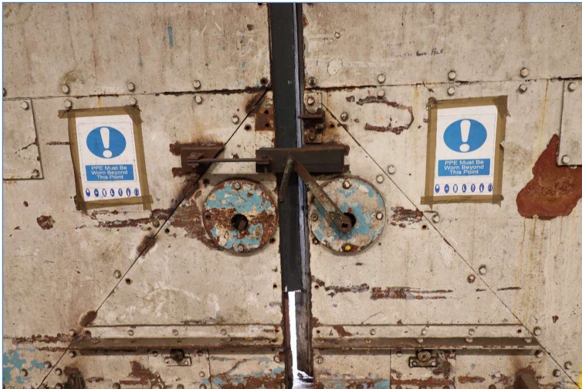
Plate 16 Hangar 19, in January 2026, detail of the original hand-cranked mechanism still used for opening the sliding doors at the southern end of the hangar.
