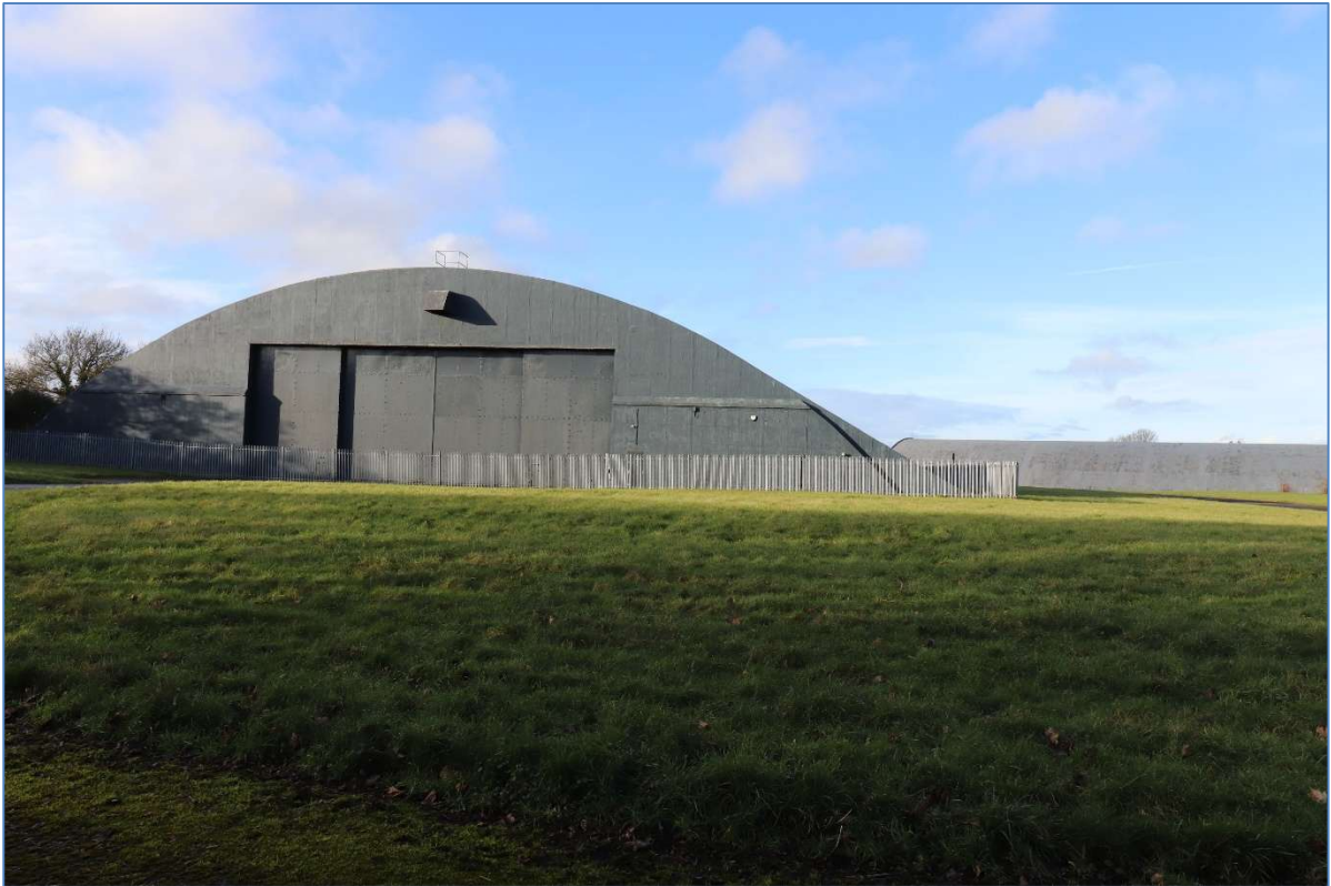
Plate 20 Hangar 20, in January 2026, looking north, showing the retained smaller sliding doors at this end, Hangar 18 in the right background.
