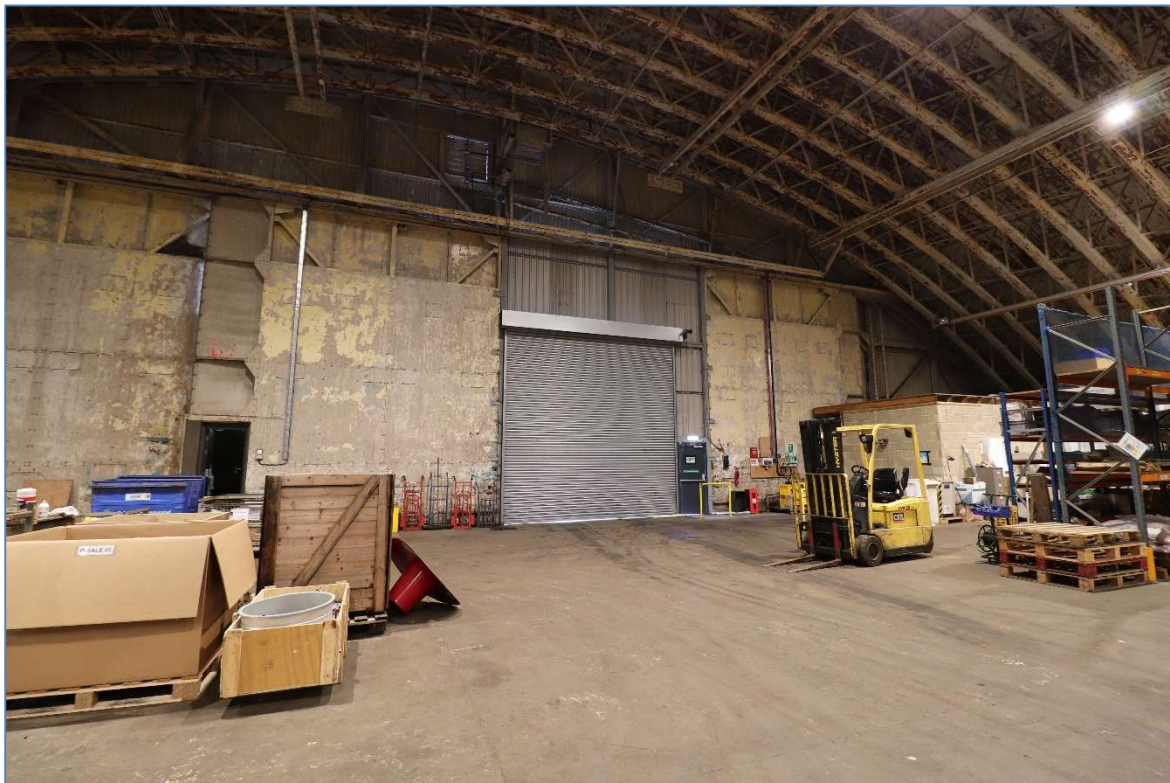
Plate 17 Hangar 19, in January 2026, the insertion of a smaller roller shutter door at the northern end, with the original sliding doors still present but fixed in a part open position. A new blockwork office structure is part-hidden behind the yellow forklift truck on the right.
