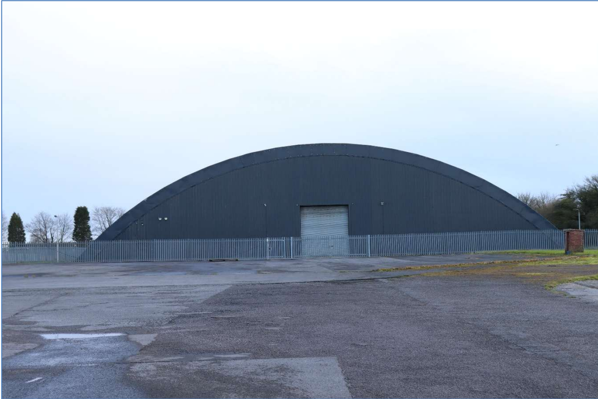
Plate 10 Hangar 20, in January 2026, showing the complete replacement of the concrete northern wall in metal, resulting in the loss of the distinctive large sliding doors, shallow crew office and boiler room annexes and 'ears' added by 1956.
