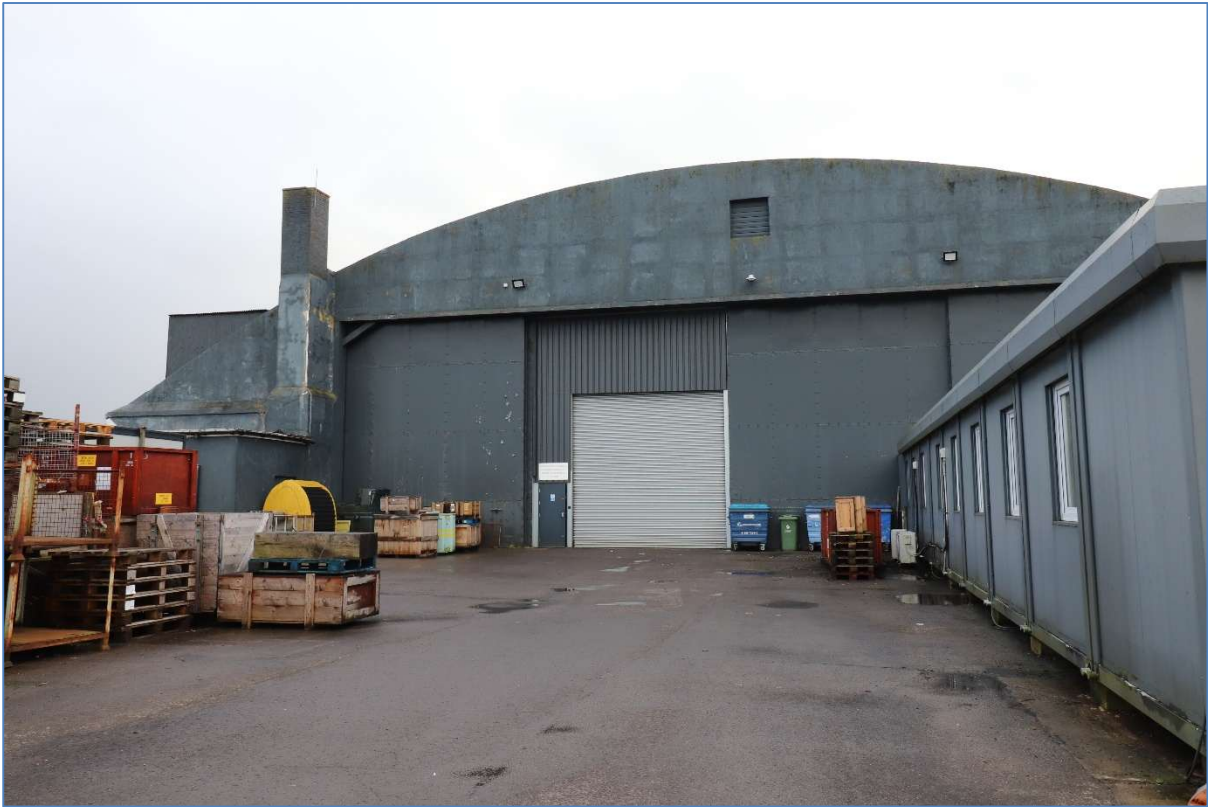
Plate 14 Hangar 19, in January 2026, showing the exterior wall and doors at the northern end.
