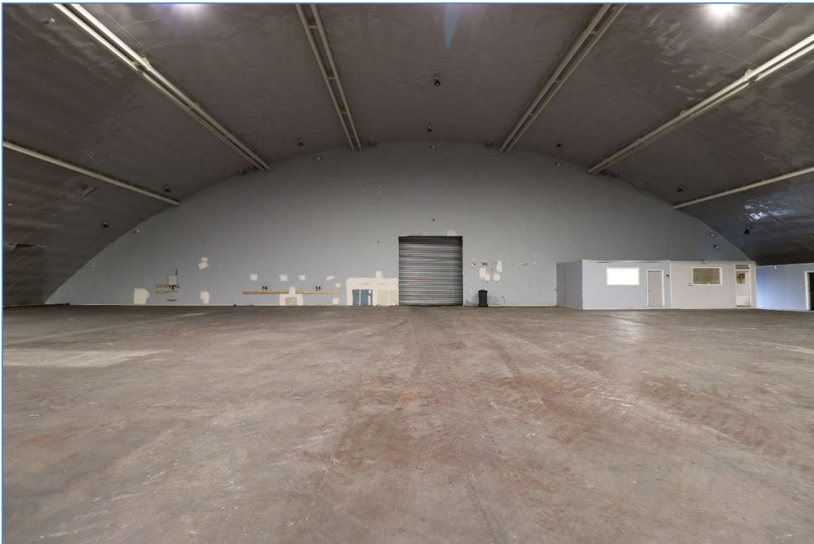
Plate 19 Hangar 20, in January 2026, looking north, showing the inside face of the rebuilt end wall and roller shutter door which replaced the original large sliding doors at this end.
