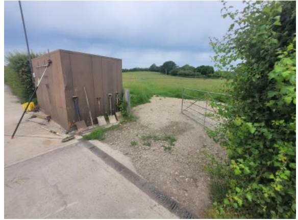
Photo 2: Compacted hardcore serving as site access.
