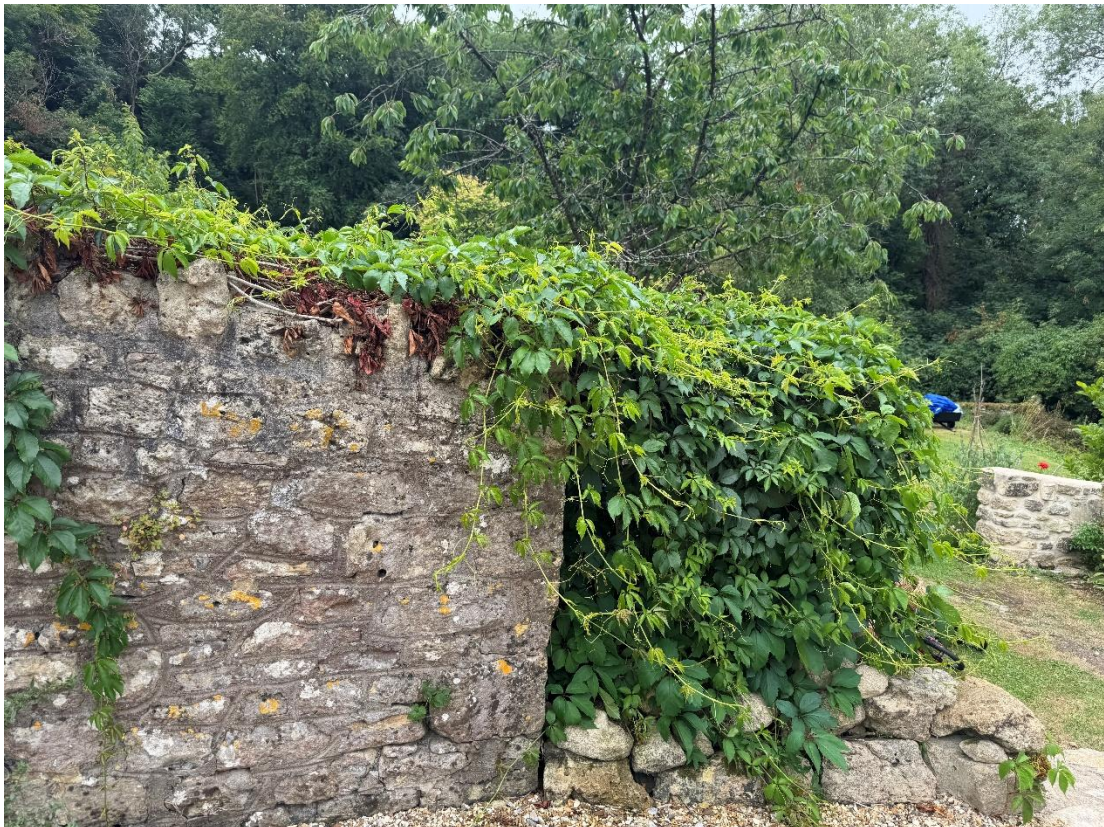
Plate 2: External view of northern elevation of the pigsty
