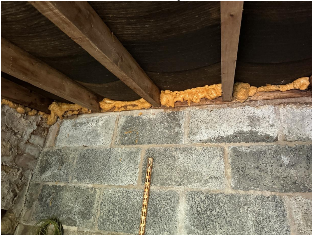
Plate A2: Eastern wall of pigsty – existing roost
