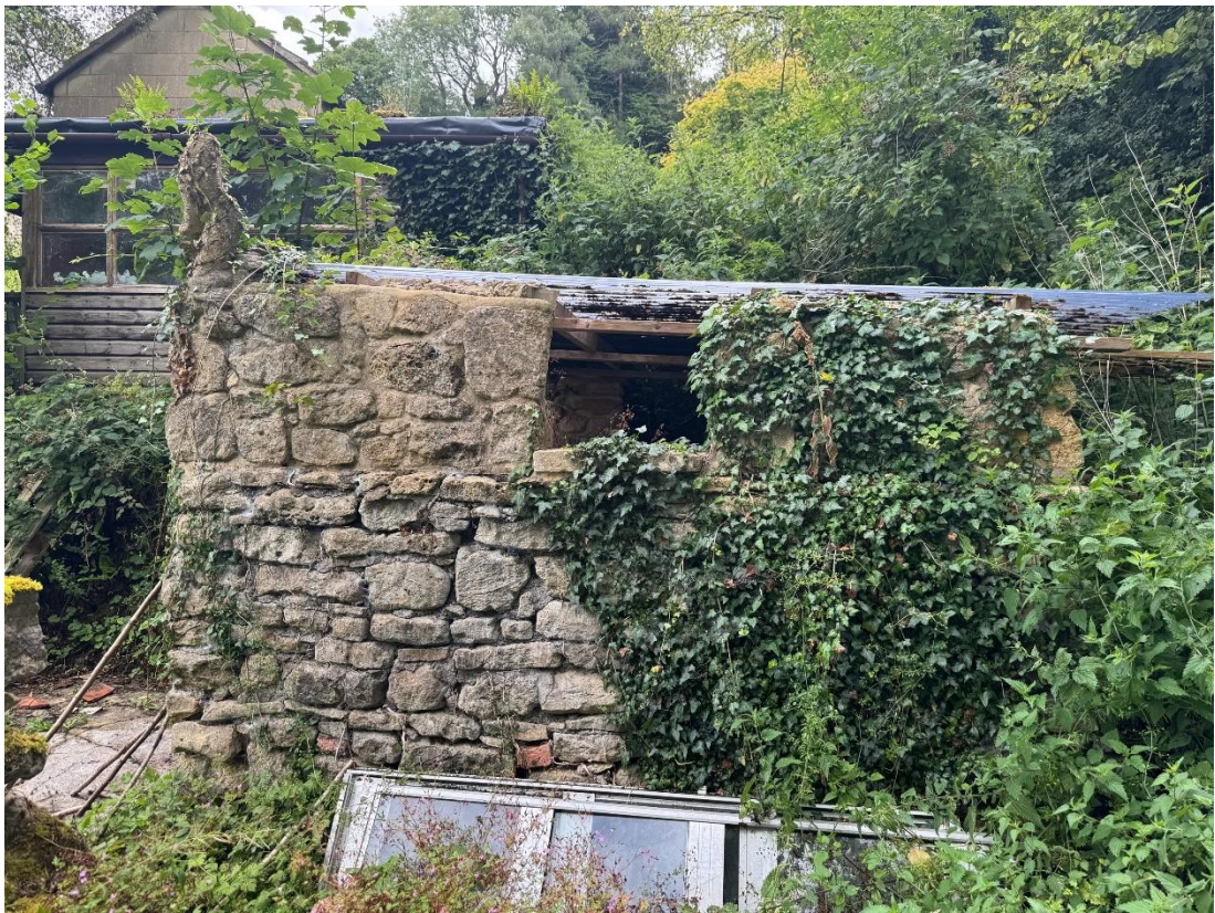
Plate 6: Showing replacement roost and proposed new entrance
