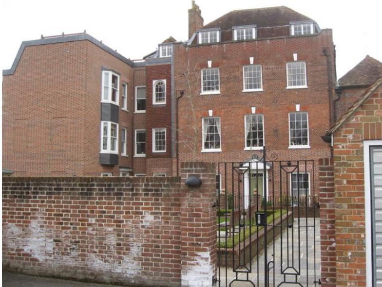
Rear elevation – 52 nearly completely obscured, 54 carefully restored (officer's photo 2013)
