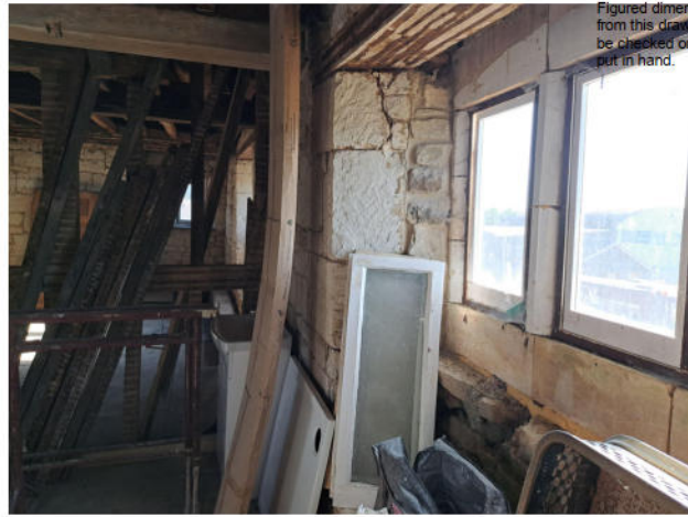
P Window WF05 and exposed wall studs
