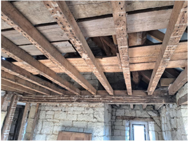
I Exposed ceiling beams
