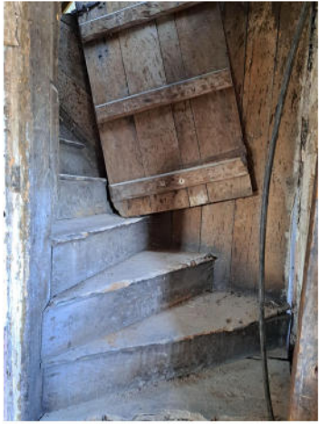
D Stairs up to main loft
