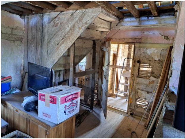
C Door DF01 and underside of stairs
