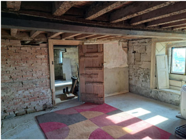
O Sitting room north east corner
