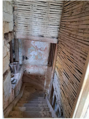
G Stairs down to kitchen
