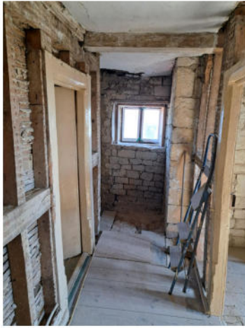
E First floor corridor looking north; Window WF02
