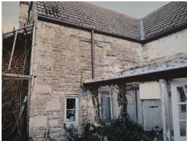
C Previous Conservatory Joining Cross Wing
