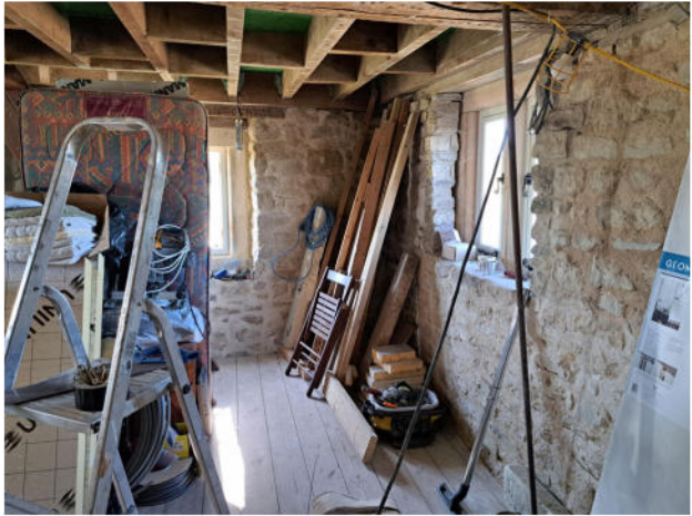
Q Back room with windows WF07 & WF08
