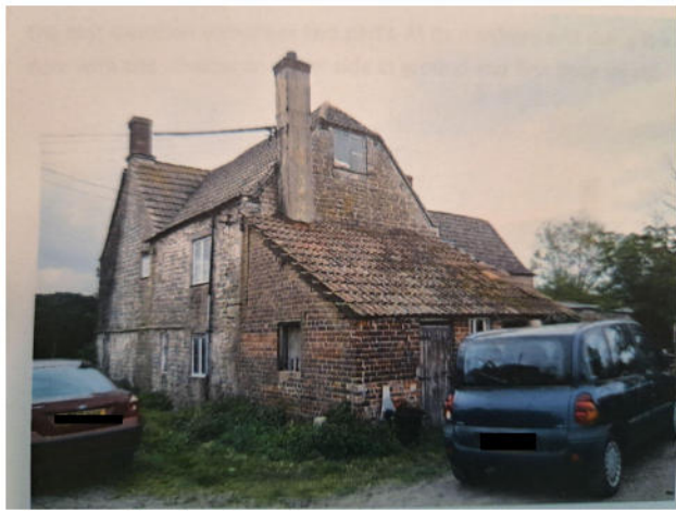
A Previous Lean-to
