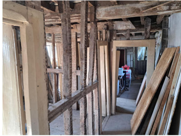
F First floor corridor looking south
