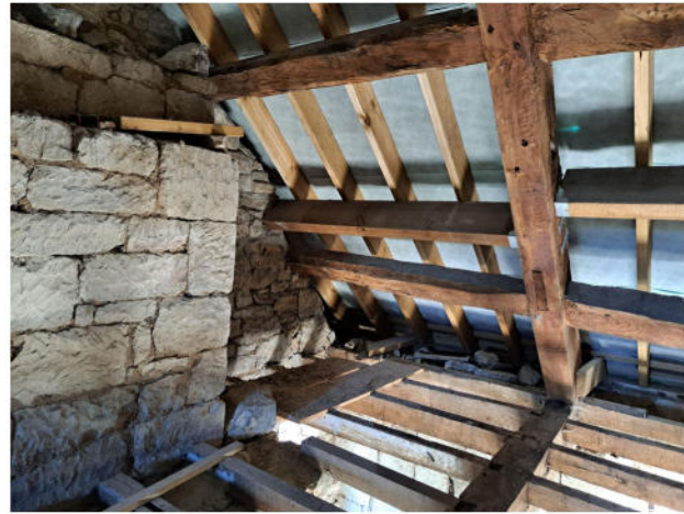
E Exposed roof structure
