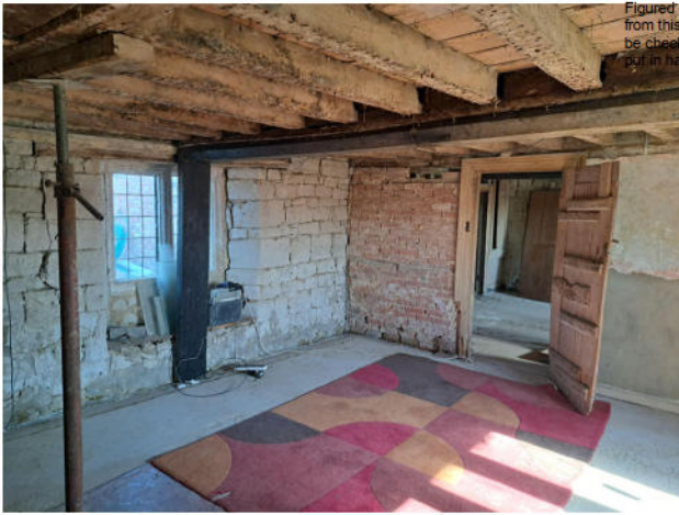
P Sitting room north west corner
