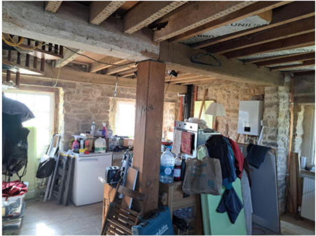
Q Utility room
