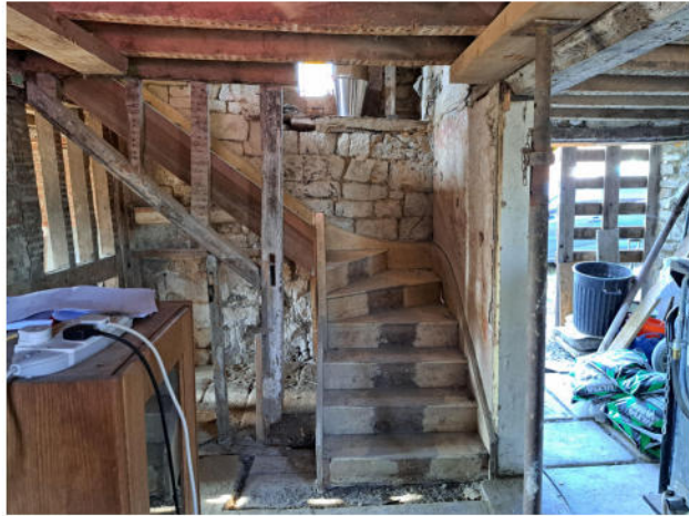
F Stair from kitchen
