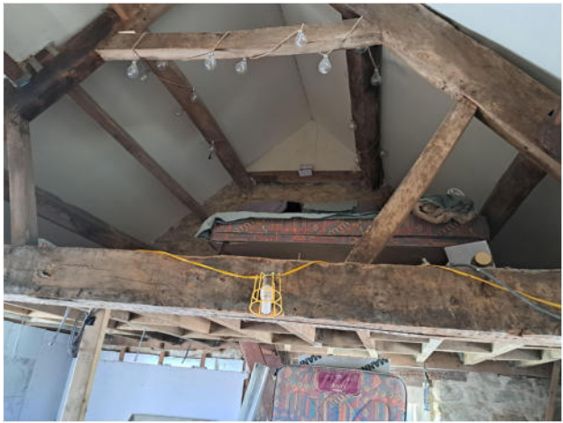
F Loft space above back room
