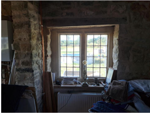
T Utility window - WG07
