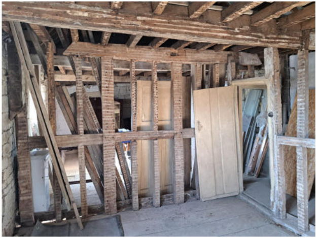
L Exposed wall studs and door DF04
