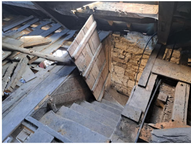
C Stairs Down
