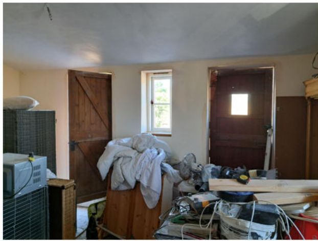
C Doors DG05 & DG06 and window WG12
