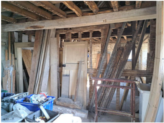
O Exposed wall studs between front and centre bedrooms
