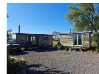
Pair of Shepherds huts (2) at south end of site, with Field Shelter (3) behind
