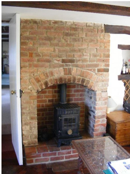
Fig 1 – RM2 Dining Room – view before showing brick fireplace with brick hearth and plastic beams on ceiling
