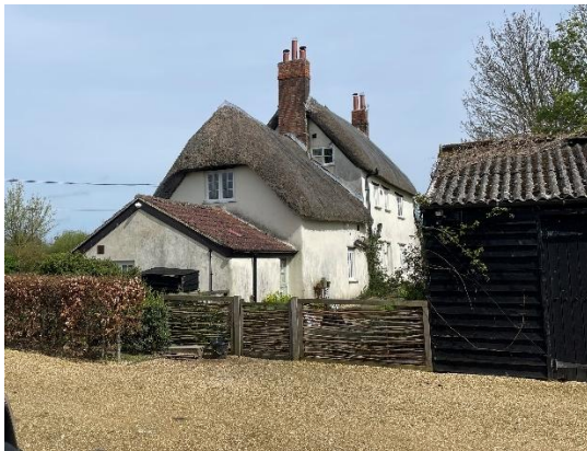
Fig 3 – View from southwest showing kitchen attached to thatched cottage, and outbuilding to the south. Timber gate and fencing separates driveway from rear garden at present.
