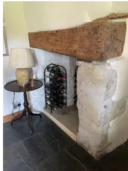
Fig 6 – RM3 Hall – view after alterations exposing original timber lintel, fireplace opened up, plaster removed at low level, stone exposed, new stone hearth and new blue lias stone flooring.
