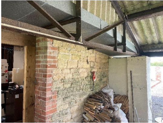
Fig 13 – Roof junction between south end of garage outbuilding and storage barn.
