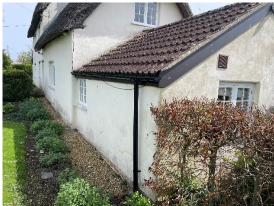
Fig 1 – Kitchen from northwest corner with tiled roof, with north façade of cottage facing the road beyond.
