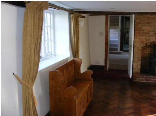
Fig 3 – RM2 dining room – view showing modern plasterboard to ceiling before removal, wood block floor and painted window sill.
