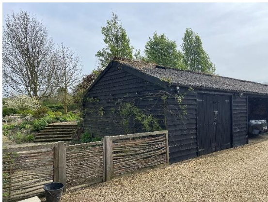
Fig 7 – View of outbuilding workshop and garage with blackened timber cladding and corrugated roof covering.
