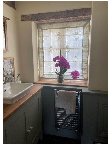
Fig 8 – RM4 WC – view after renewal of WC fittings, new dado panelling, new oak window board and original lintel exposed
