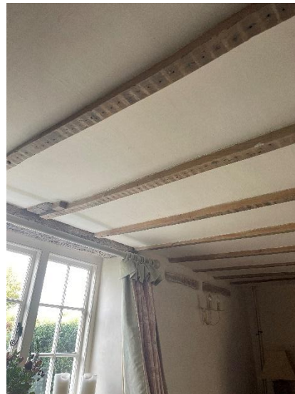
Fig 4 – RM2 dining room -view after plasterboard removed to leave joists exposed
