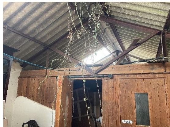
Fig 16 – View of storage barn interior with metal roof truss, corrugated roof covering, and timber sauna and shower rooms visible below.
