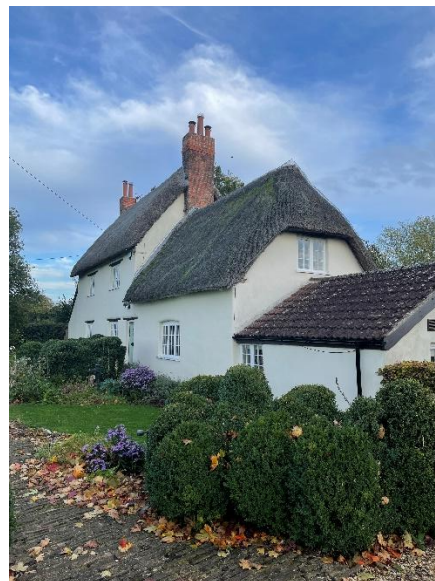
Fig 24 – Exterior from north west showing ventilator terminal in gable wall of kitchen extension, and raised chimneys
