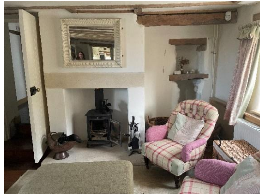
Fig 2 – RM2 dining room – view after new stone lintel and hearth fitted to fireplace finished and finished with lime plaster
