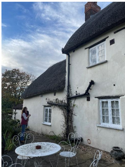
Fig 23 – Exterior from south showing ventilator terminals from bathroom and ensuite
