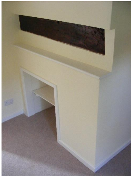
Fig 5 – RM3 Hall – view before alterations showing plastered fireplace alcove, boarding and trim and carpet floor finish
