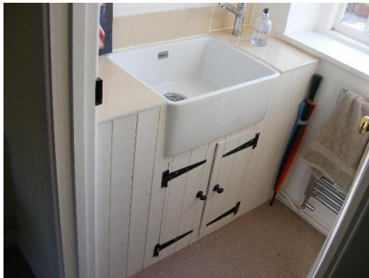
Fig 7 – RM4 WC – view before renewal of basin and replacement floor finish.
