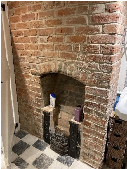
Fig 21 – R11 Ensuite – brick fireplace revealed and repointed, and stone tiles visible
