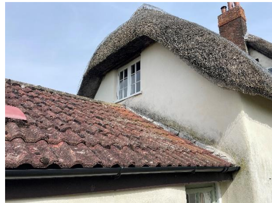
Fig 2 – Kitchen roof to south with entrance door visible, and first floor windows of cottage in west gable wall under the thatch.
