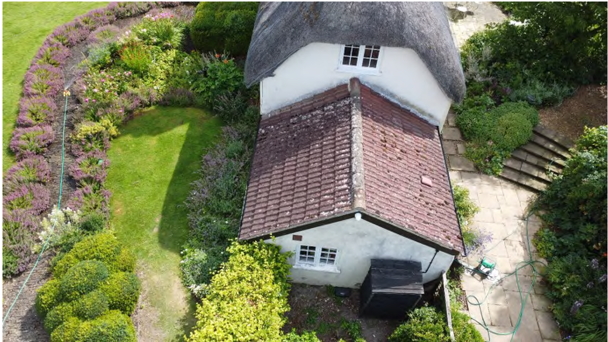
Plate 3 showing kitchen roof with negligible potential for roosting bats and birds
