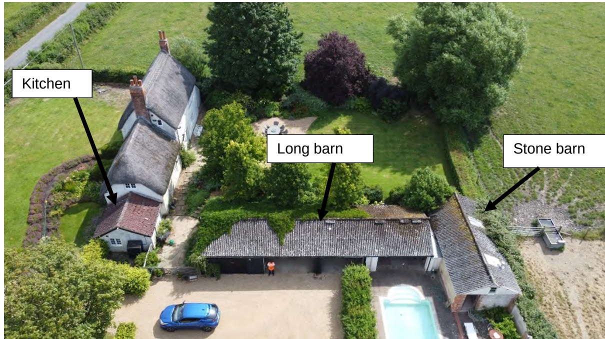
Plate 1 buildings being surveyed 3 Bears cottage
