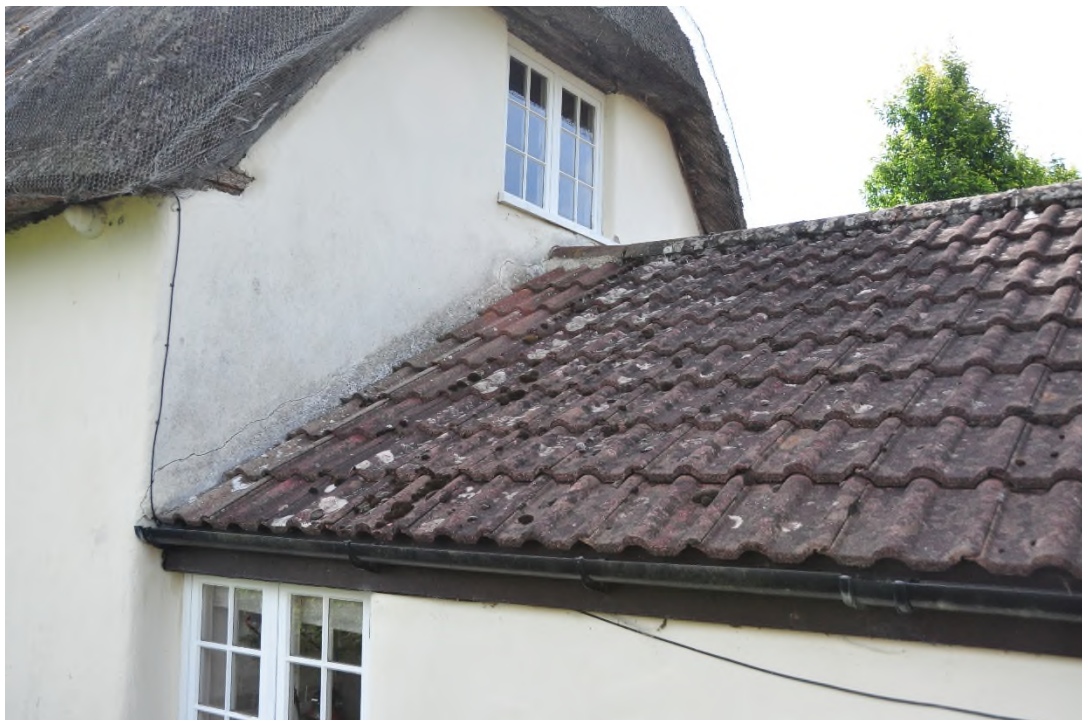
Plate 6 kitchen roof intact and tightly finished
