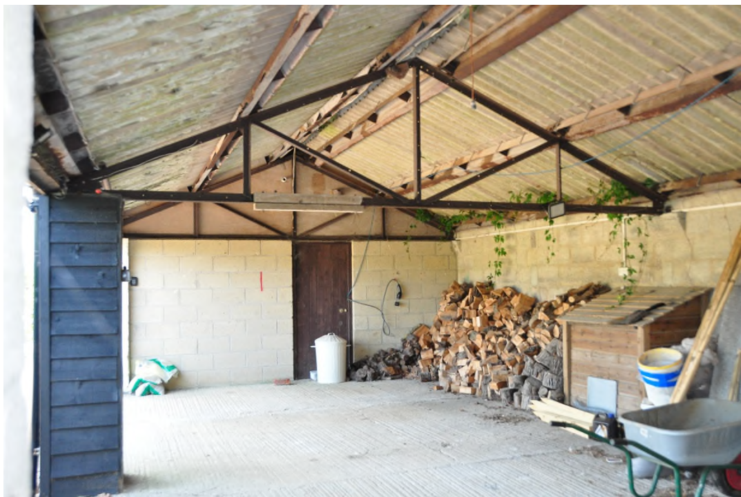
Plate 8 single skin interior roof of the long barn
