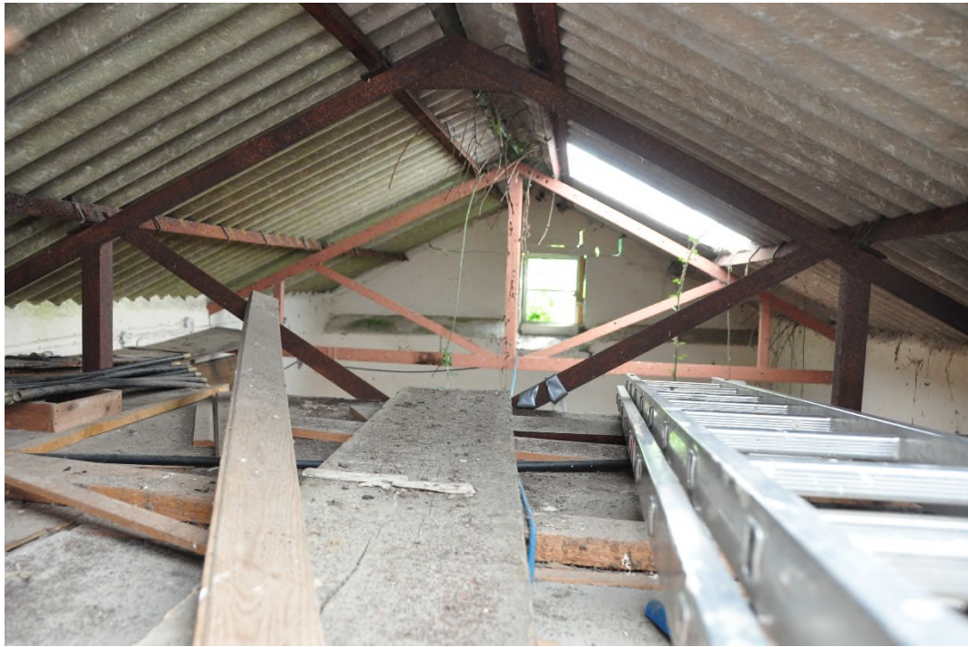
Plate 7 single skin asbestos roof of the stone barn same design as the long barn
