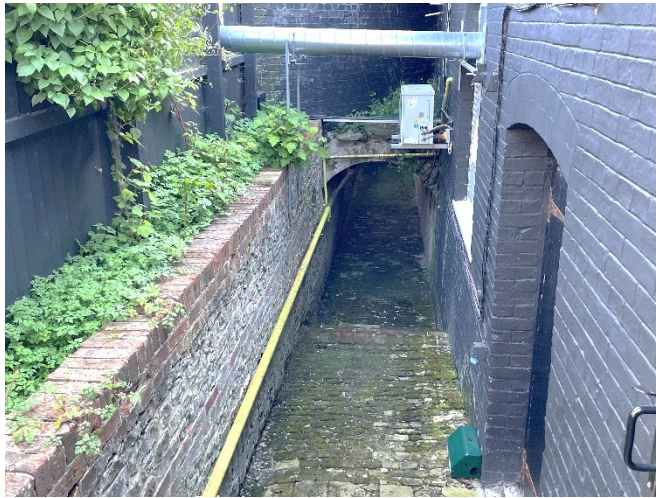
Fig 8: Basement stair: view of basement stair
