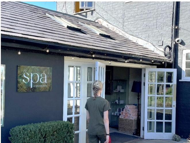
Fig 9: Spa entrance: Two rooflights above spa entrance C20
