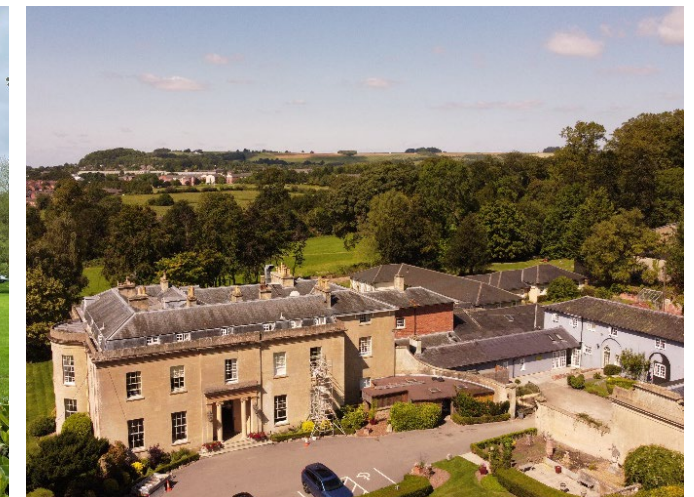
Fig 18: Elevated view of Bishopstrow House
