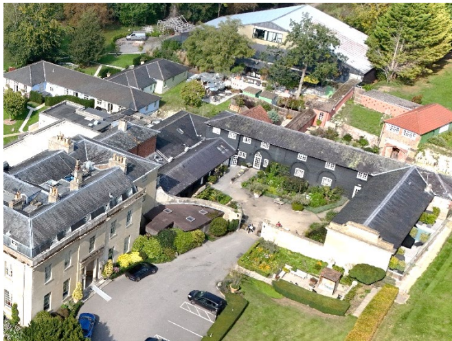
Fig 11: Existing courtyard: aerial view above existing courtyard
