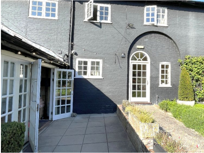
Fig 5: Existing Spa entrance: view to the north corner
