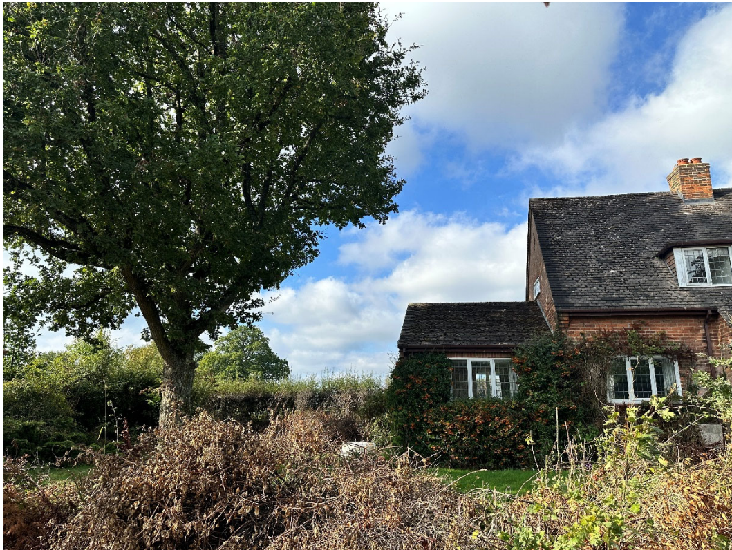
Figure 1: T1 (oak) and existing dwelling.
