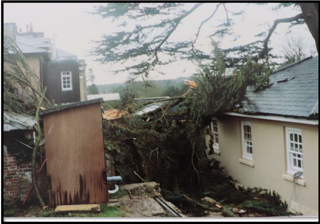
Storm damage to the annexe, late January 1990 (Wiltshire Buildings Record B688)
