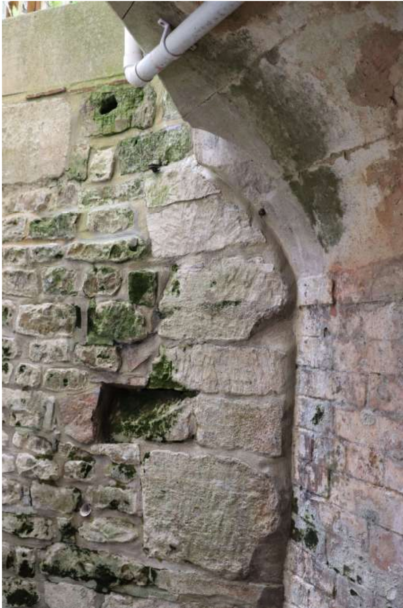
Figure 15 The junction of the Period 1b access area stonework with the bricks of the Period 1a basement
