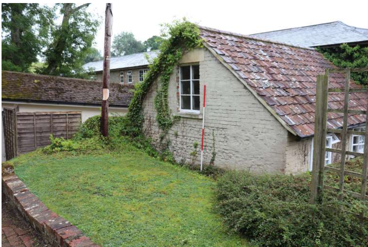
Figure 62 The John Pinch Room looking south-east
