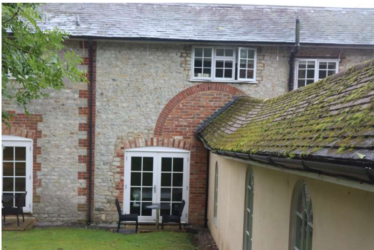
Figure 57 The north side of the arch through the Period 1c block in the stable range, blocked and abutted by post-1976 works, Period 1b carriage house to left
