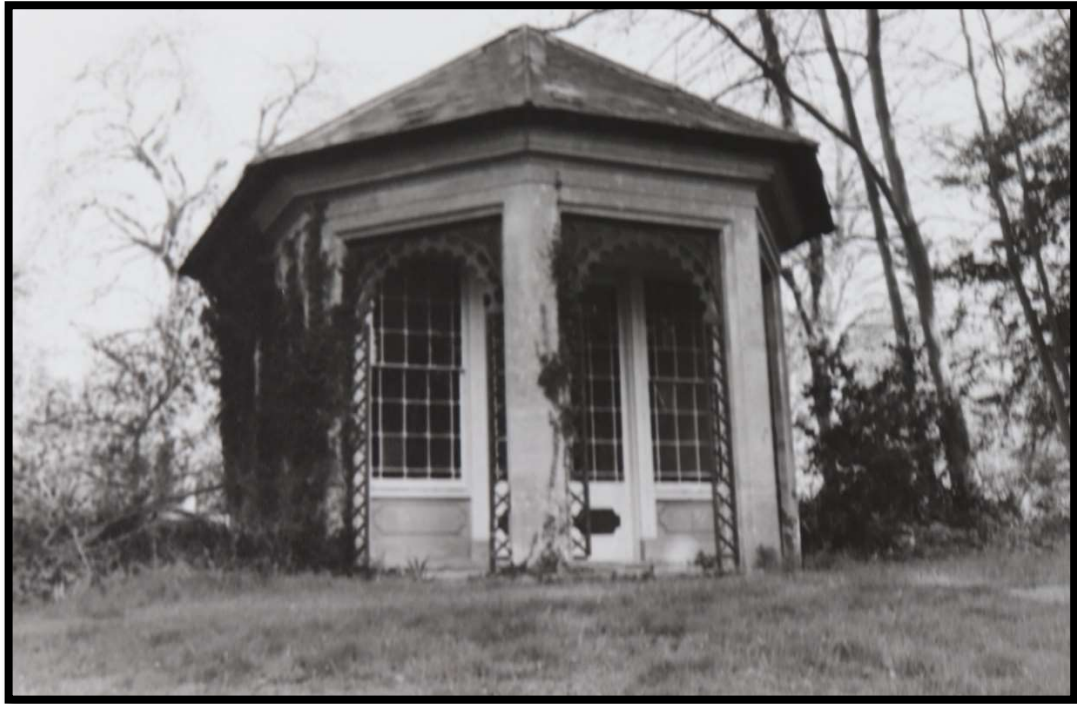
The summer house in 1987 with its fretwork and windows still intact (Wiltshire Buildings Record B688 pt4)
