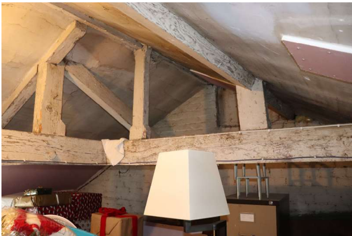
Figure 44 The roof structure in the space over the Oval Room
