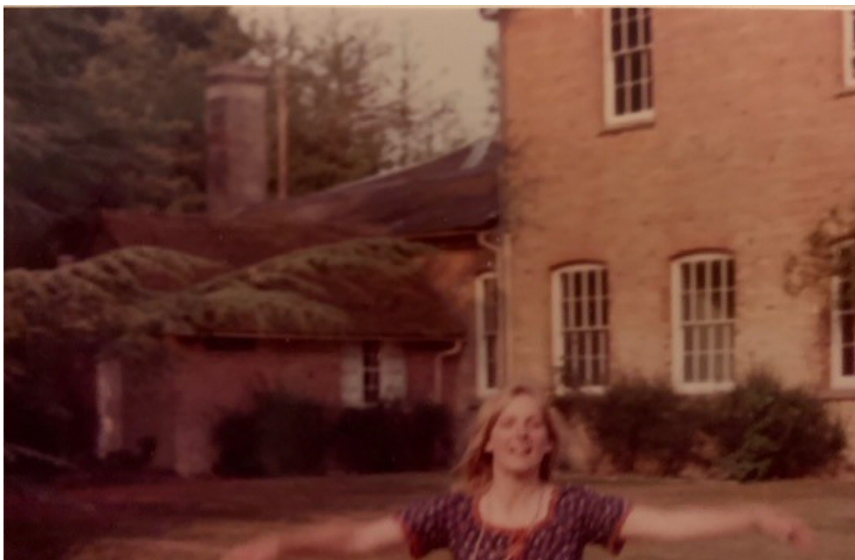
Figure 18 The west elevation of the Period 1c section after the ground floor windows had been altered. Courtesy of Ms Diana Berry
