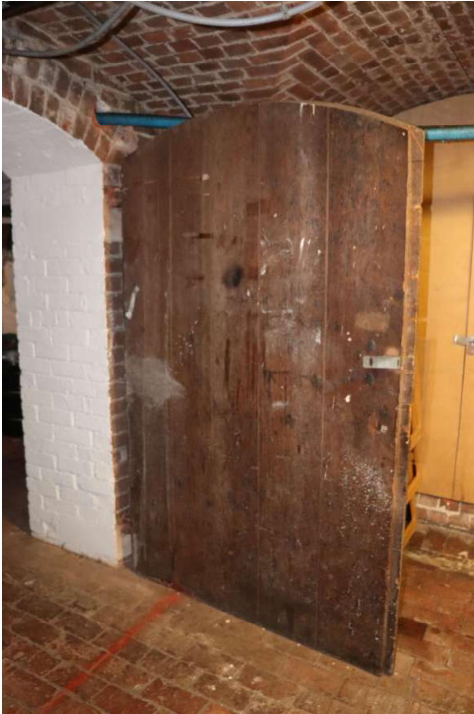
Figure 52 An original door in the basement between Rooms B6 and B9
