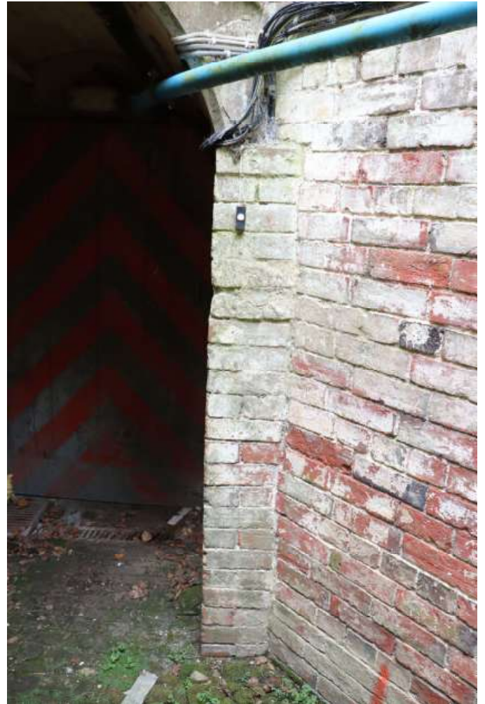
Figure 14 The junction of the bricks of the period 1a and 1b sections at basement level
