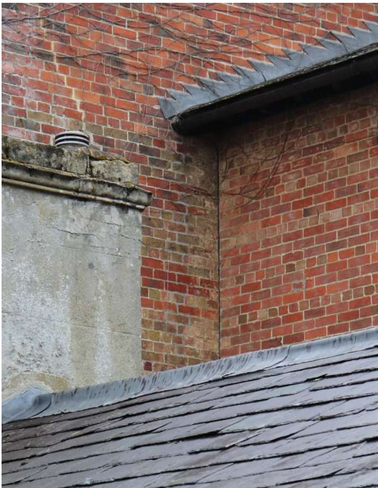
Figure 21 The brickwork of the Period 1c wing (on right) abutting that of the Period 1b block (on left) .
