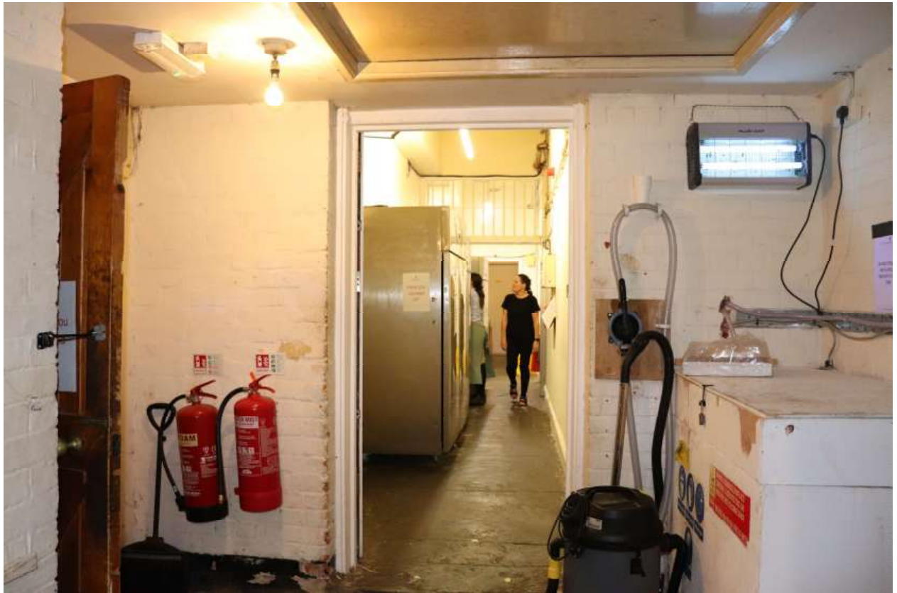
Figure 20 The external door to the central corridor in the Period 1b block, looking south from the later corridor in the Period 1c addition
