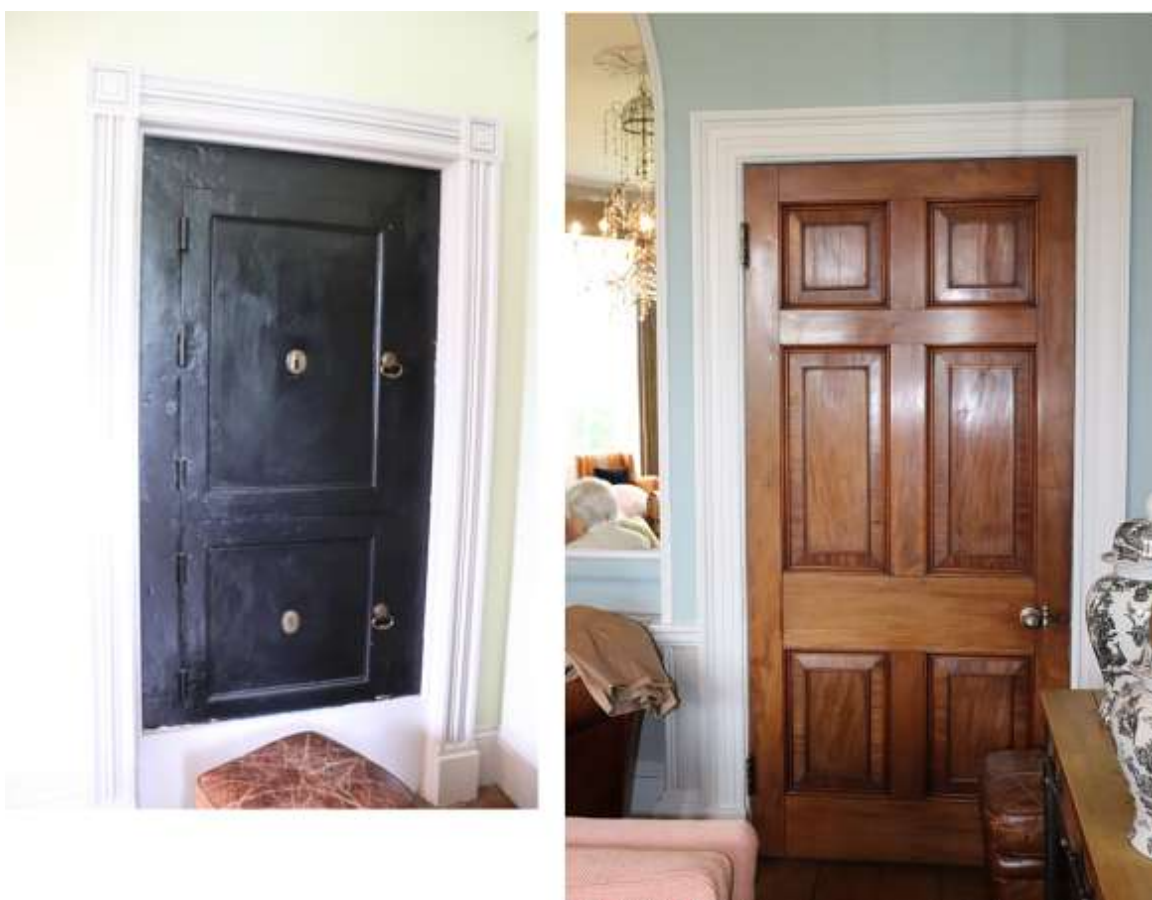
Figure 31 The safes in the Library and the cupboard in the Lounge, occupying former doorways
