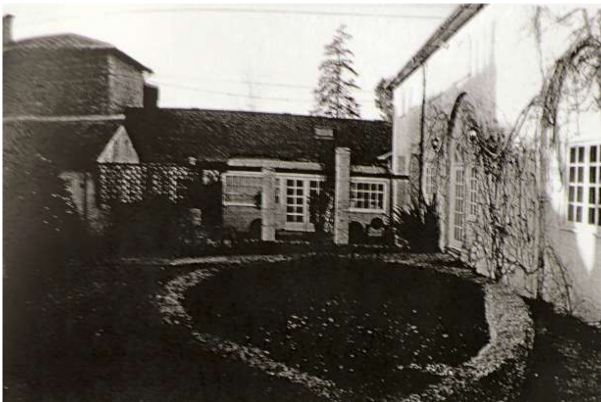
Figure 51 Photograph from 2007 showing the north end of the Period 1d single-storey range on the west side of the stable courtyard removed
