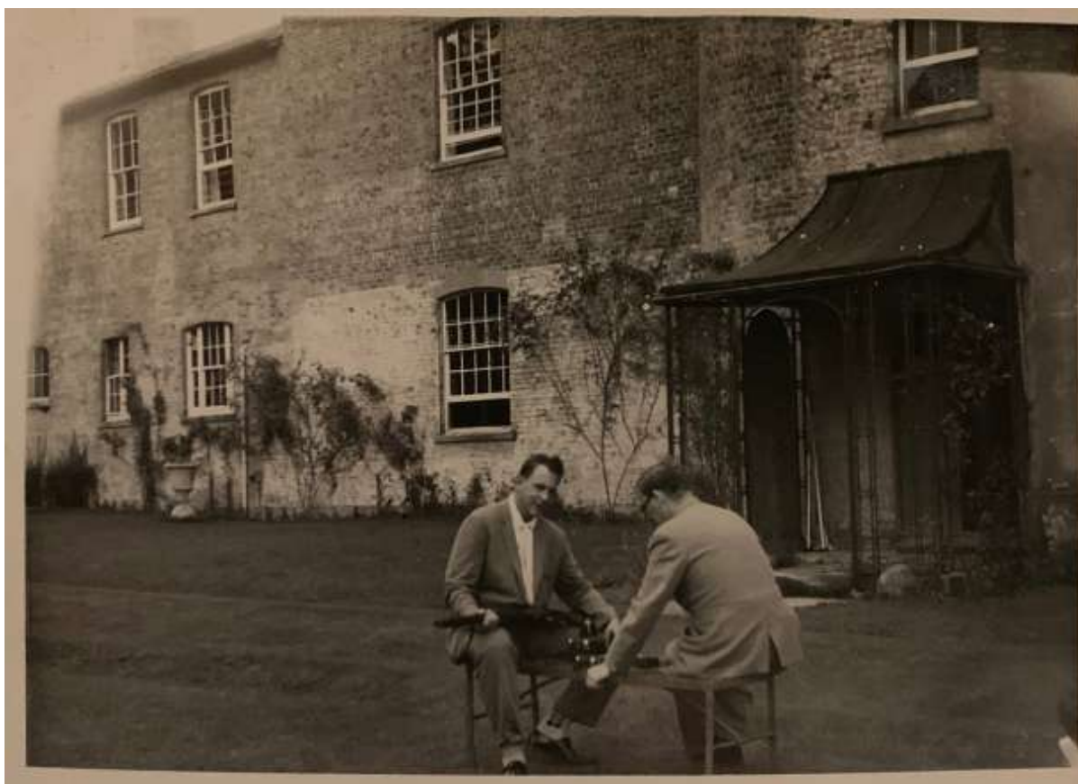
Figure 17 The west elevation of the Period 1b and 1c additions, c. 1965, before the alterations to the ground floor windows in the two-storey section, courtesy of Ms Diana Berry
