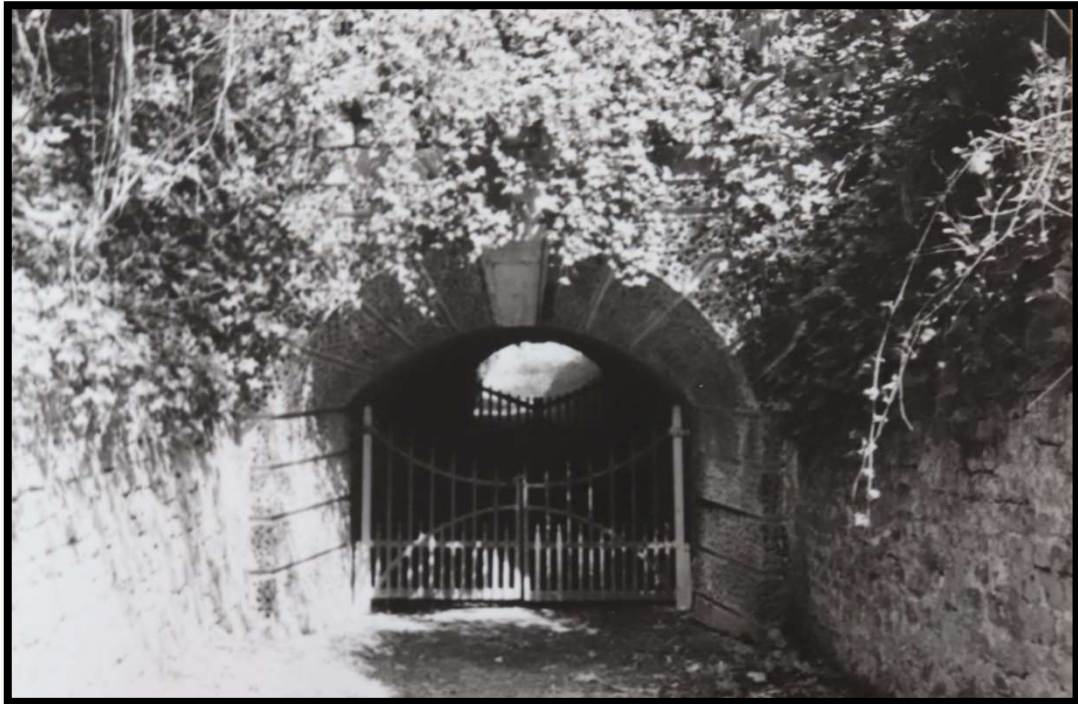
The tunnel with a set of gates still intact, date unknown but possibly 1987 (Wiltshire Buildings Record B688.1)
