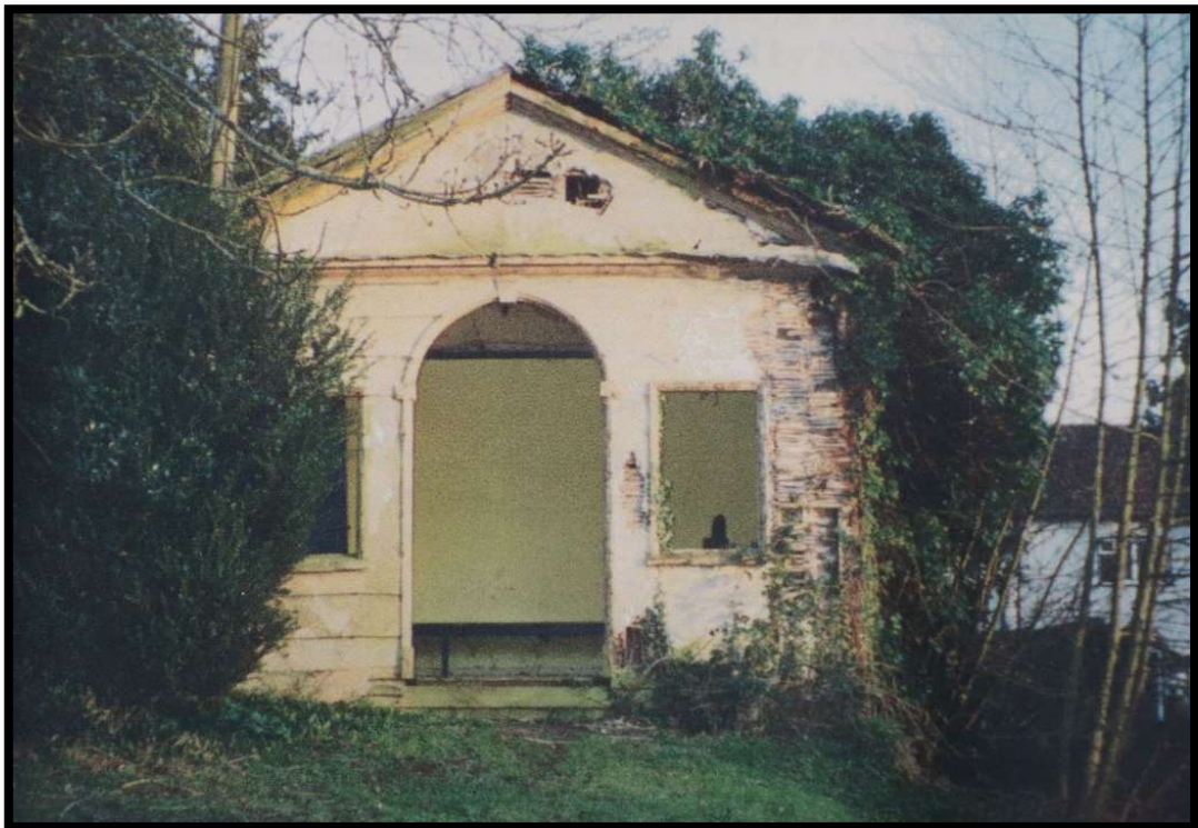
The garden shelter/pump house in or before 2002 (Wiltshire Gardens Trust)
