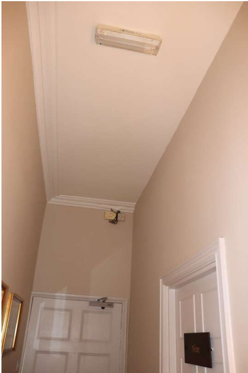
Figure 50 The corridor in the first floor of the period 1c range, cornice showing it formerly part of Room 9 to the right
