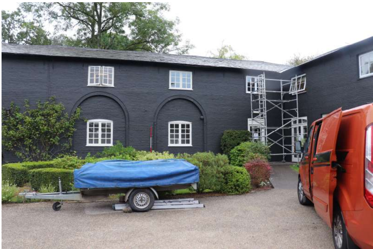
Figure 55 The south side of the Period 1b carriage house
