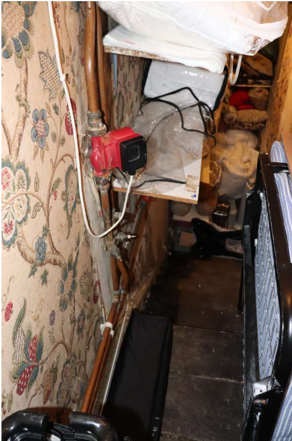
Figure 45 The upper flight of the former service stair to the first floor, looking west, now a lumber room
