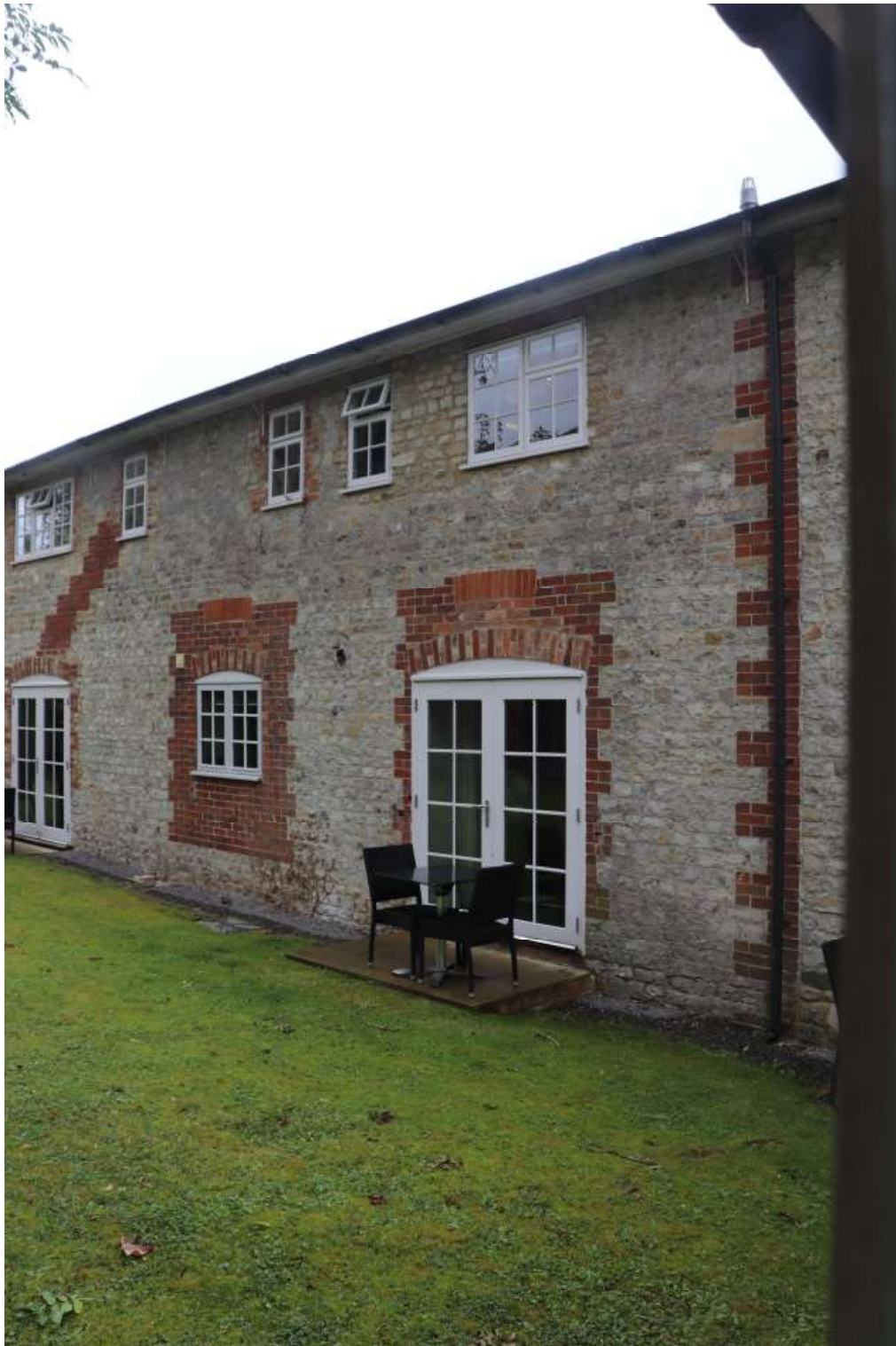
Figure 54 The north side of the Period 1b stable block showing the brick quoining and the remains of the original windows
