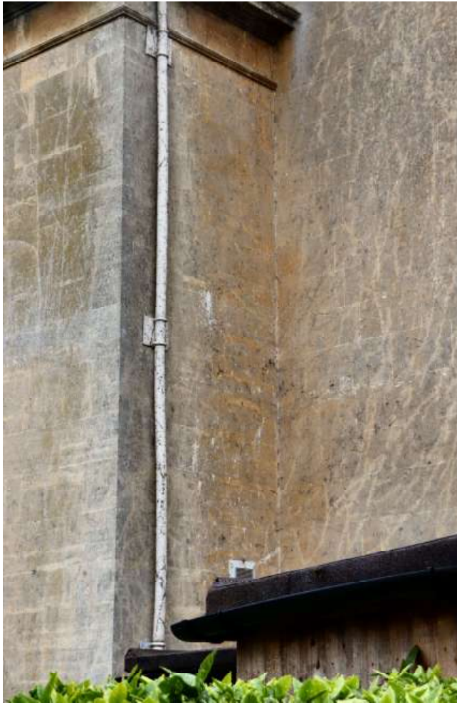
Figure 13 The junction of the Period 1a and 1b blocks on the east elevation
