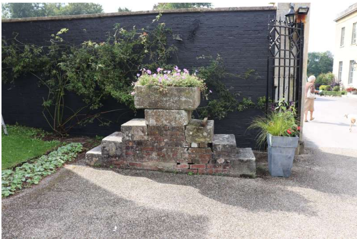
Figure 61 The stone and brick mounting block in the stable courtyard
