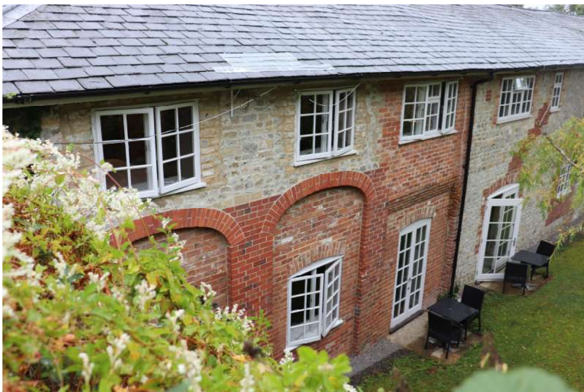
Figure 58 The north side of the Period 1c stable blocks, looking south-west
