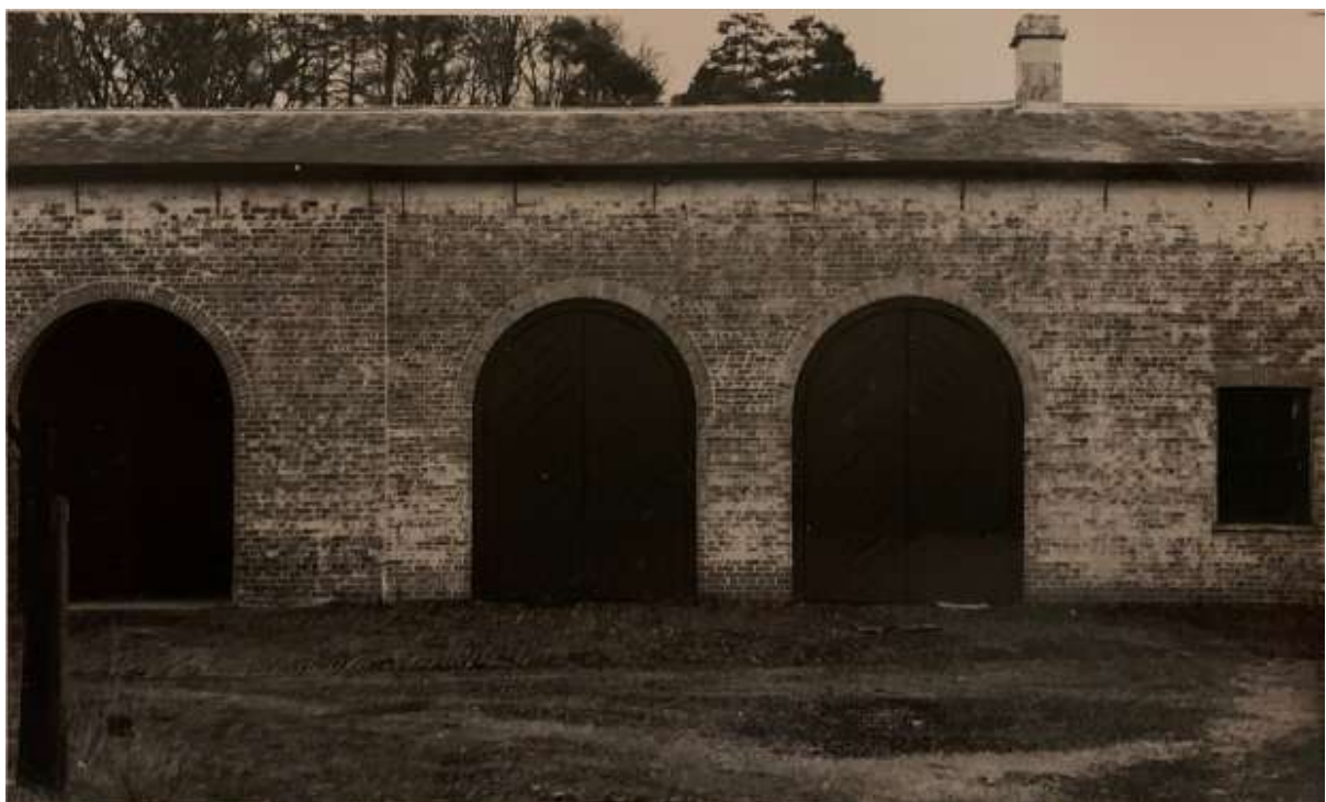
Figure 56 The Period 1b carriage house and Period 1c archway, probably in the 1950s before repainting before 1964. The remnants of probably original whitewash are visible, courtesy Ms Diana Berry
