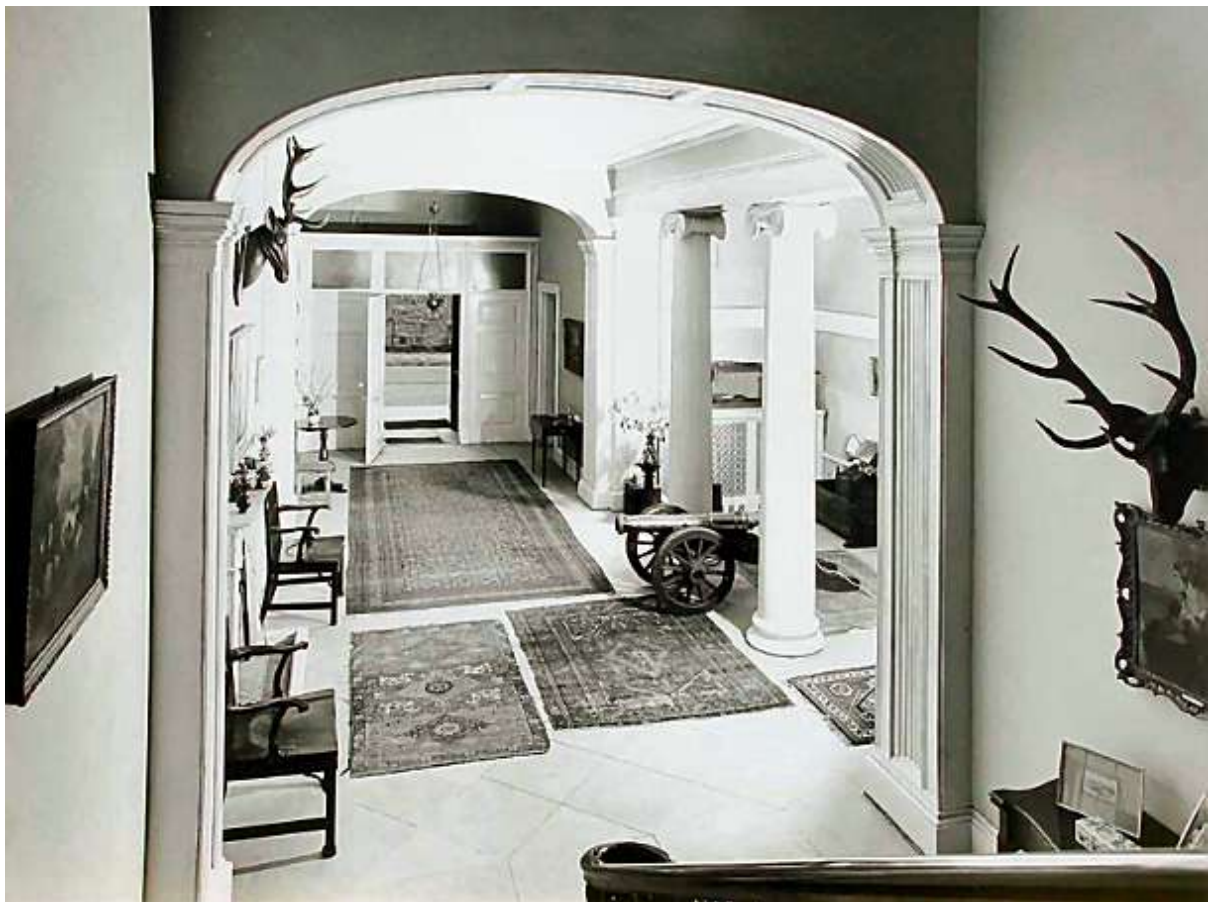
Figure 29 The Inner Hall before the removal of the Ionic columns and repositioning of the screen
