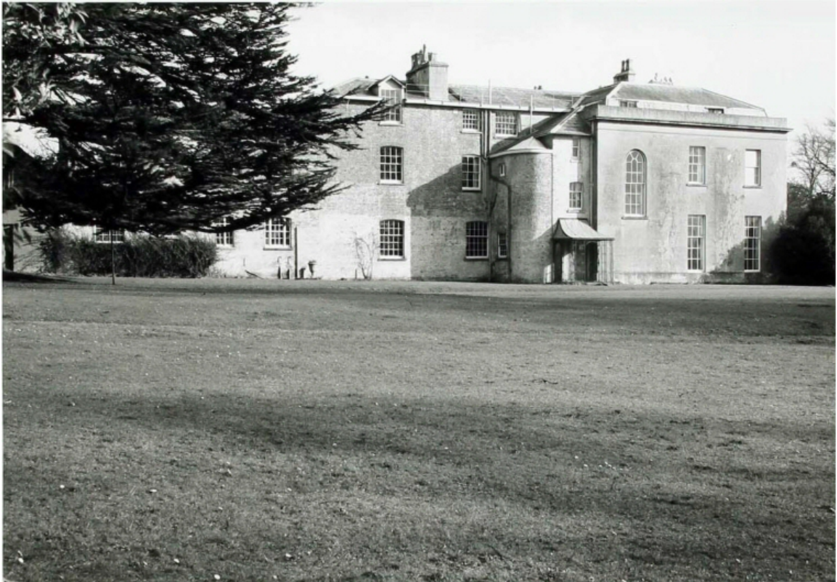
Figure 12 The west elevation of Periods 1a-1c block, c. 1965, before the alterations to the ground floor windows in the Period 1c section (Historic England archive)
