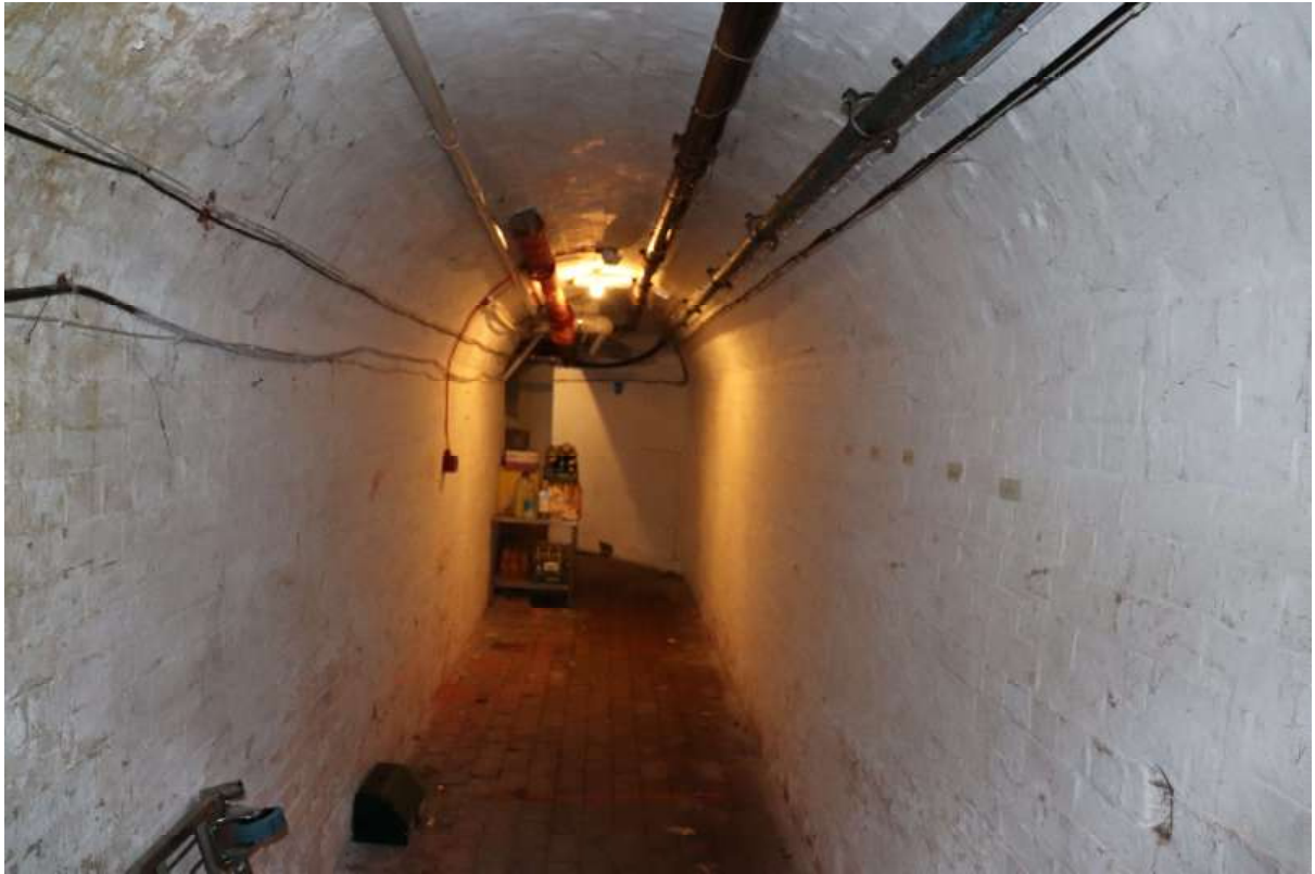
Figure 53 The tunnel in the basement, looking south-west
