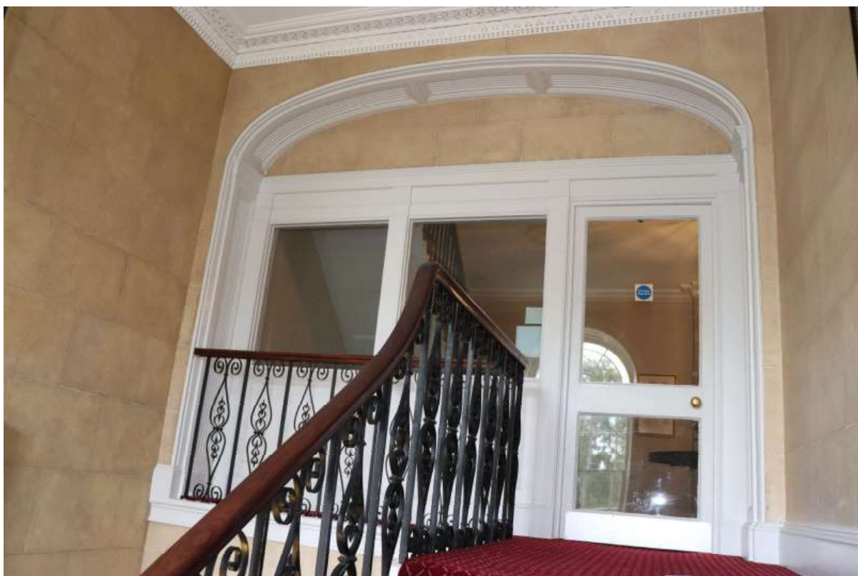
Figure 37 The top of the main stair, showing the cornice and modern wall treatment and the fire stop screen
