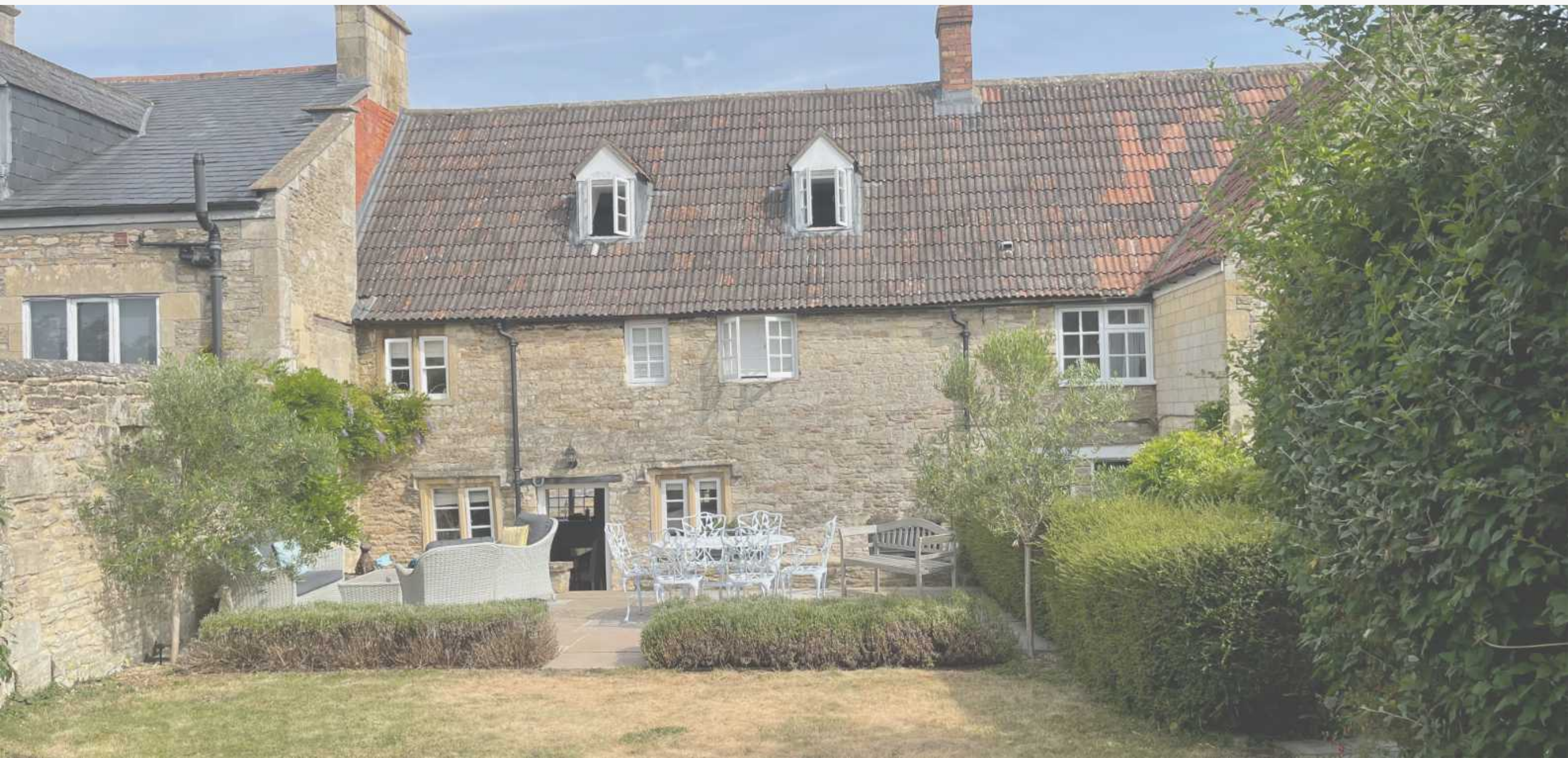
Wickham Cottage, Rear Facade
