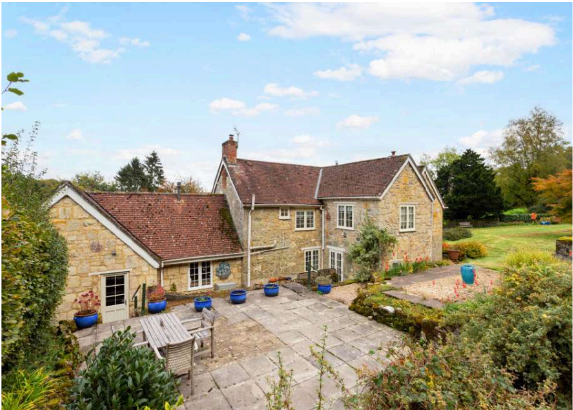
Rear elevation of house
