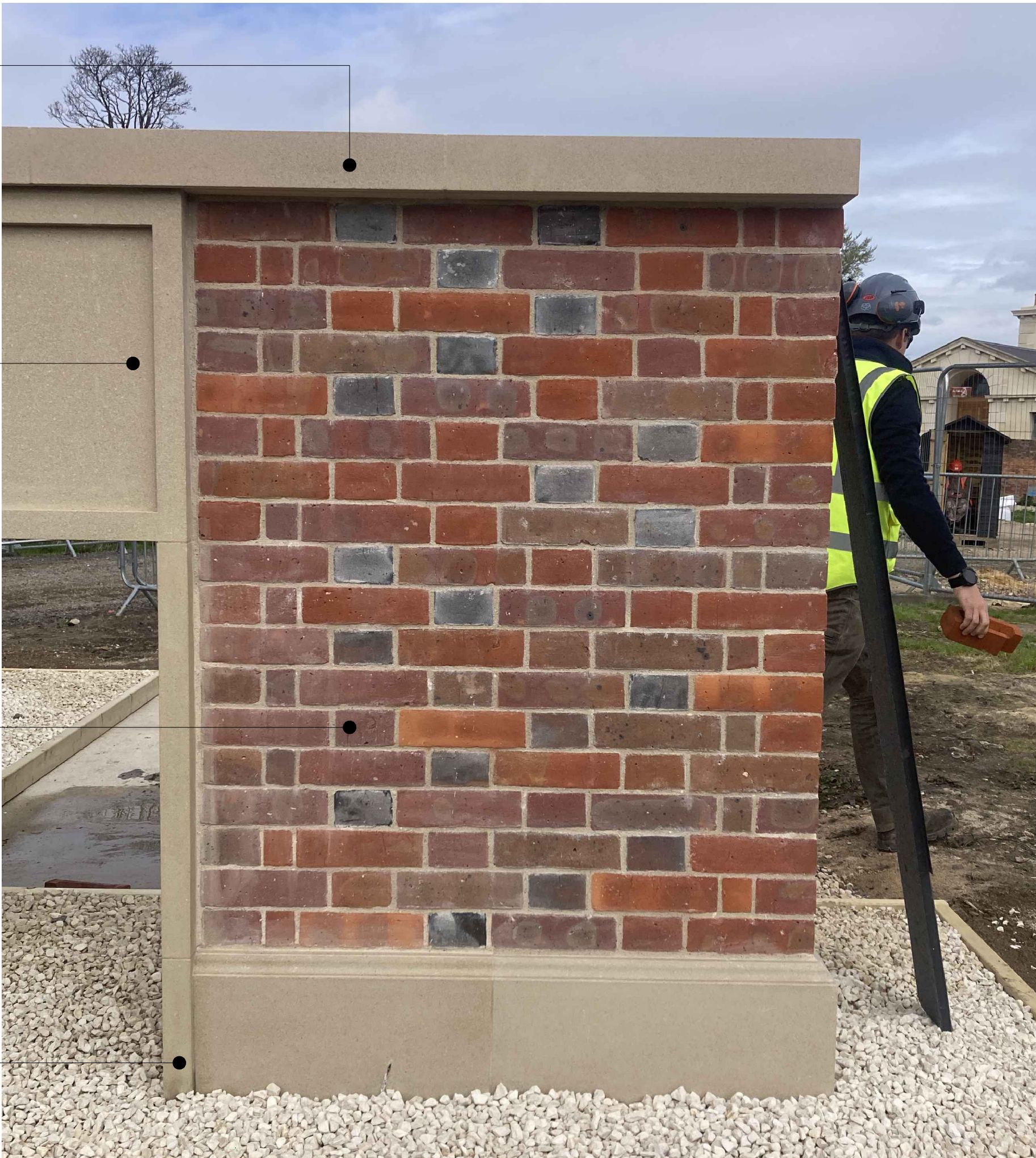
External Mockup Photograph (14/4/26)
