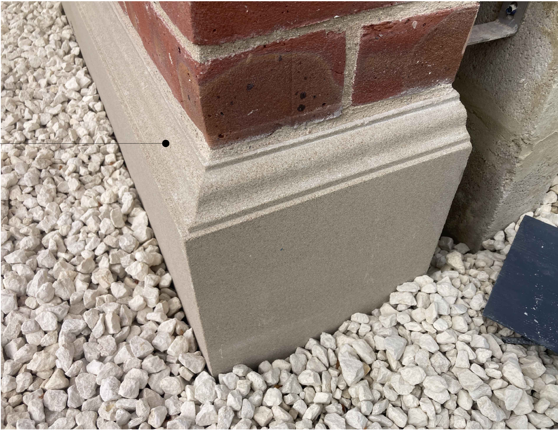
External Mockup Photograph (14/4/26)
