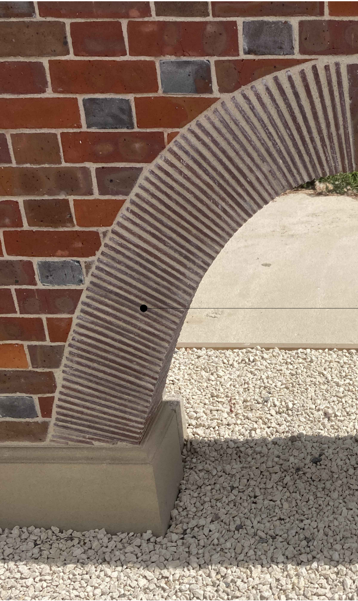
External Mockup Photograph (14/4/26)
