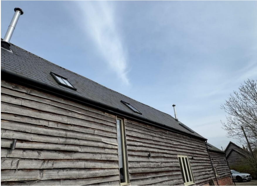
Fig.4 Southwest elevation to barn
