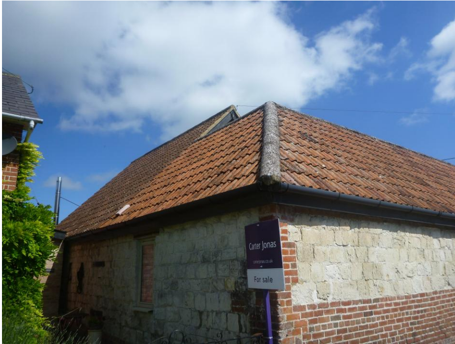
Fig 7: There are no roof lights installed in the south or west faces of the roof of the Little Barn.
