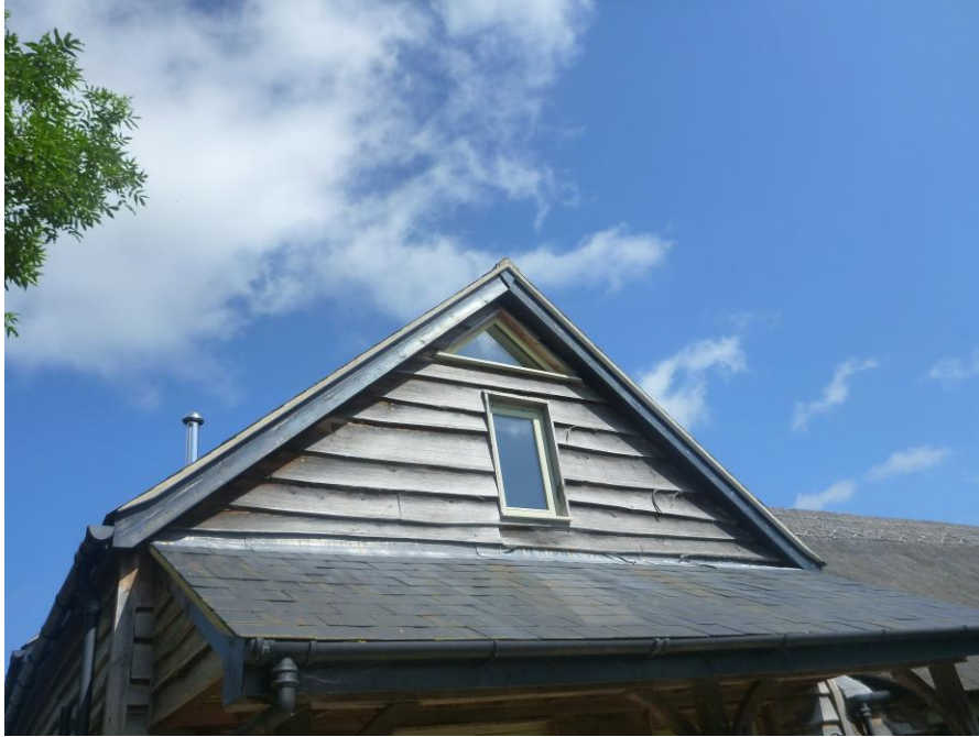
Fig 5: The mortar at the roof verges is in a good state of repair.
