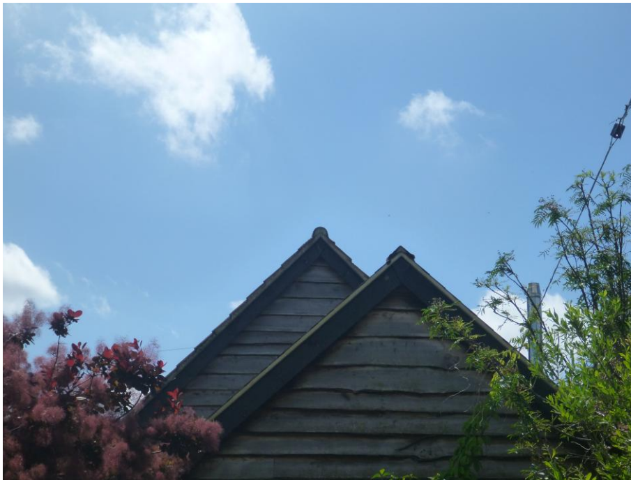
Fig 8: The mortar at the roof verges is in good condition.
