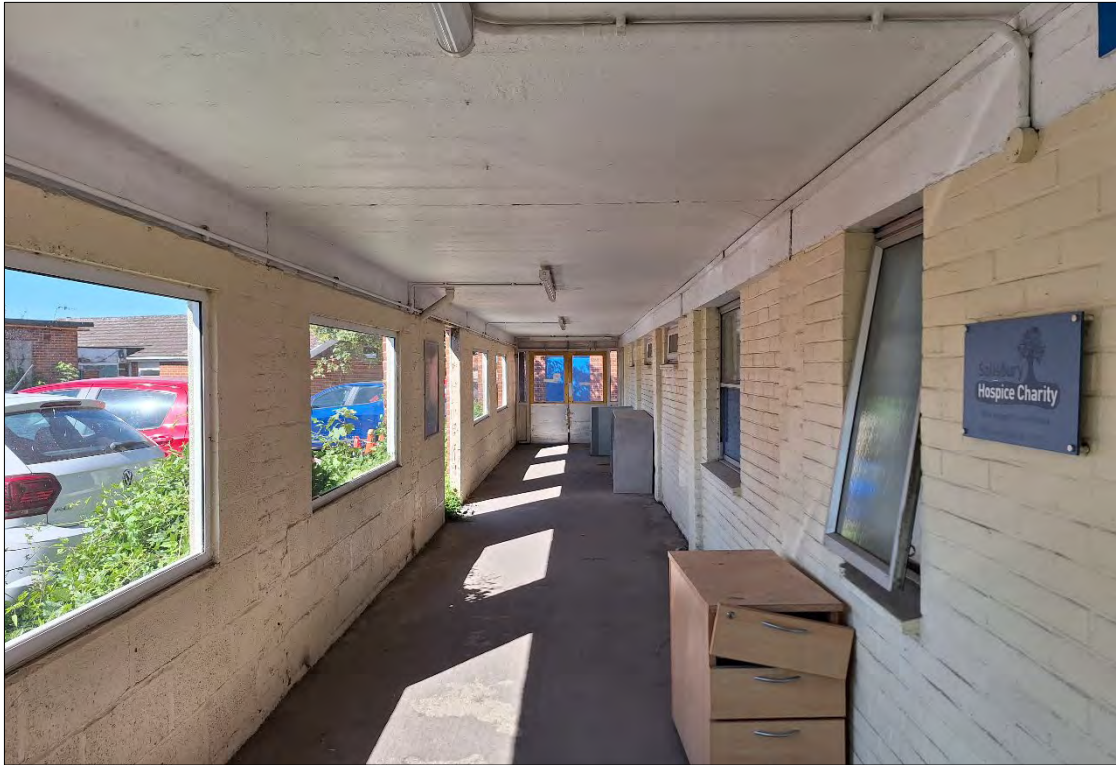
Photo 6: Corridor connecting parts of Building 15, looking west
