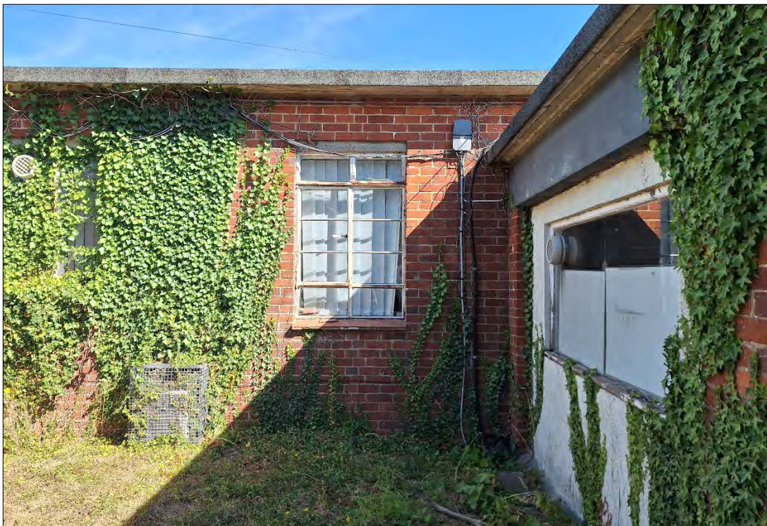
Photo 9: Building 15 rear exterior
