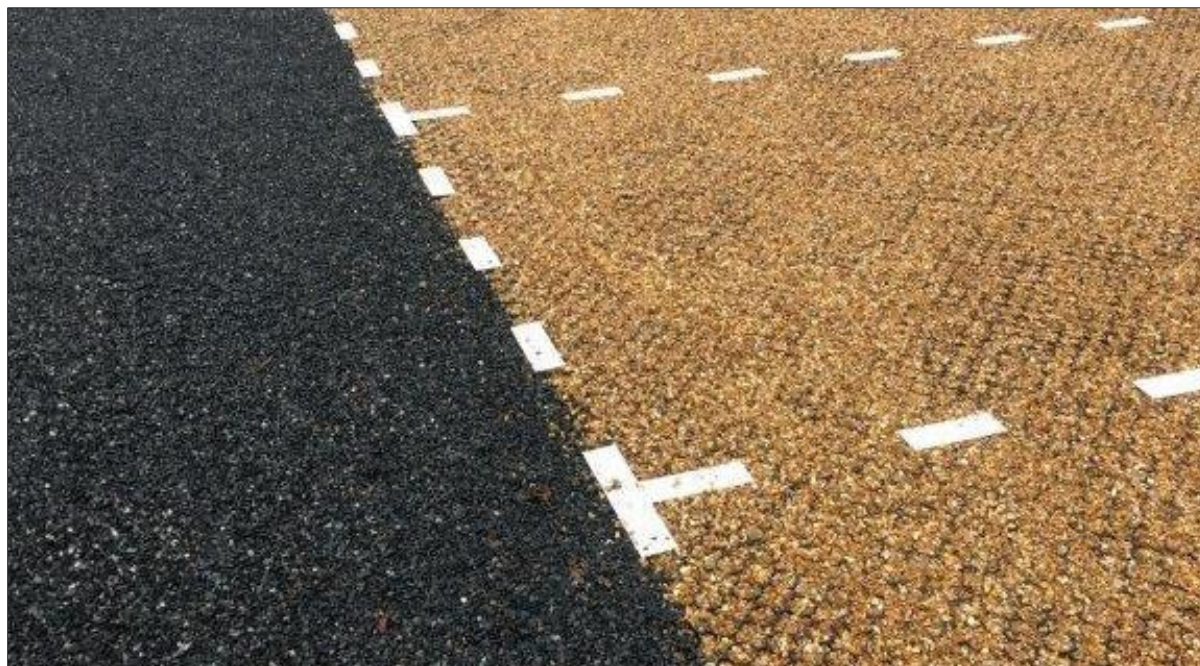
Figure 4.2: Example of Bodpave Car Park
