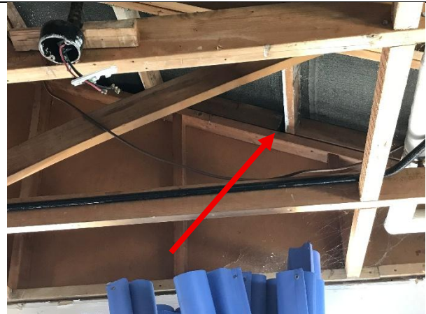
Photograph 14. B16, space behind hanging tiles at gable end with access into building
