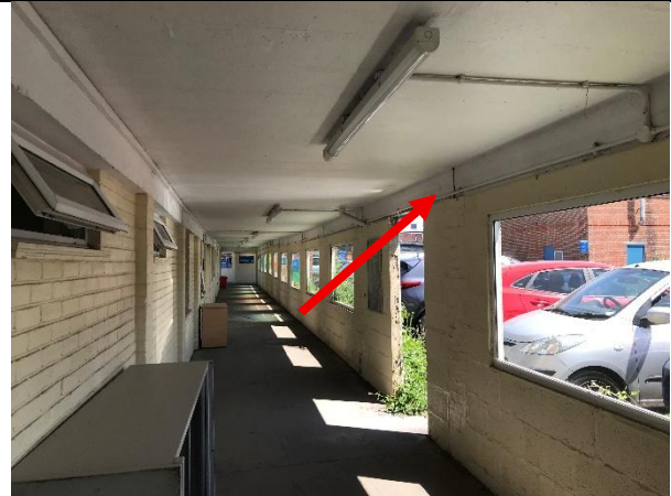
Photograph 8. B15 corridor on south side, open to bats with potential roosting features
