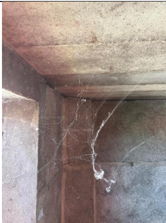
Photograph 9. Inside B15 tower
