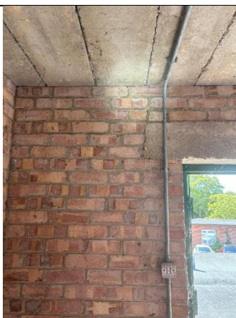
Photograph 17. Inside B17 tower
