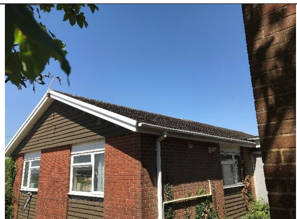
Photograph 12. B16, south gable and east soffit potential roost features with access into building
