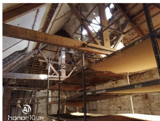
Plate 2. Internal upper floor of Building 1.
