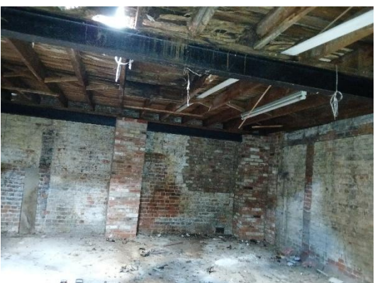
Plate 15. Internal view of Building 2.
