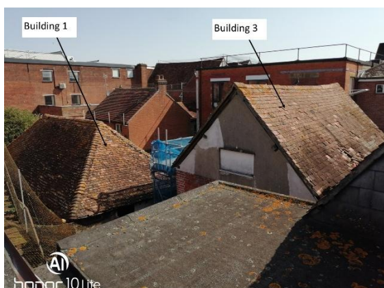
Plate 9. Southern and western elevations of Buildings 1 and 3.
