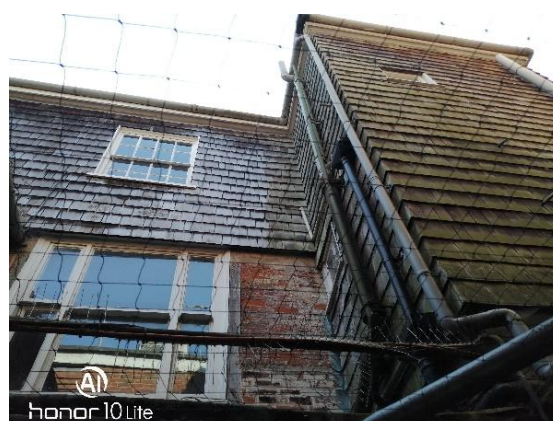
Plate 10. Western elevation of Building 5.
