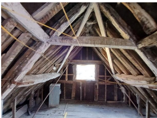
Plate 17. Internal view of Building 4.
