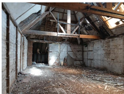
Plate 14. Internal view of Building 1.
