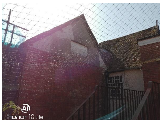
Plate 7. Western elevation of Building 3.
