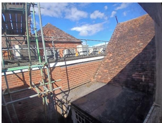
Plate 16. Western elevation of Building 1 and Building 3.
