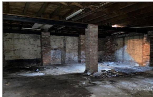
Figure 1 - Existing flat roof structure
