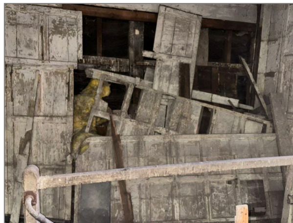
Figure 4 - Existing panelling to be repaired and reused
