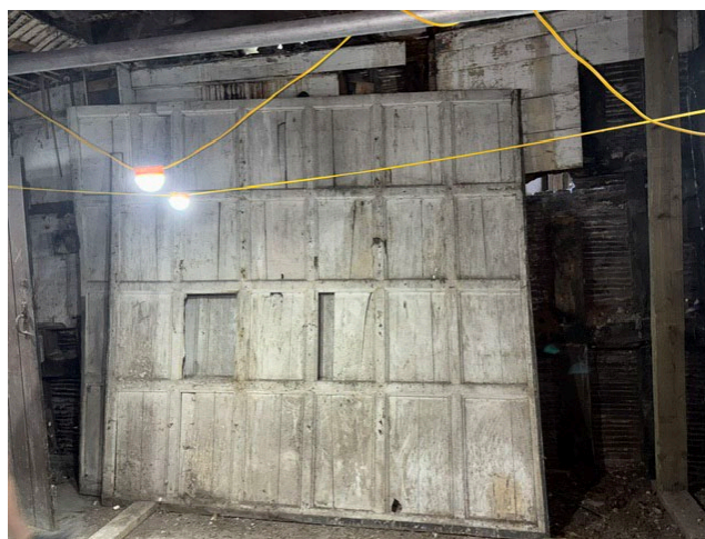
Figure 5 - Existing panelling to be repaired and reused
