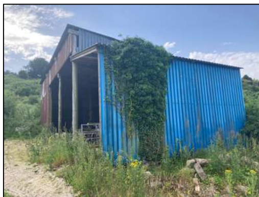
Figure 1 – northern corner of the barn with lean-to extension.
