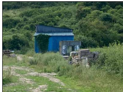
Figure 2 – north-western elevation of the barn in context of the surrounding habitat.
