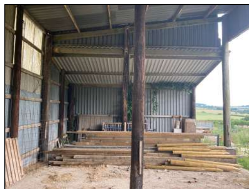
Figure 4 – interior of the barn looking northwest.
