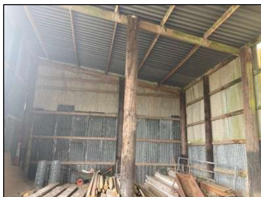
Figure 3 – interior of the barn looking southeast.
